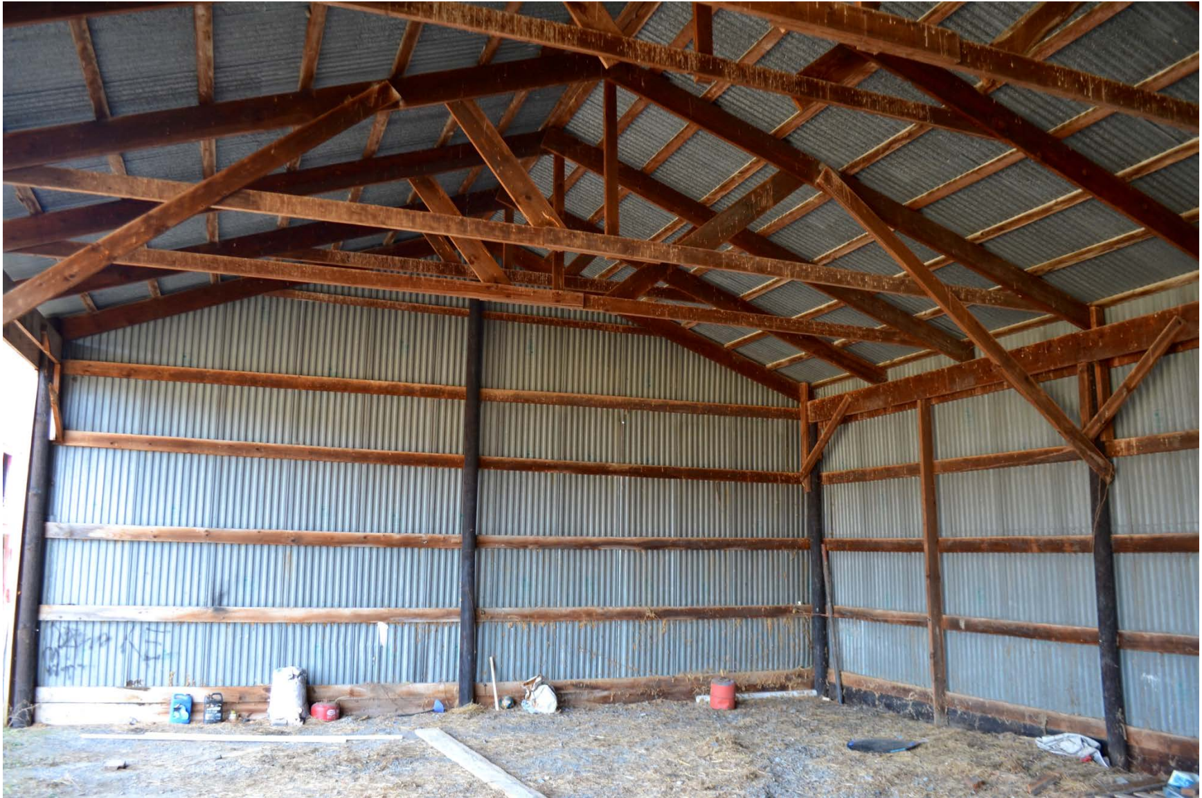
Photo 37. Facing south Interior of northernmost outbuilding on farm complex.
