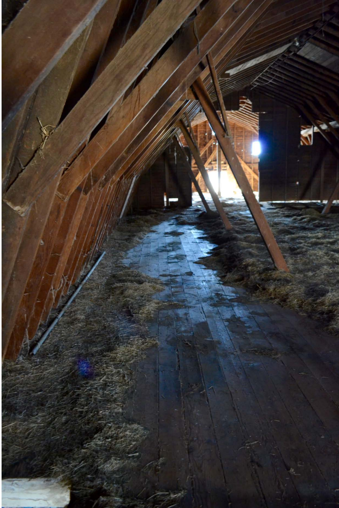
Photo 25. Interior of main barn. South side of interior facing west. Showing construction of the roof support and the wooden floor.
