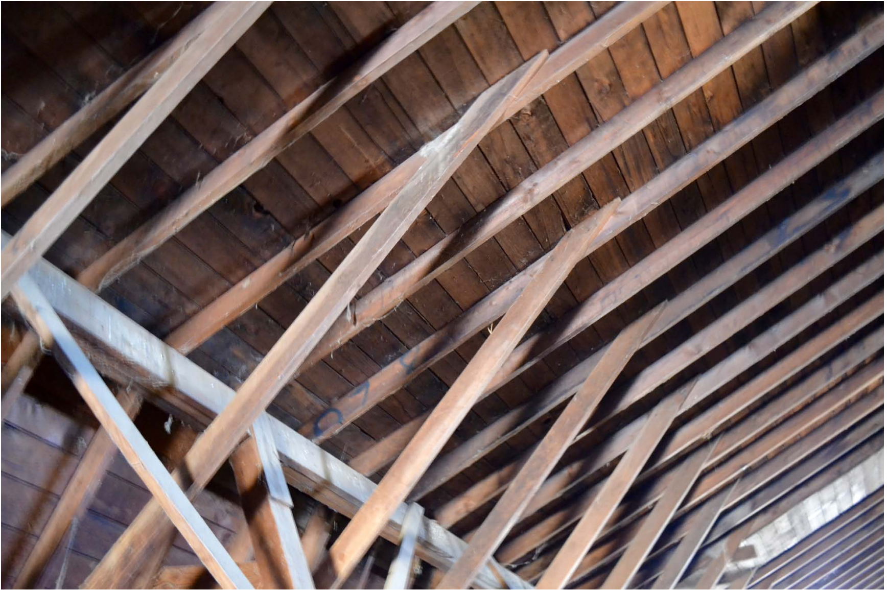
Photo 26. Interior photo of gambrel roof construction of main barn. View from second floor.
