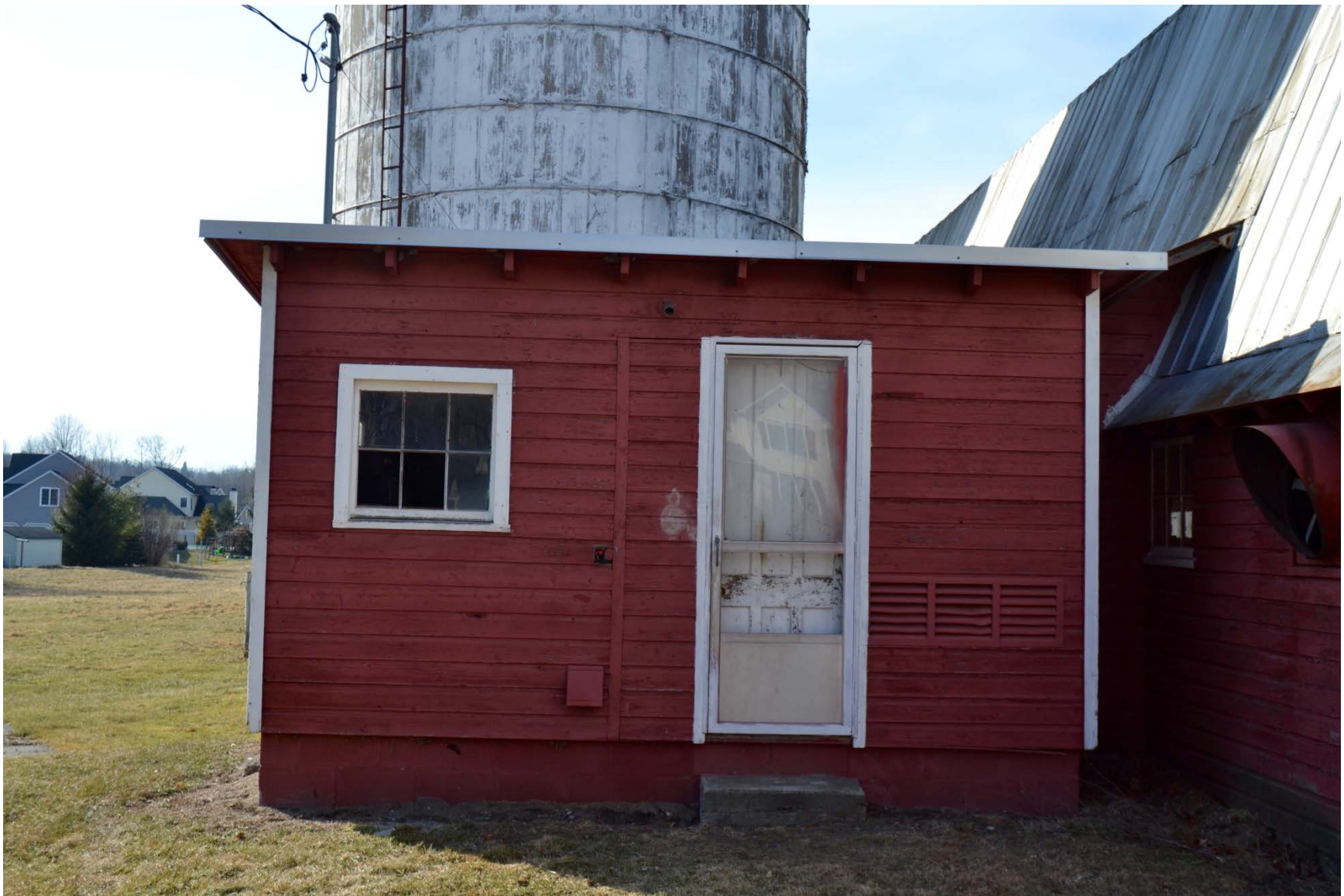
Photo 7. Facing west. Front facade of milk house.
