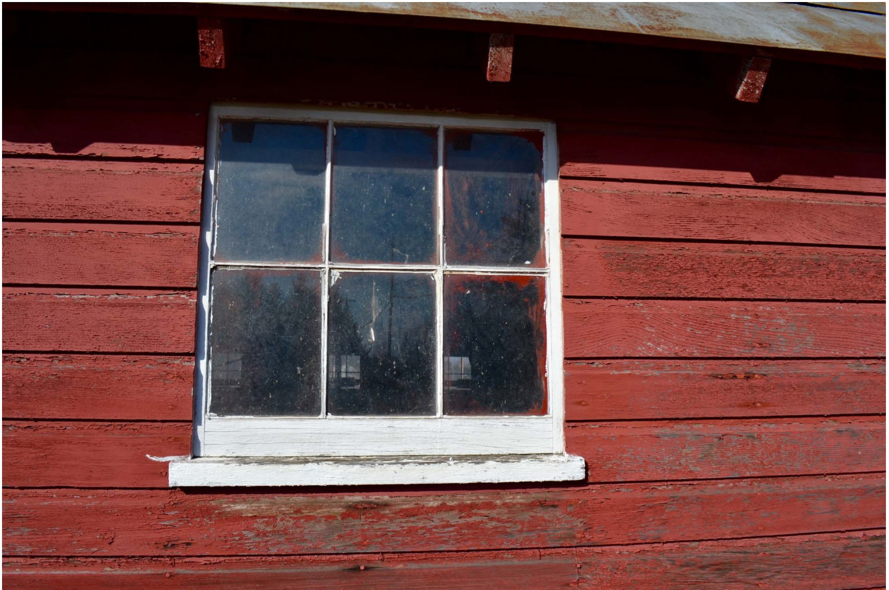
Photo 13. Six light wooden sash casement window. Typical of the fenestration of the main barn.
