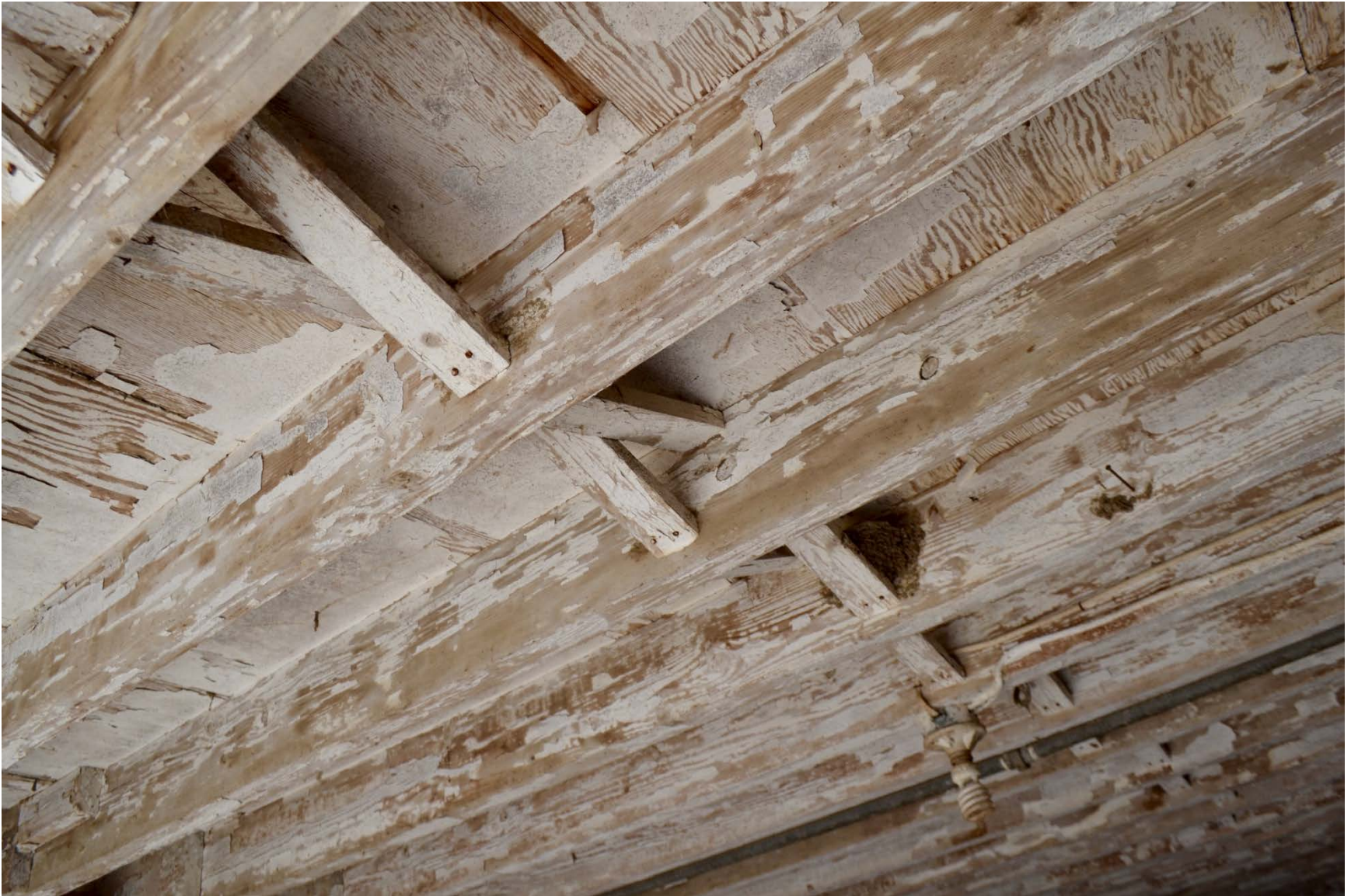
Photo 22. First floor ceiling joists and stabilizers.
