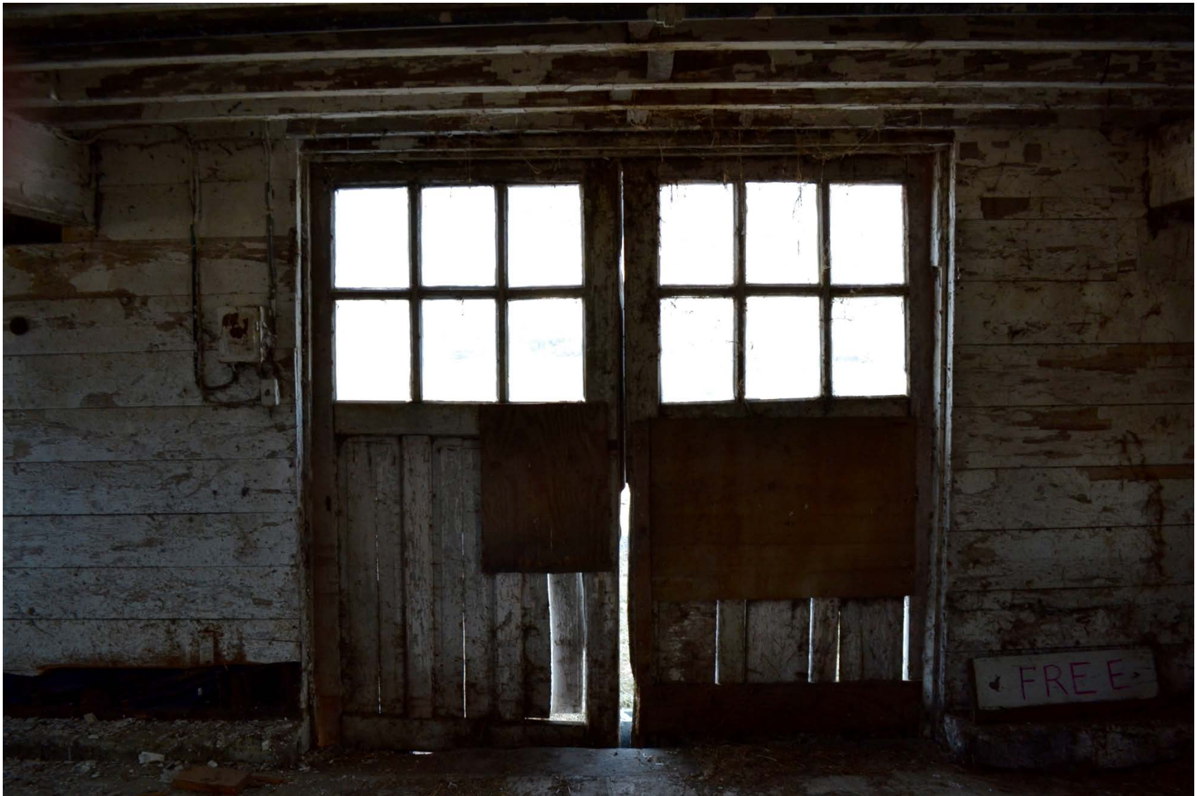
Photo 19. Interior of front sliding doors of main barn on first floor.
