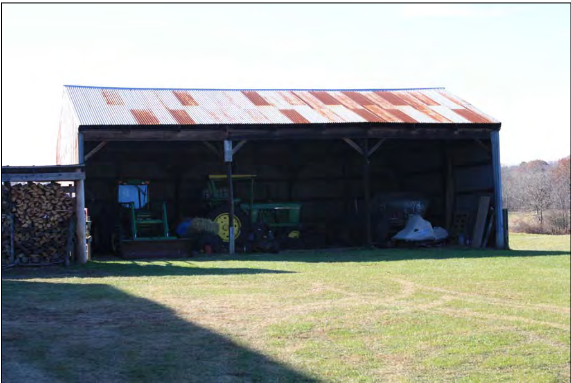
View West of Metal Equipment Shed "D" (IMG 4890)
