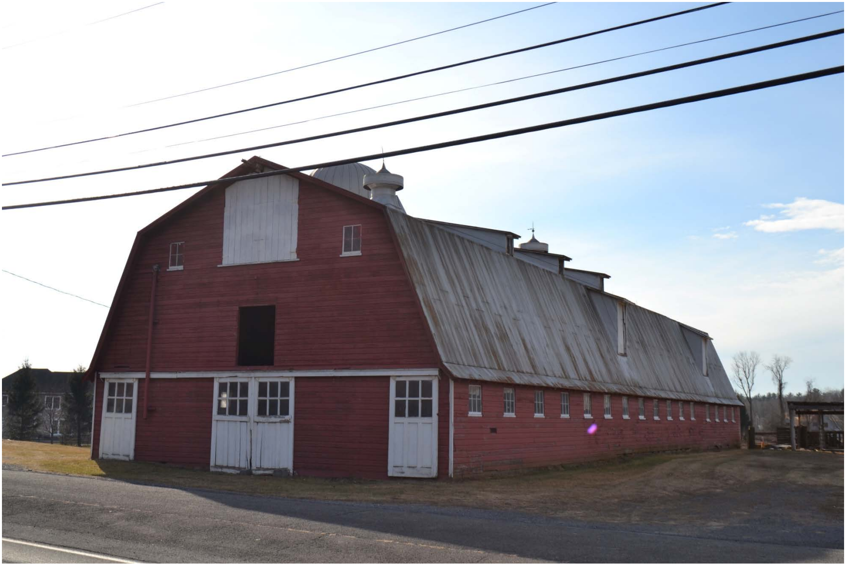
Photo 16. Facing southwest. Exterior of main barn.
