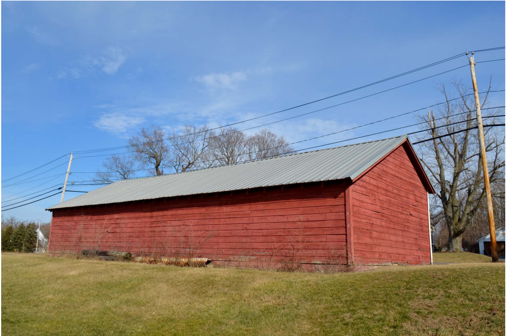
Photo 3. Facing northeast. Rear of southernmost outbuilding on farm complex.
