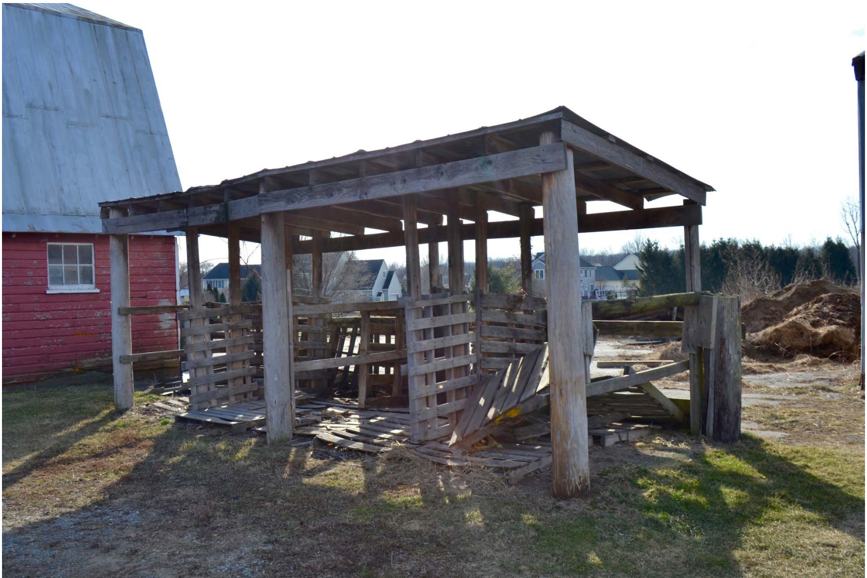
Photo 38. Facing southwest. Horse stanchions.
