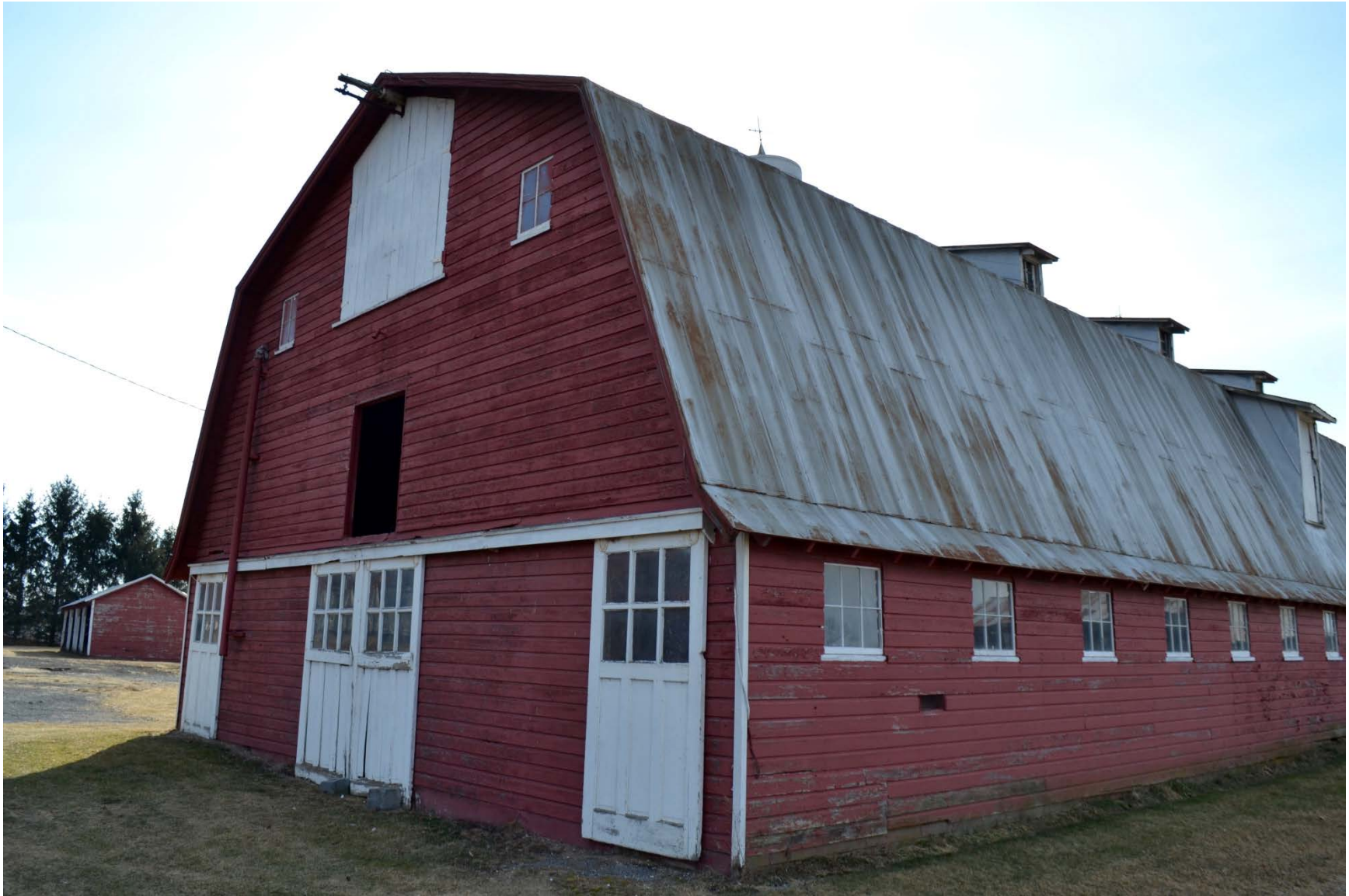
Photo 17. Facing southwest. Exterior of main barn. Showing front facade, gambrel roof, fenestration layout, and positioning of roof dormers.
