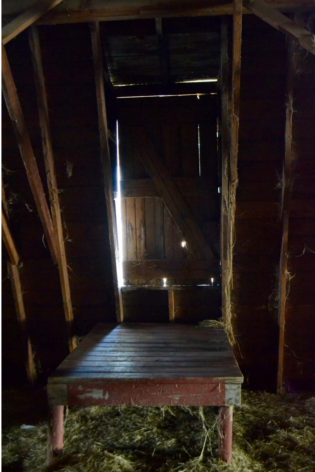
Photo 27. Interior photo of exterior door in main barn on the second floor.
