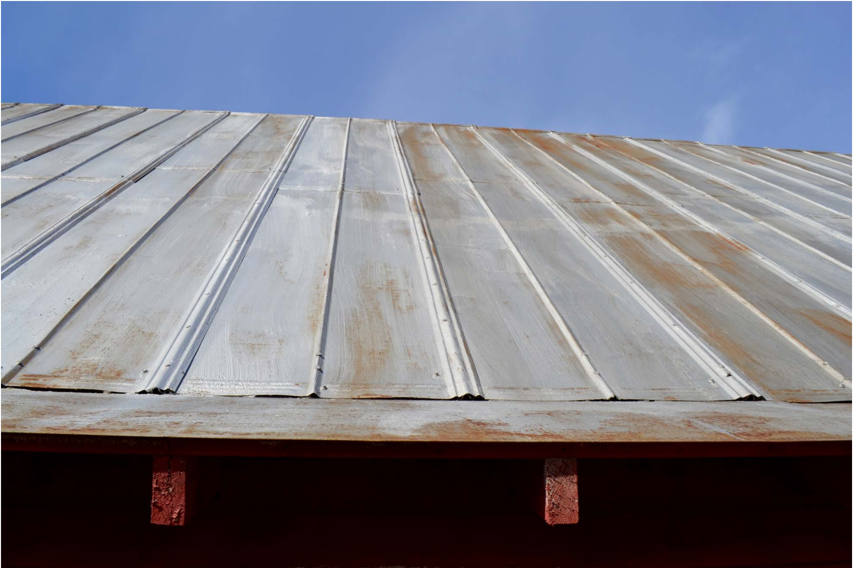
Photo 14. Metal roof detail of the main barn.
