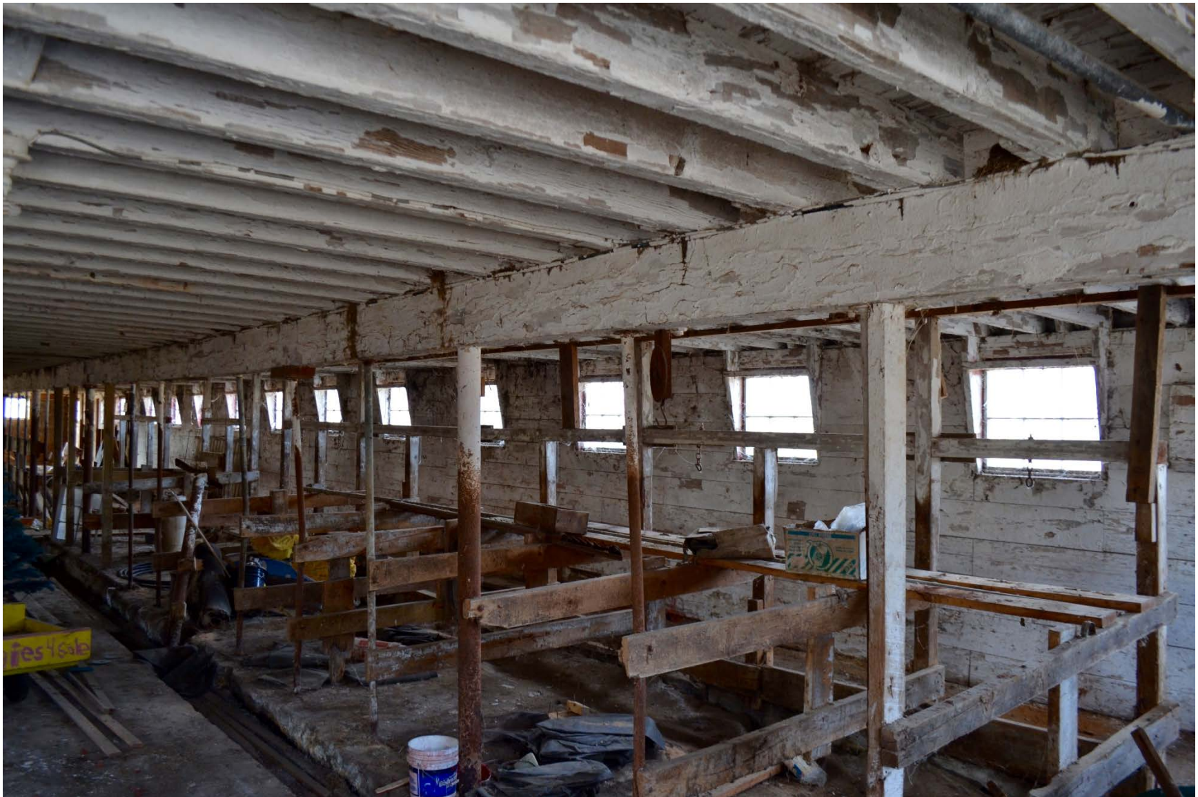
Photo 20. Interior of main barn, first floor showing layout of stanchions made of steel pipe and wood.
