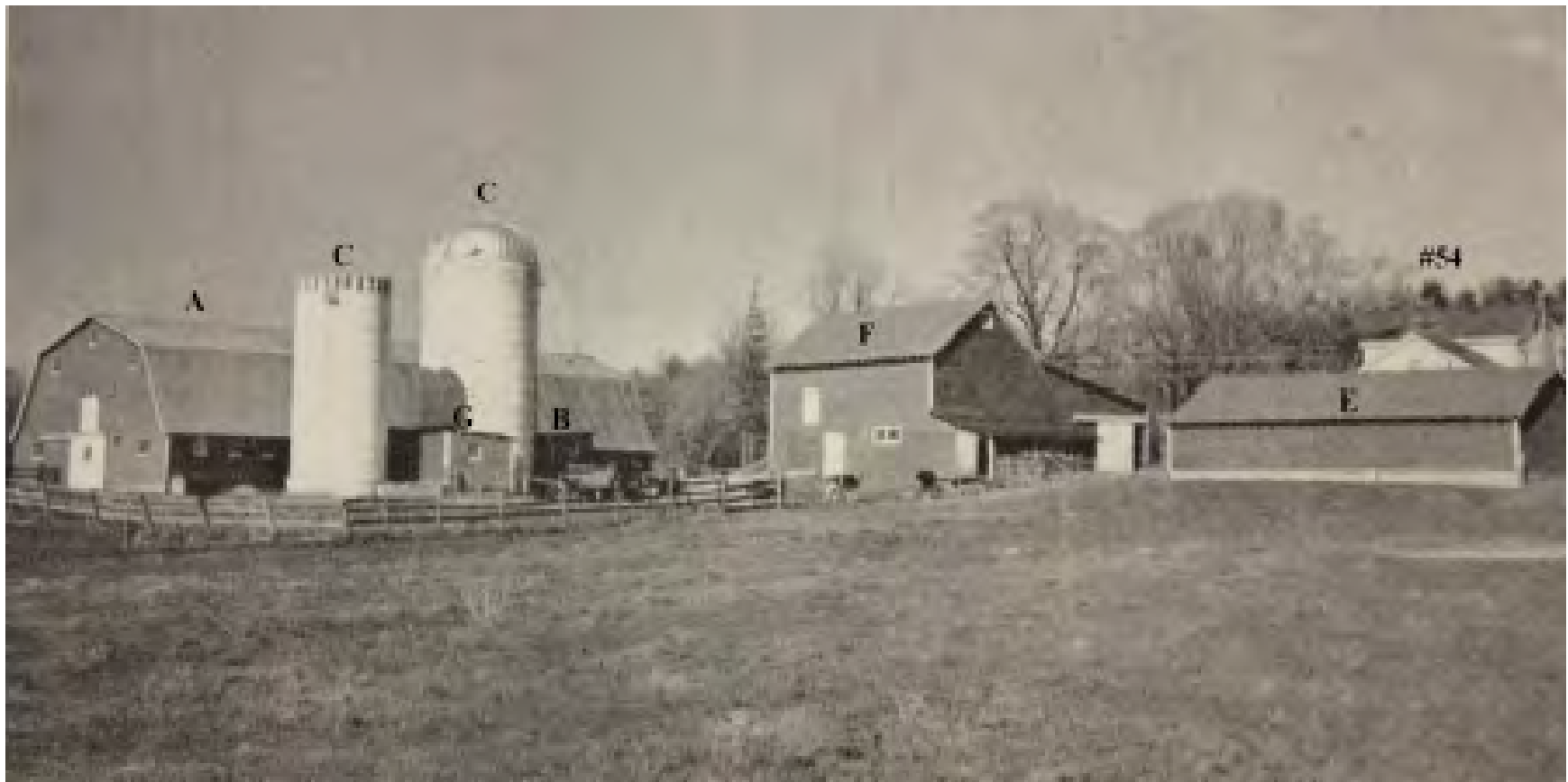
Figure 4. Historic photograph circa 1960 showing the view of the Sandy Creek Farm-Newell Dairy Infrastructure from the north.
