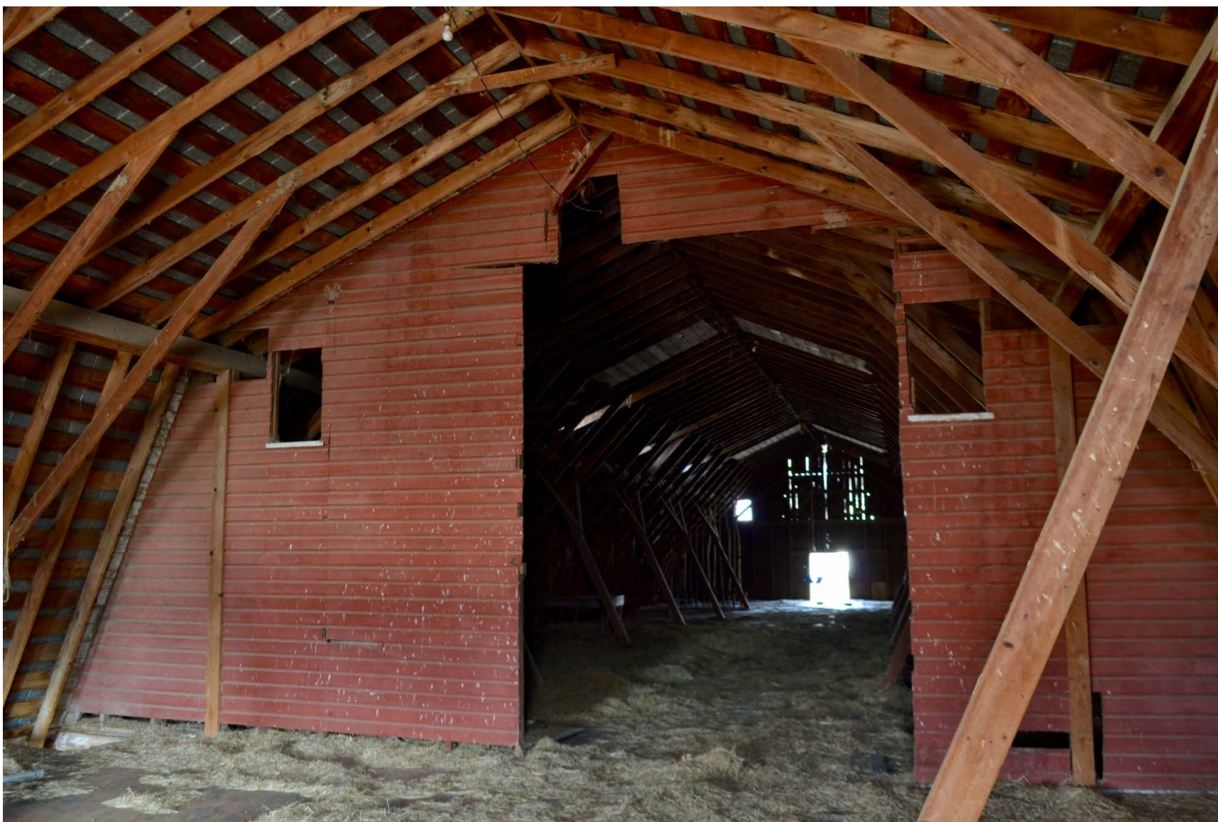
Photo 29. Facing east. Interior of main barn, second story. Showing an addition on the western end of the main barn.
