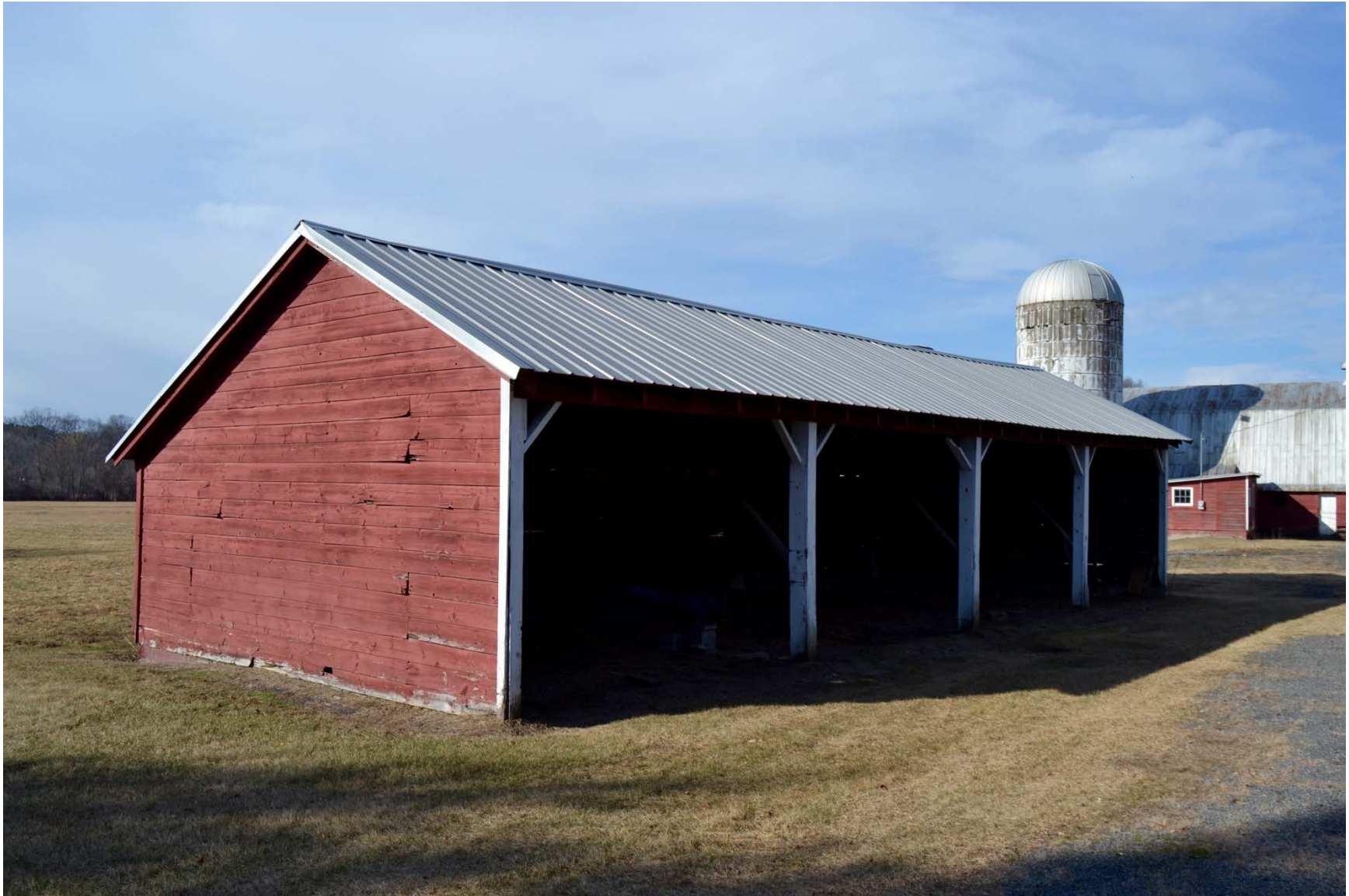
Photo 1. Facing northwest. Front of southernmost outbuilding on farm complex.
