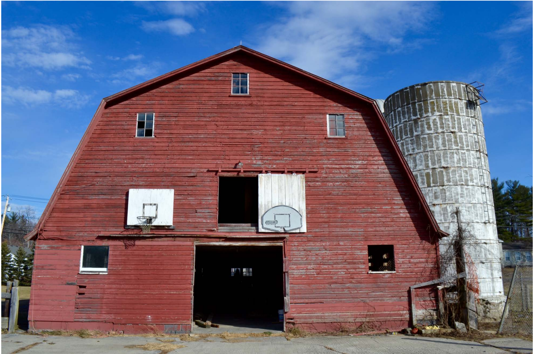
Photo 33. Facing north. Rear facade of main barn.
