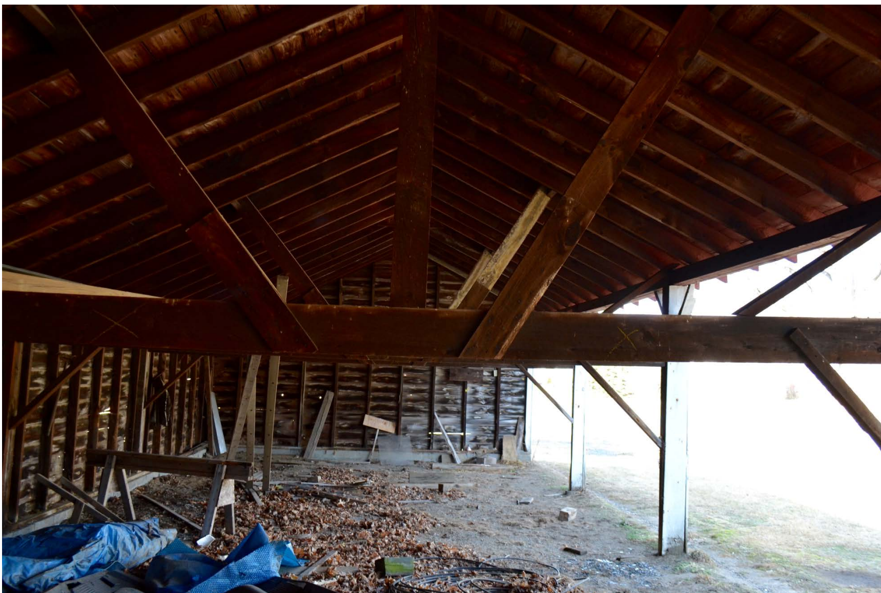
Photo 2. Facing north. Interior of southernmost outbuilding on farm complex.
