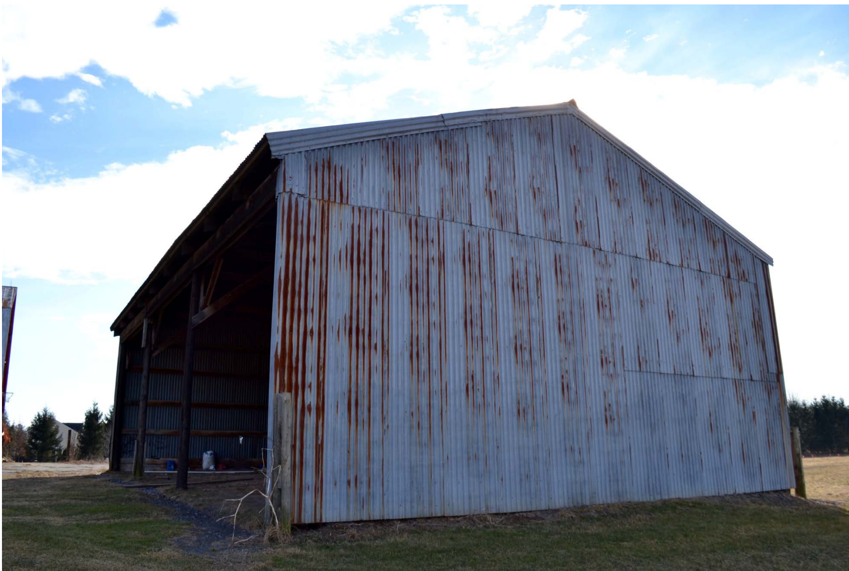
Photo 36. Facing south. Northernmost outbuilding on farm complex.
