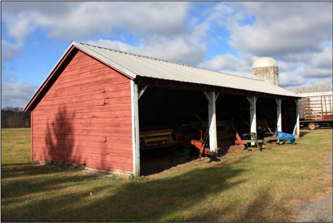
View northwest of Frame Equipment Shed "E." (IMG 4993)
