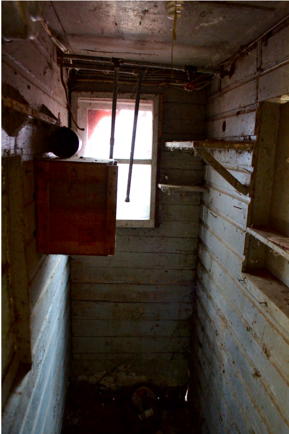
Photo 11. Interior hallway between milk house and main barn.
