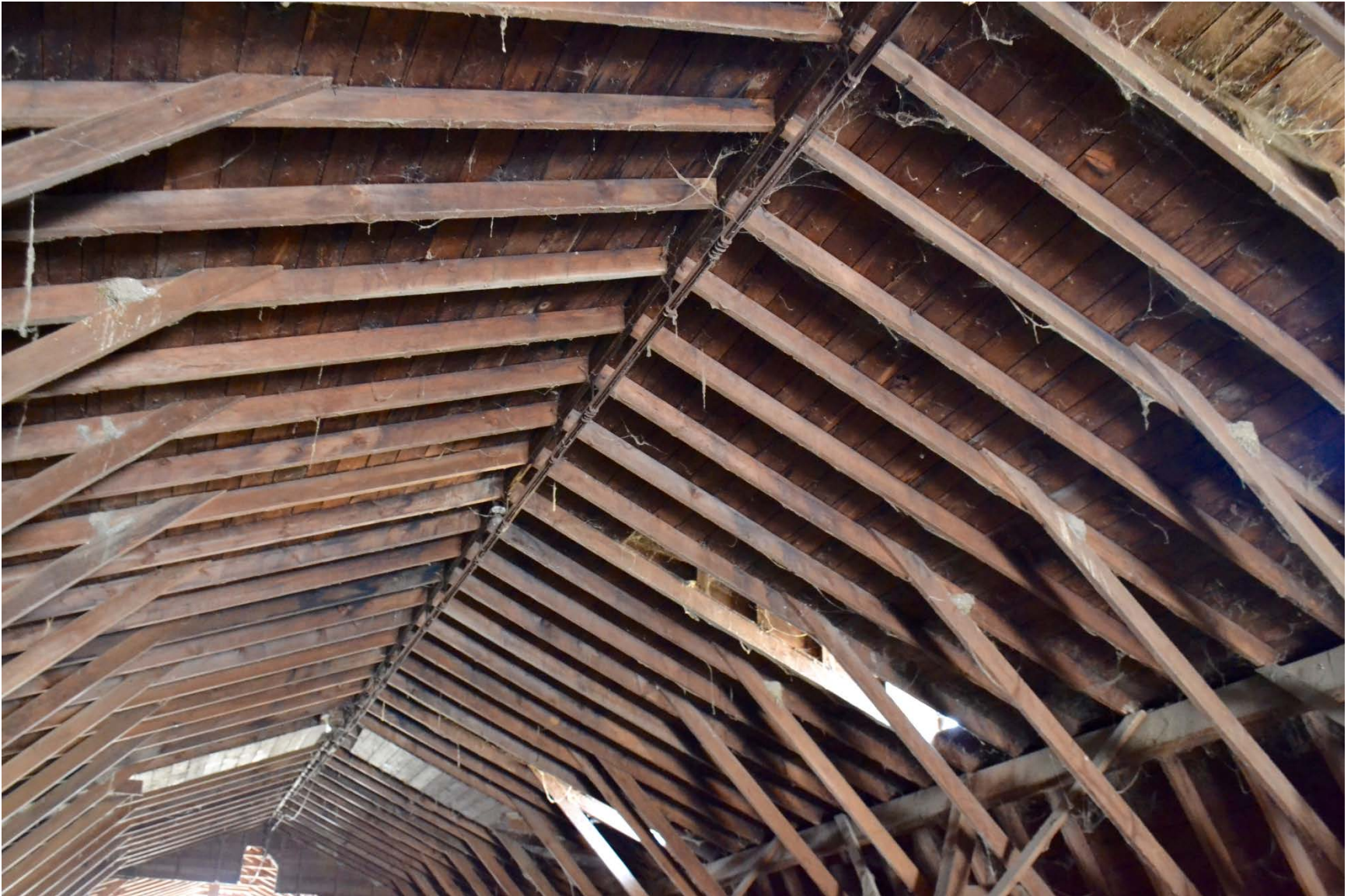
Photo 23. Gambrel roof construction of main barn. View from second floor.
