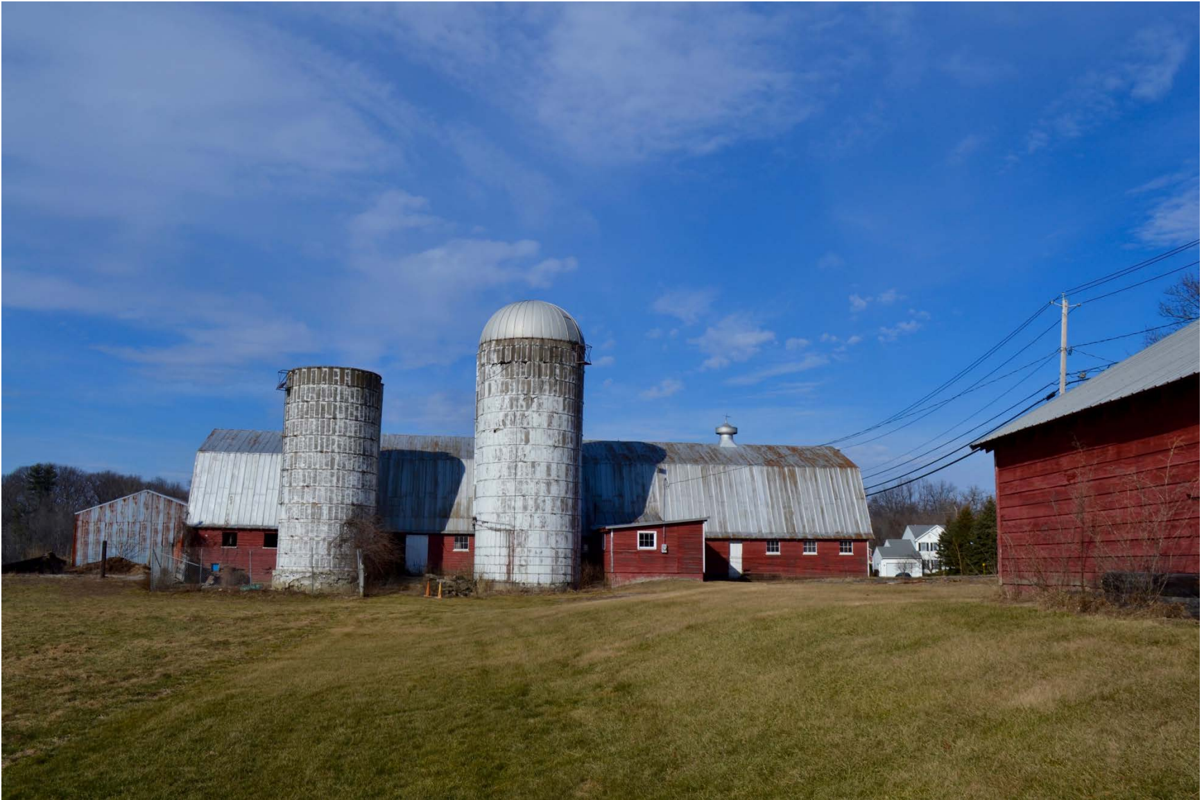
Photo 4. Facing north. Exterior of main barn on complex.
