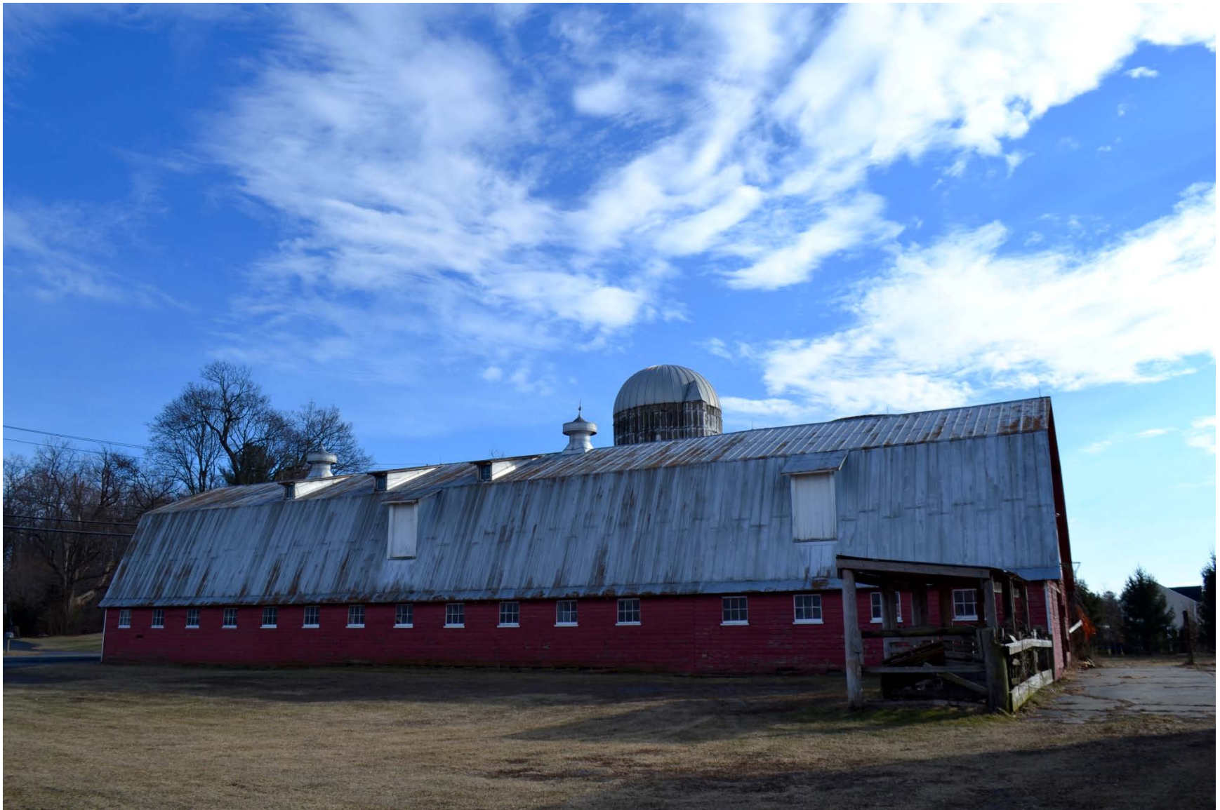
Photo 34. Facing south. Showing main barn and horse stanchions in the foreground.
