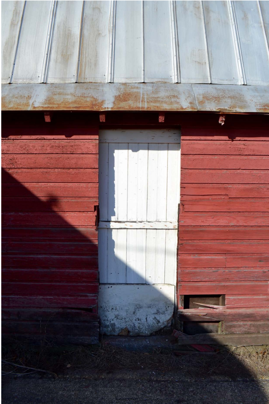
Photo 12. Facing north. Exterior wooden door of main barn. Also clearly showing the clapboard siding and the metal roof material.
