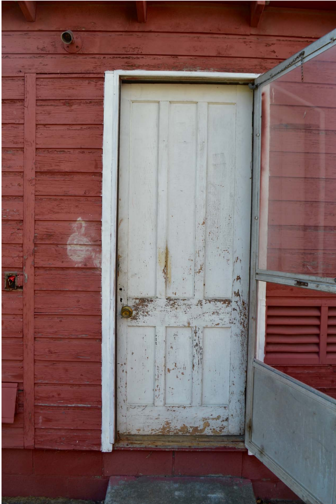
Photo 8. Six paneled front door and clapboard siding on milk house with aluminum storm door open.
