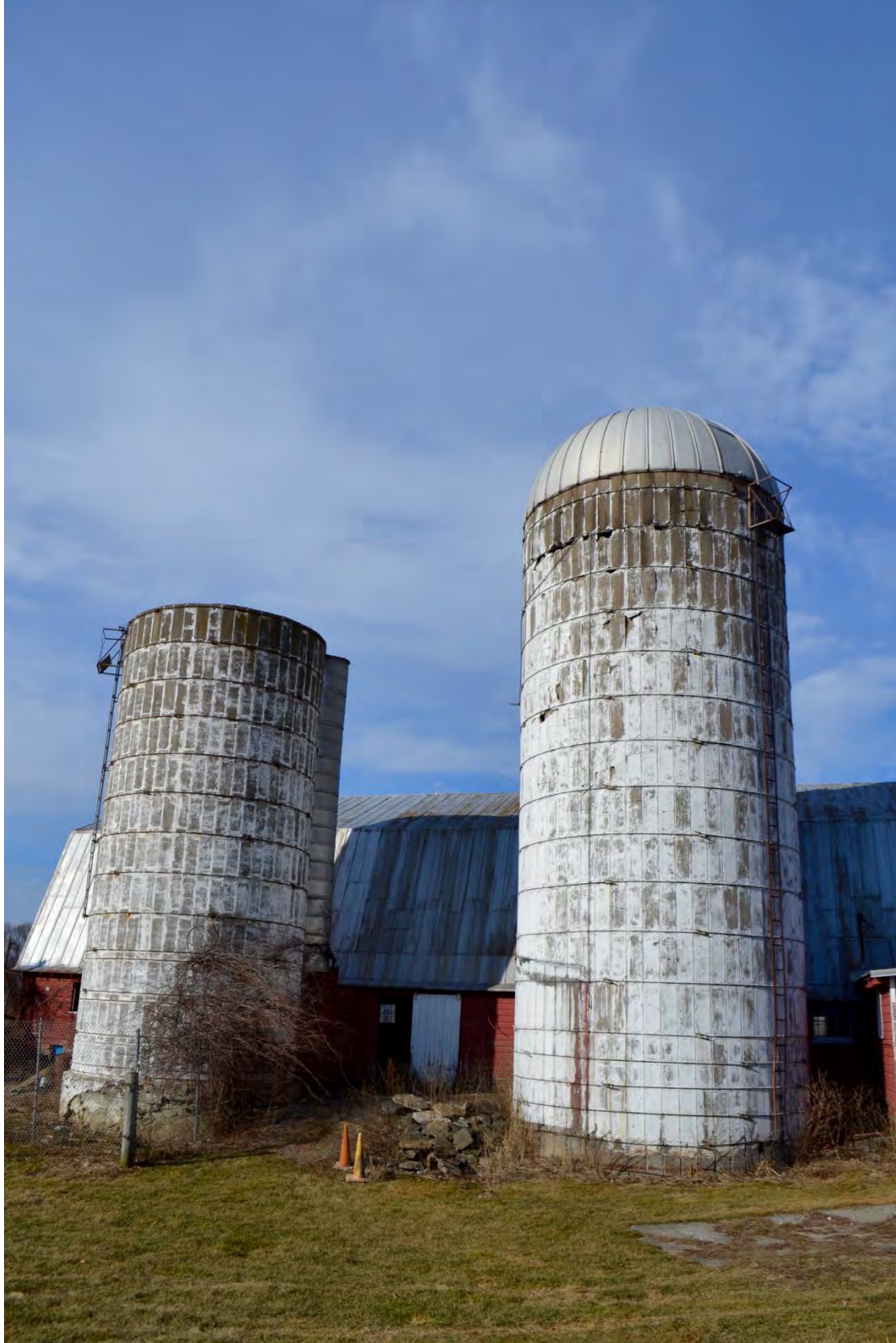
Photo 5. Facing north. Grouping of two silos adjacent to main barn.
