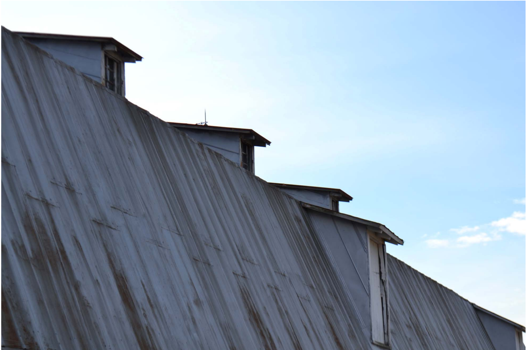
Photo 18. Detail of roof dormers on main barn.
