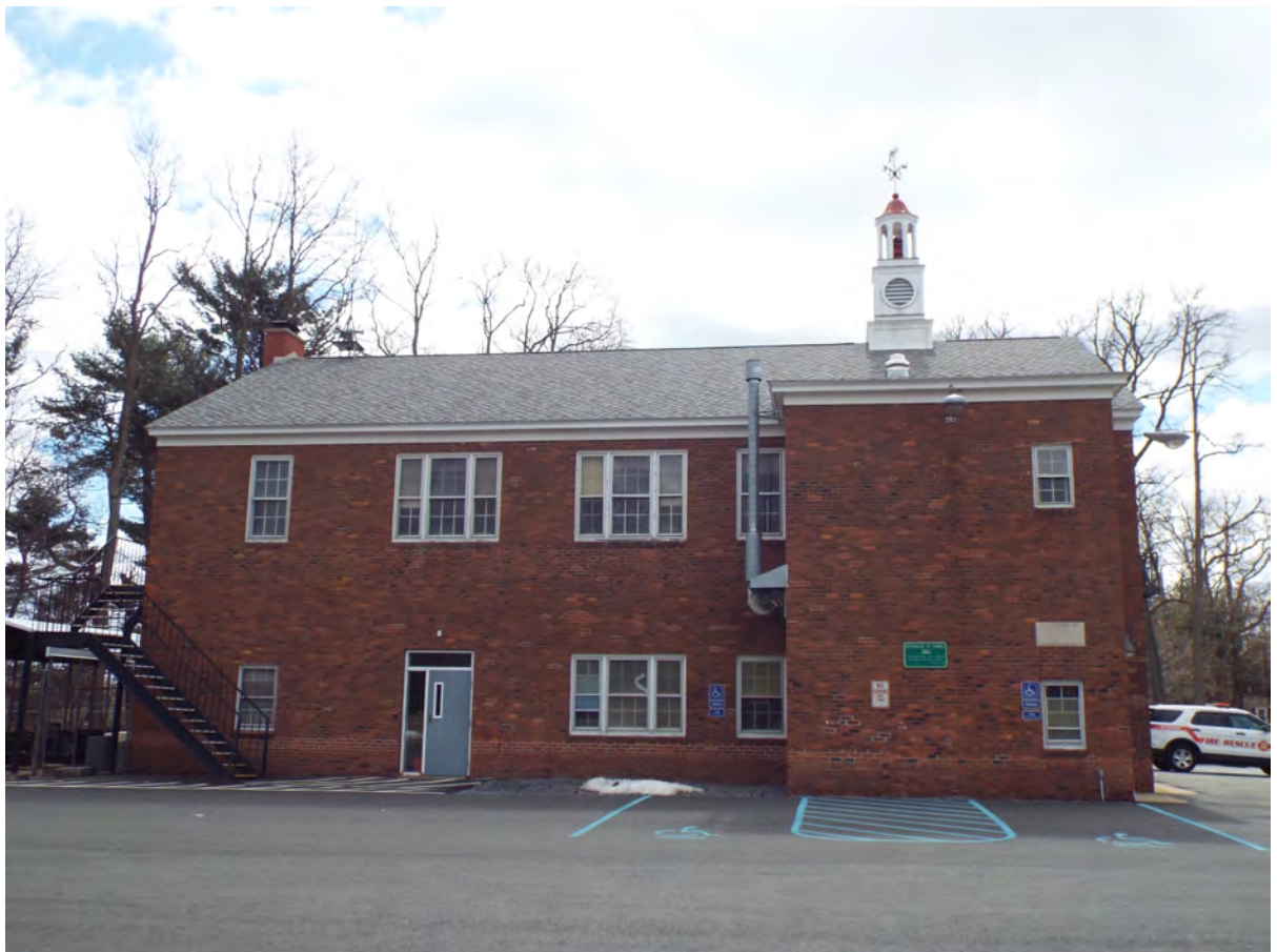
Photo 2. Rotterdam Fire District #7, facing south.
