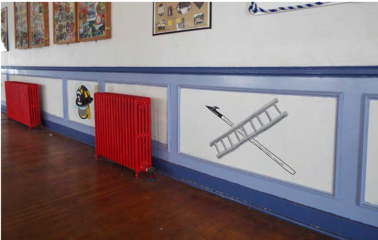
Photo 14. Rotterdam Fire District #7, view of paneled wainscoting which surrounds entire auditorium on second floor.
