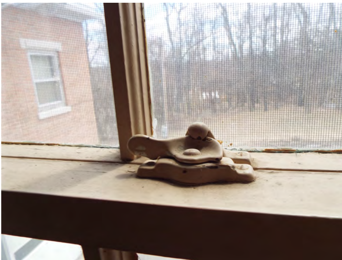
Photo 16. Rotterdam Fire District #7, view of top rail of interior of window in upstairs. Shows original hardware and the quality of sashes still in place.
