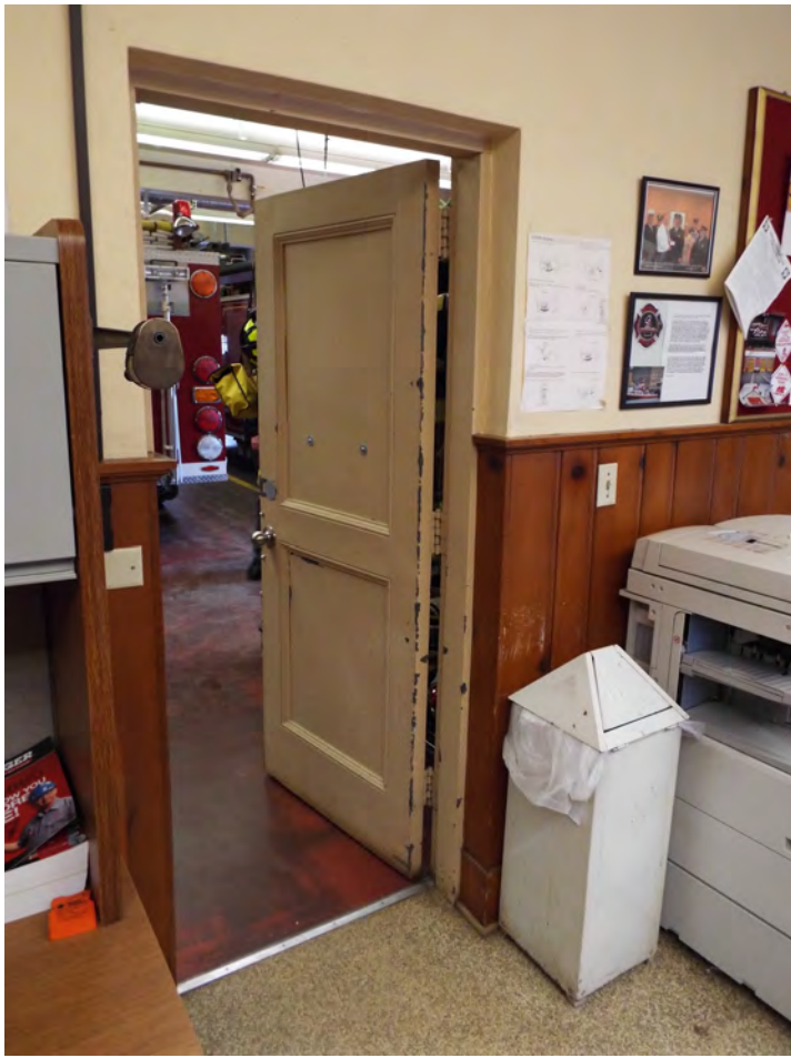
Photo 9. Rotterdam Fire District #7, view of first floor interior, two paneled door with associated trim. Between main garage space and break room.
