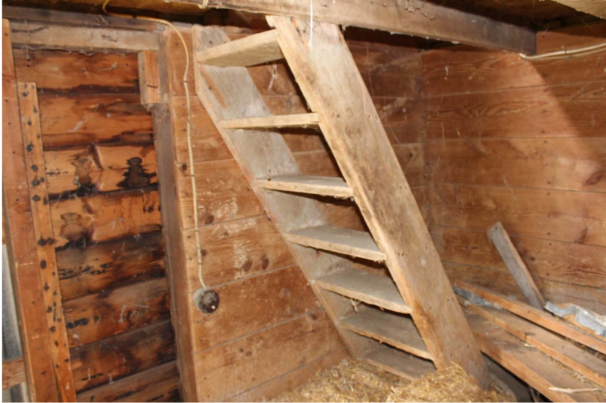
Photo 29. View of stair leading to the upper level of the poultry house.
