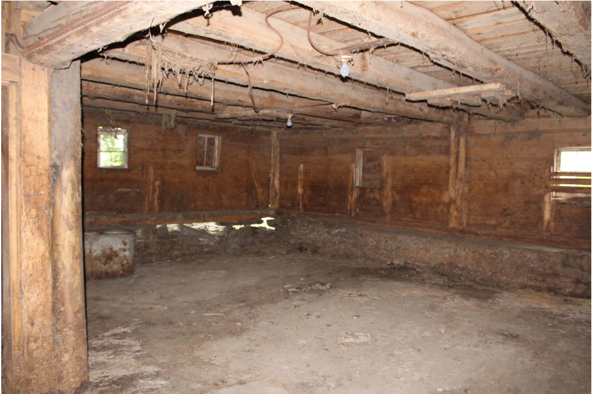
Photo 22. View of the first floor of the horse barn showing the stone foundation.
