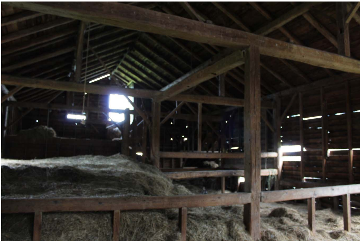
Photo 6. Interior of the main barn showing the truss system and divided hay mows.
