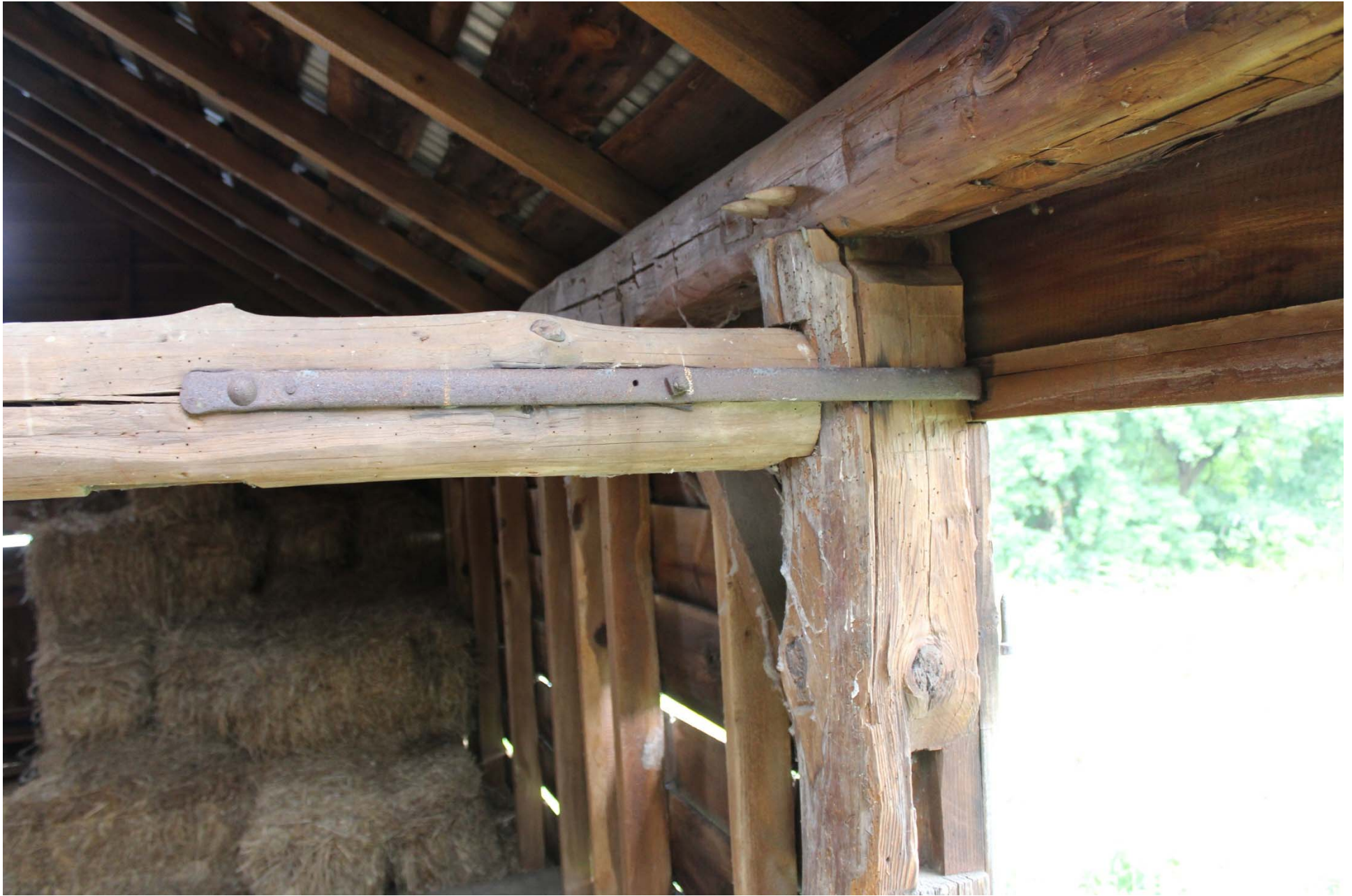
Photo 15. View of wrought iron strap used to connect the purlins to the wall post.
