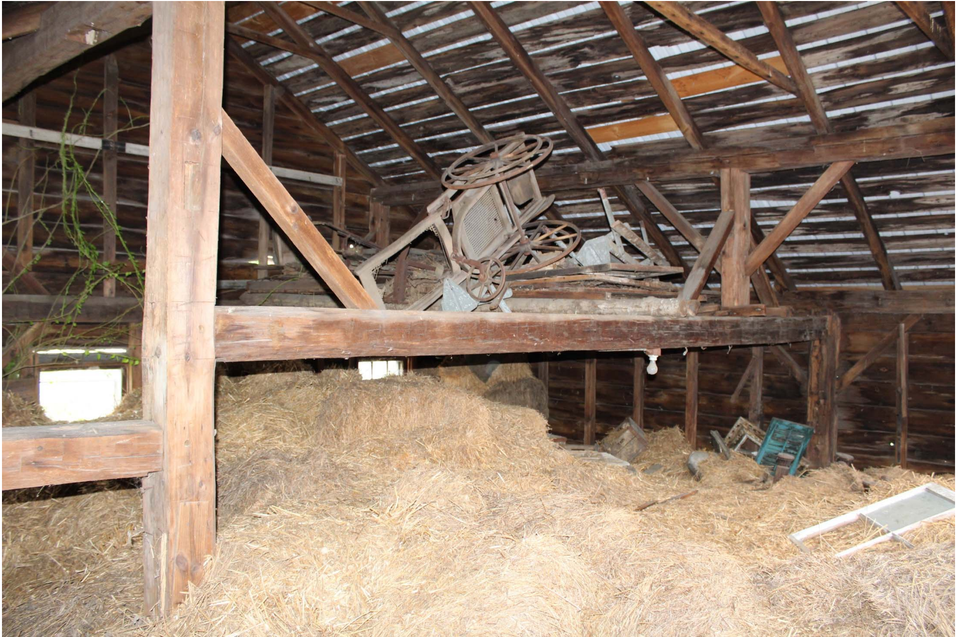
Photo 21. View of framing in the upper story of the horse barn. Note asymmetrical framing and partial H bent at left.
