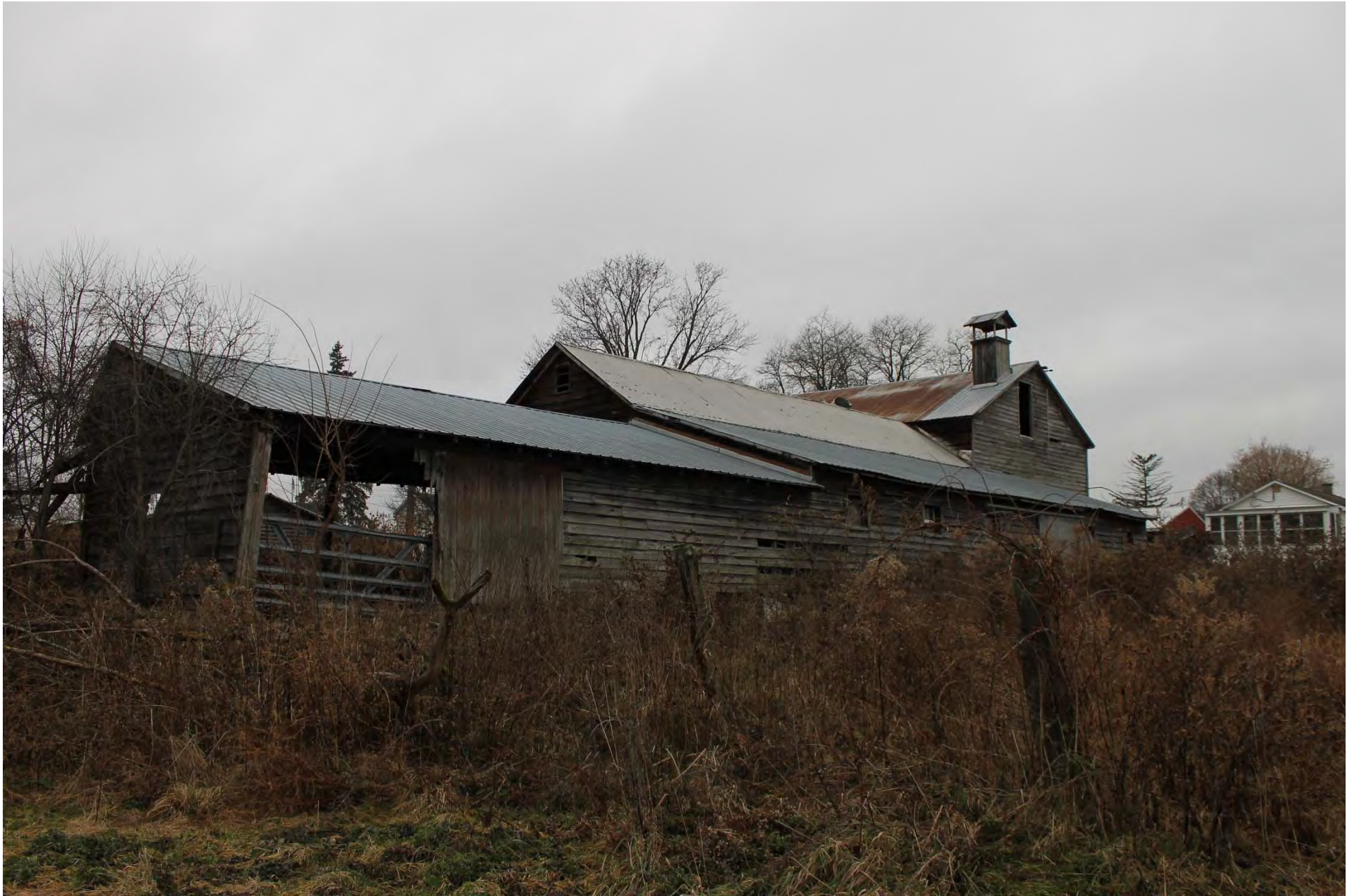
Photo 4. View of 20th century shed addition at the southeast corner of the main dairy barn complex.
