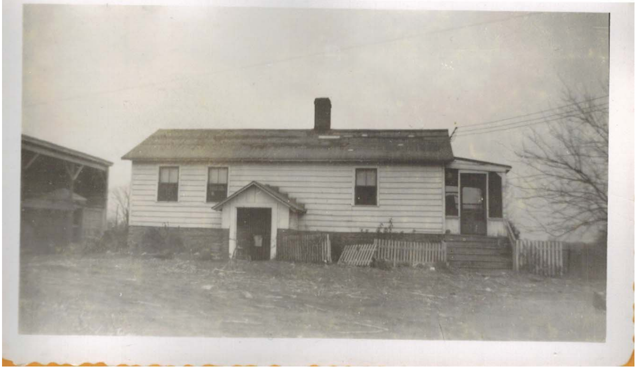
Photo 41. Historic photograph of the mid- 20 th century house built upon an 18 th century brick foundation. Photo courtesy Bethlehem Town Historian.
