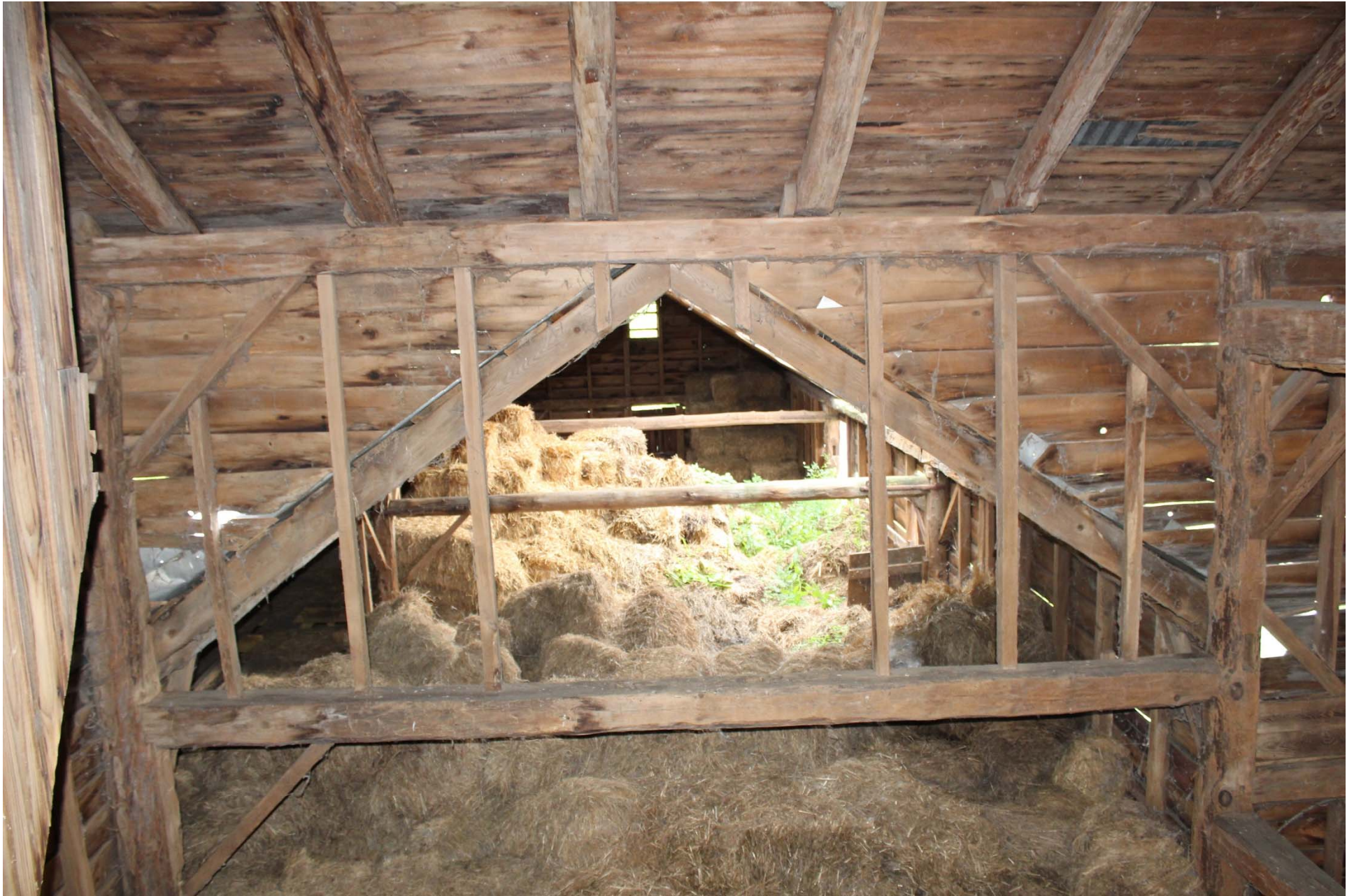
Photo 16. View of the 19th century addition from the main dairy barn. Note how the vertical framing of the original barn was cut to allow entry into the new addition.
