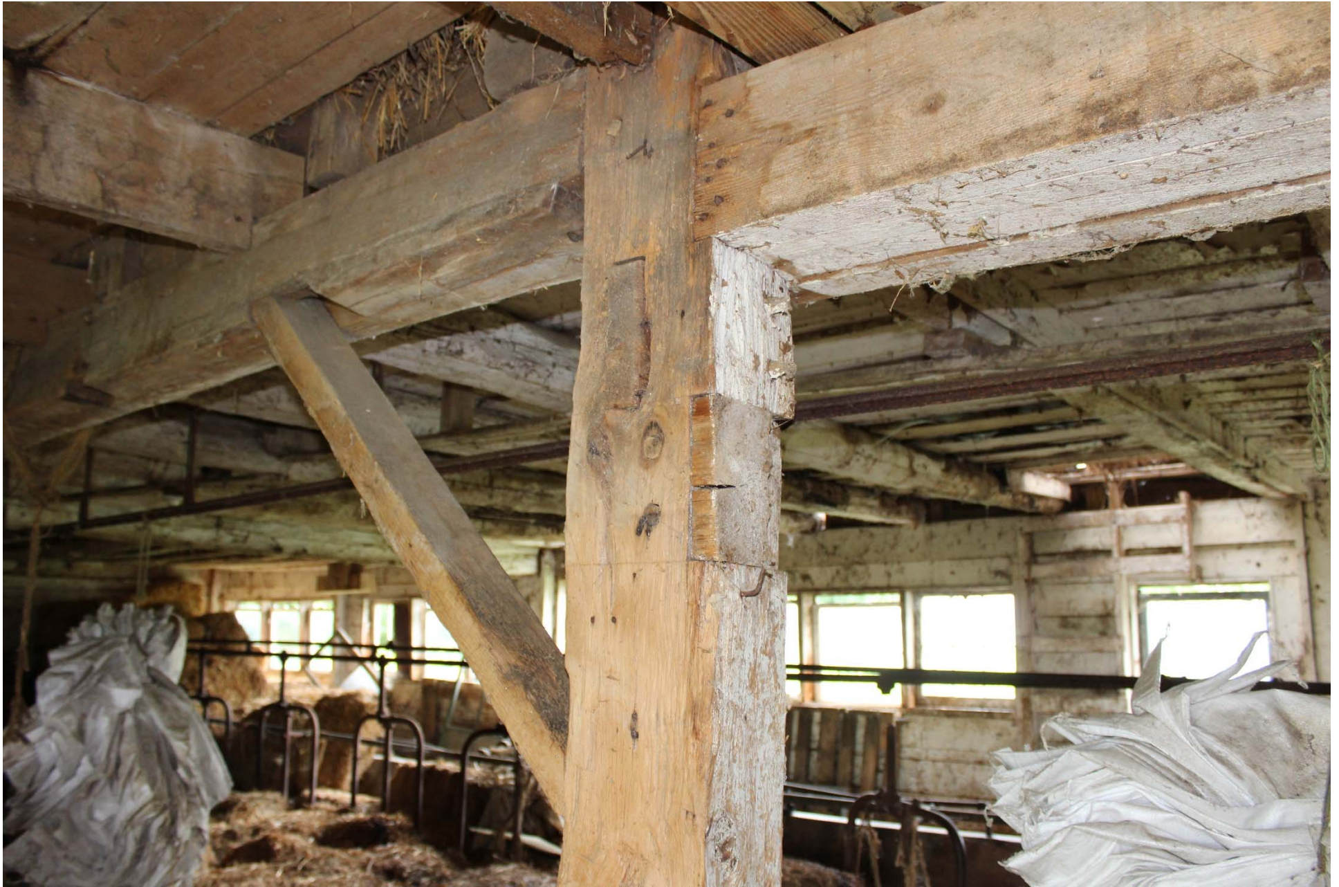
Photo 19. View of timber framed joint with brace in the first floor of the main dairy barn.
