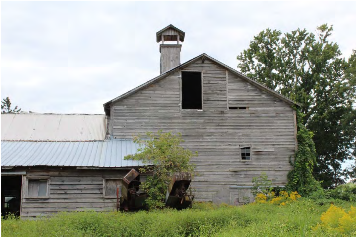
Photo 5. Northern façade of the main dairy barn showing its distinctive wooden vent and a 20 th century shed addition to the left.
