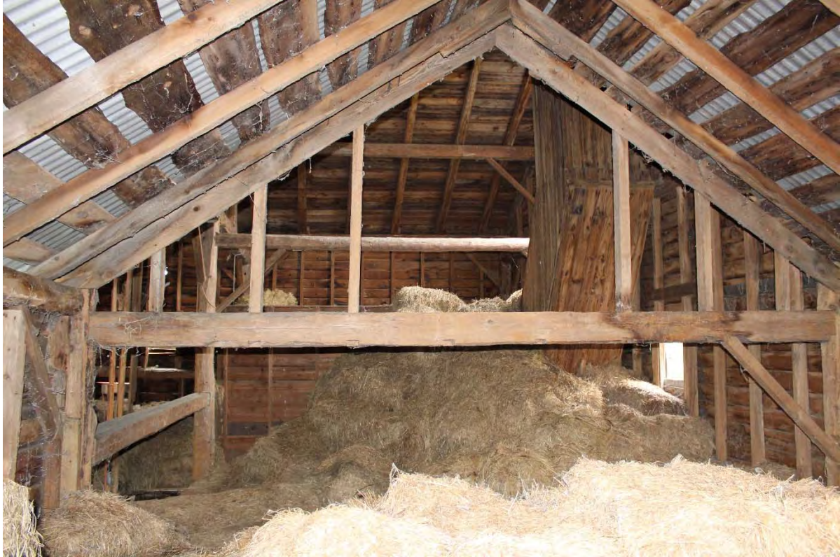
Photo 11. View from the 19 th century addition looking toward the original barn building showing framing, Note wooden vent on the right side of the photograph.
