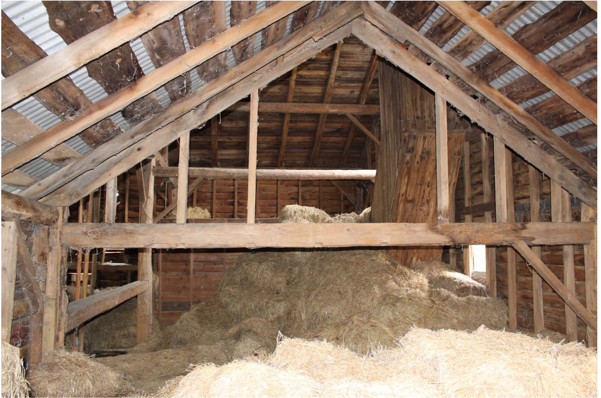
Photo 13. View from the 19th century addition looking toward the original barn building showing framing, Note wooden vent on the right side of the photograph.
