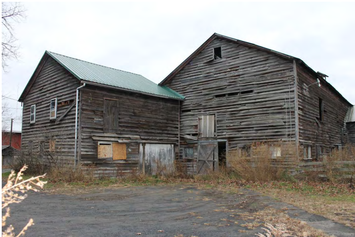
Photo 19. View of horse barn on the left and the original main barn on the right.
