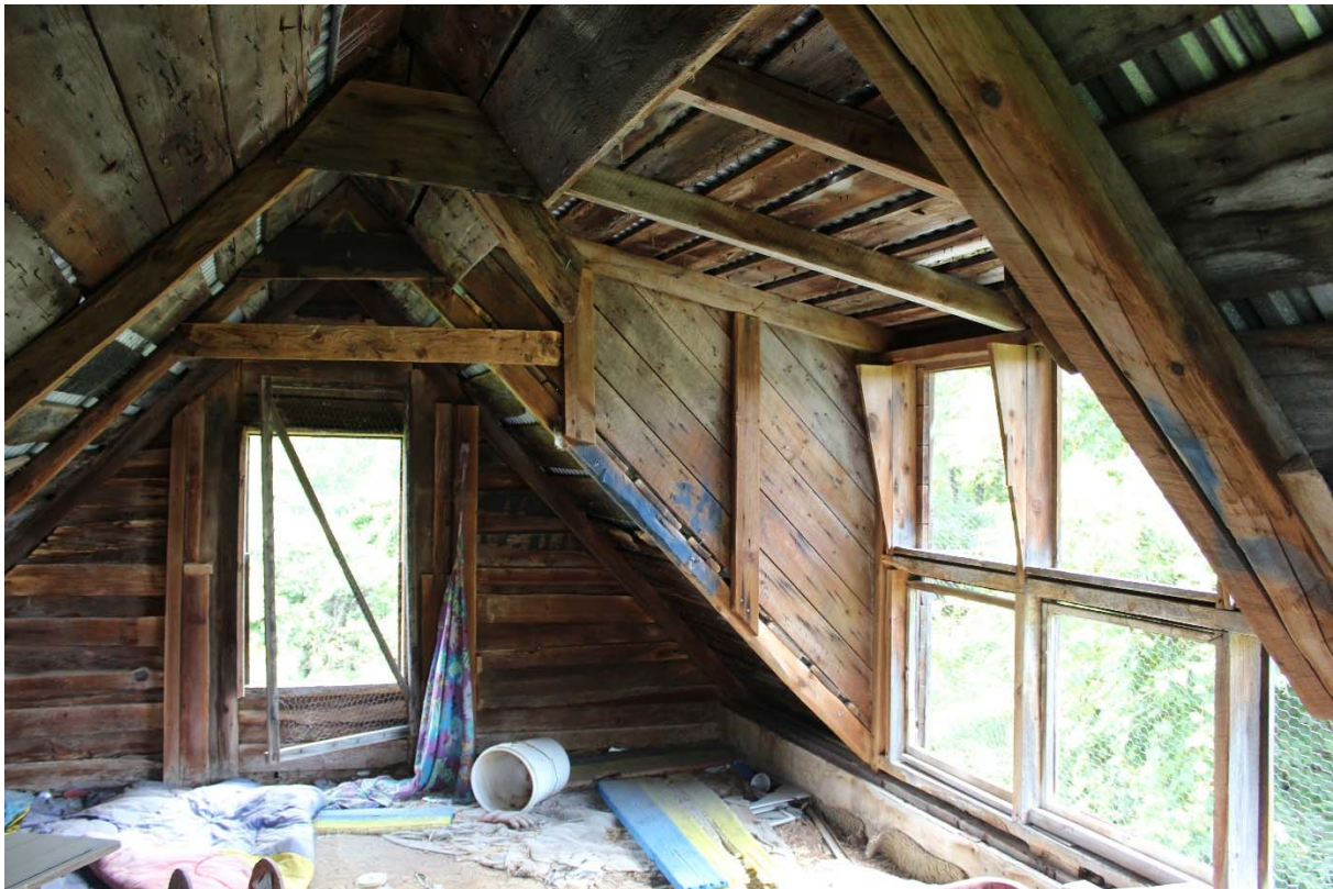
Photo 30. View of the interior of the upper story of the poultry house.
