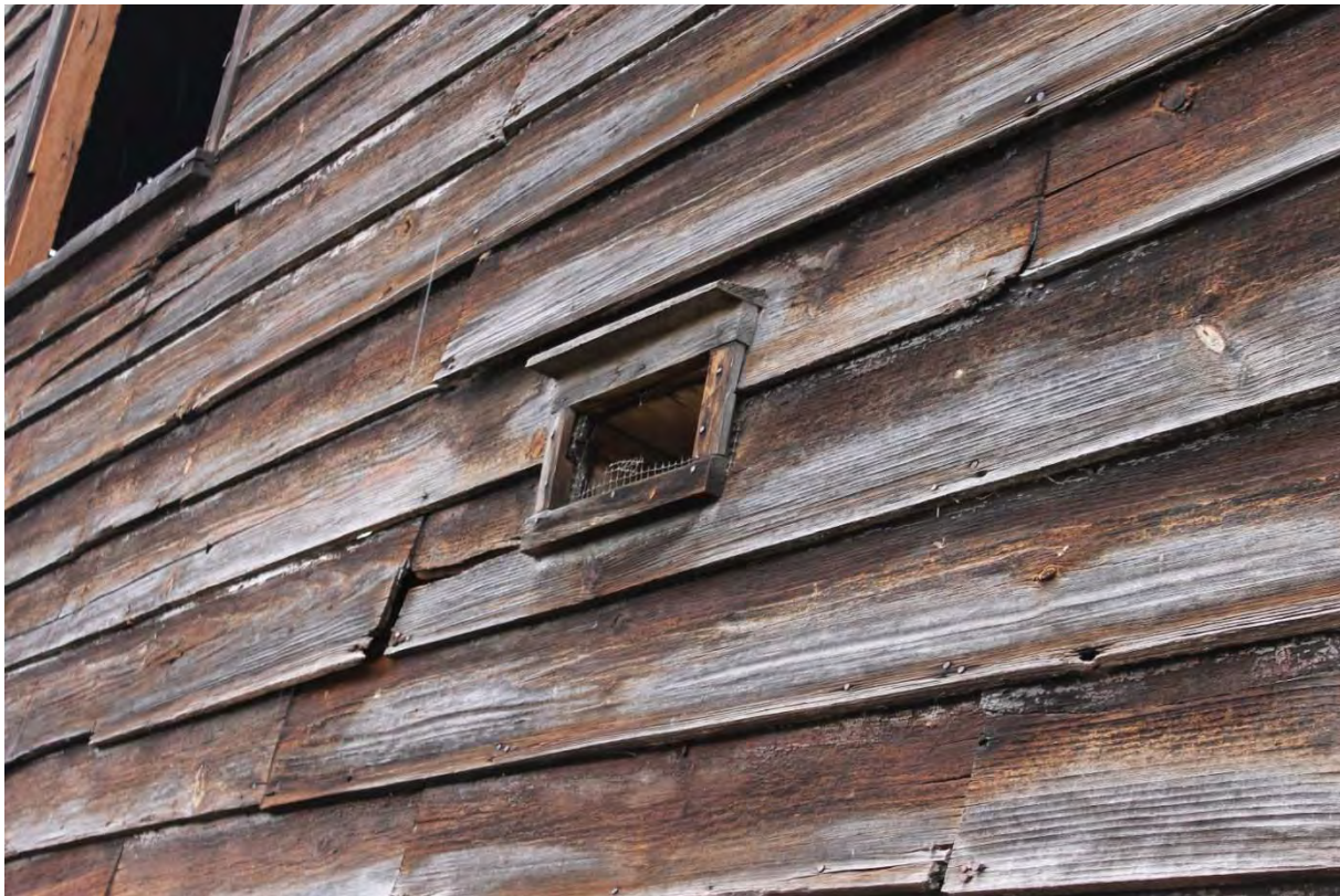
Photo 9. Vent on the exterior of the main dairy barn.
