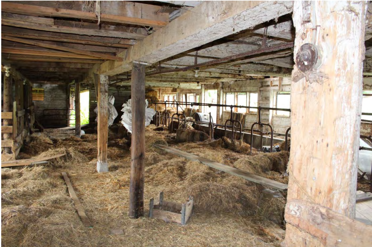
Photo 15. View of dairy stanchions on the first floor of the 19 th century addition.
