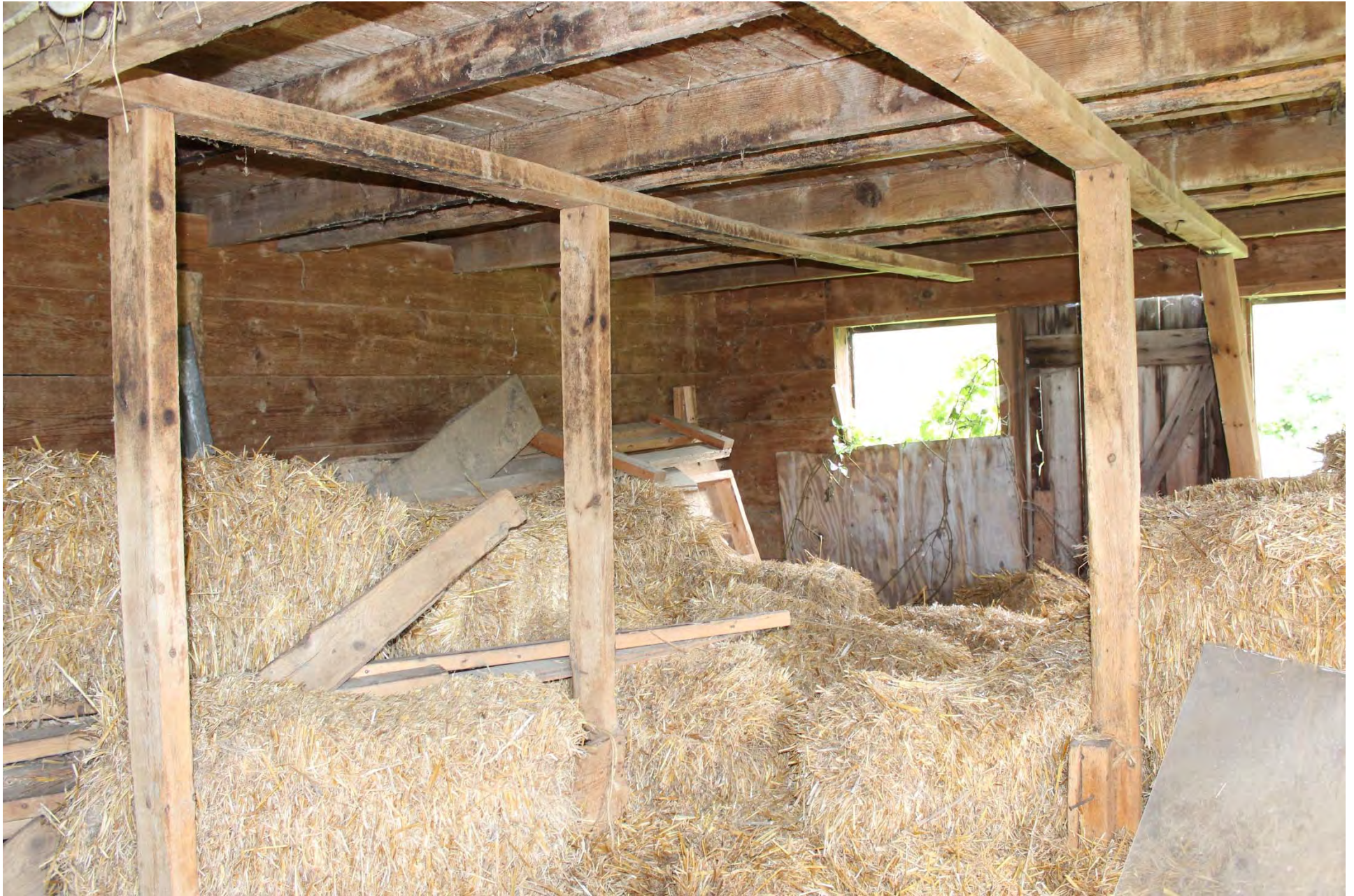
Photo 30. Interior of the lower level of the poultry house.
