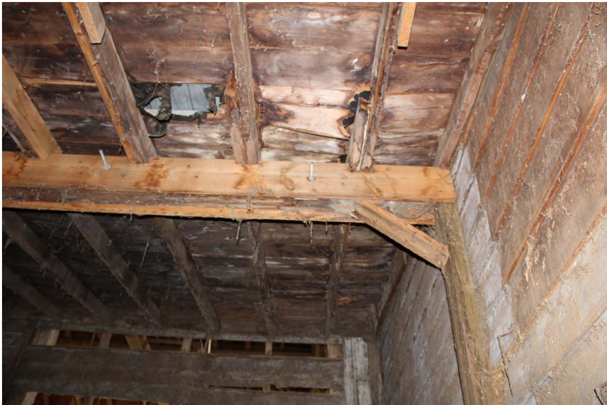
Photo 23. View of sistered and braced rafter and roof repair in the shed addition.
