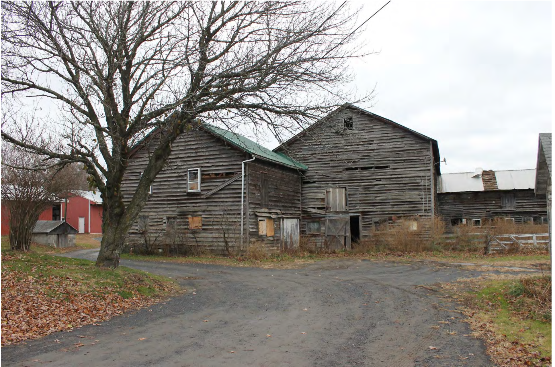
Photo 1. View of horse barn on the left and the original main barn on the right.
