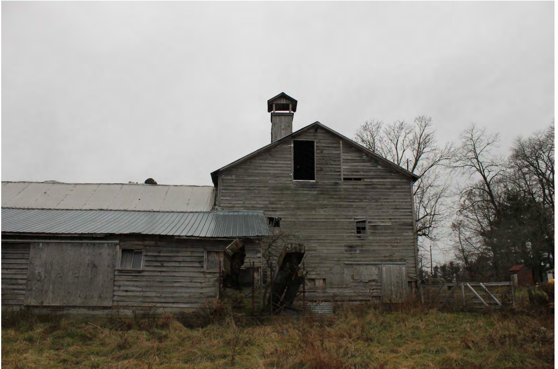
Photo 3. Northern façade of the main dairy barn showing its distinctive wooden vent and a 20 th century shed addition to the left.
