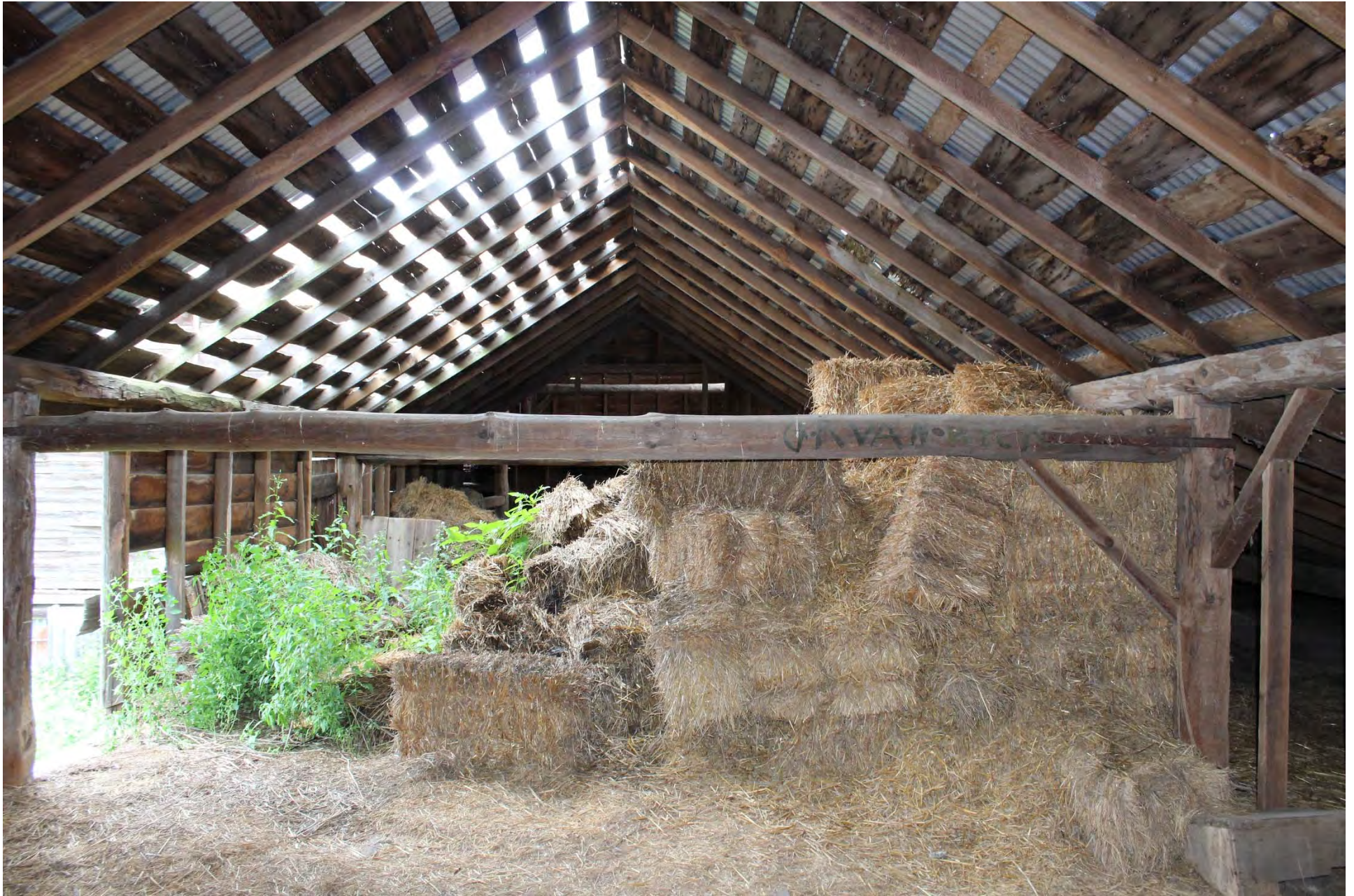
Photo 14. View of framing member in the upper story of the 19th century addition. Note the name "G.R. Van Dyck" painted on the crossmember.
