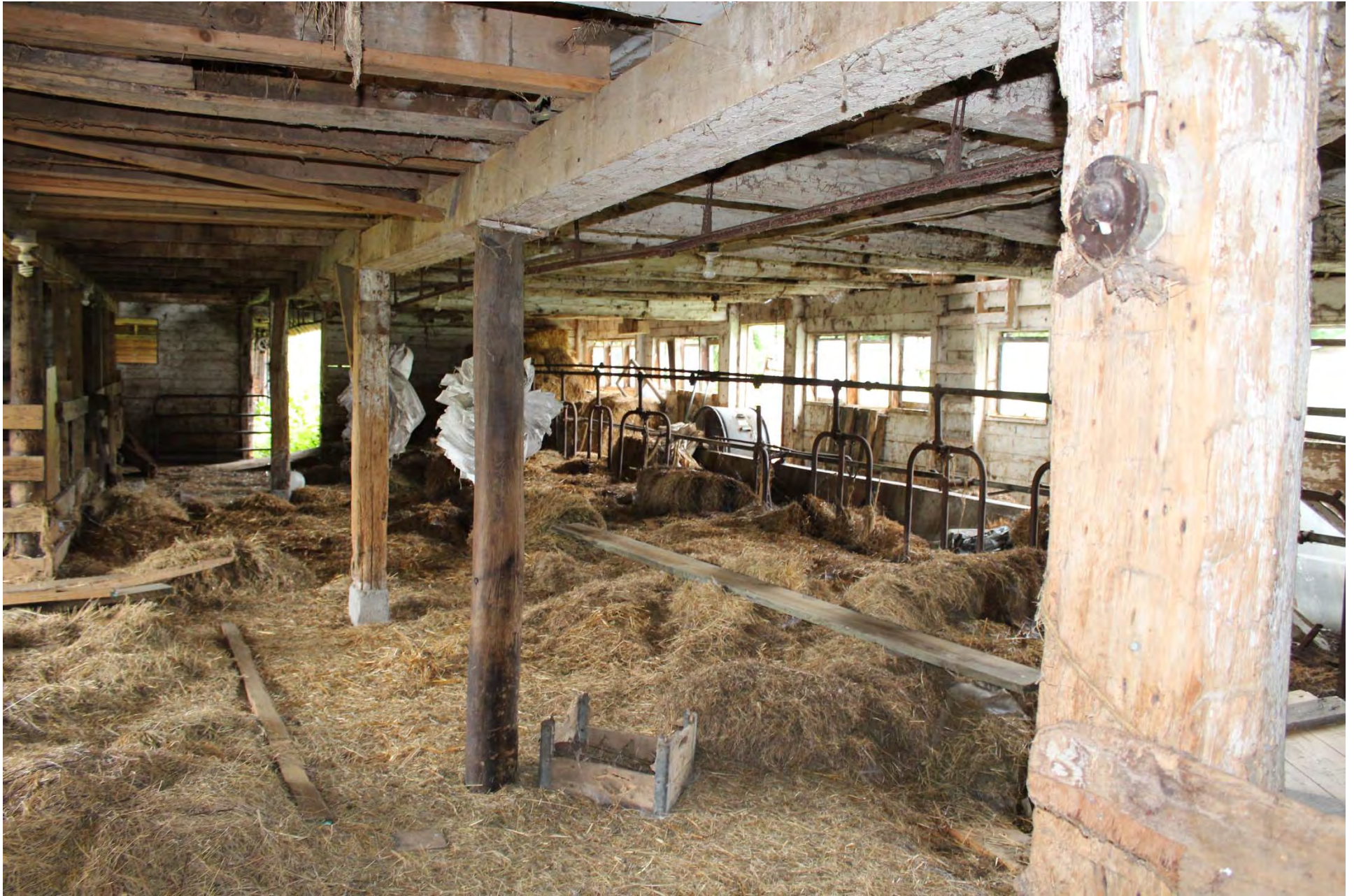
Photo 17. View of dairy stanchions on the first floor of the 19th century addition.
