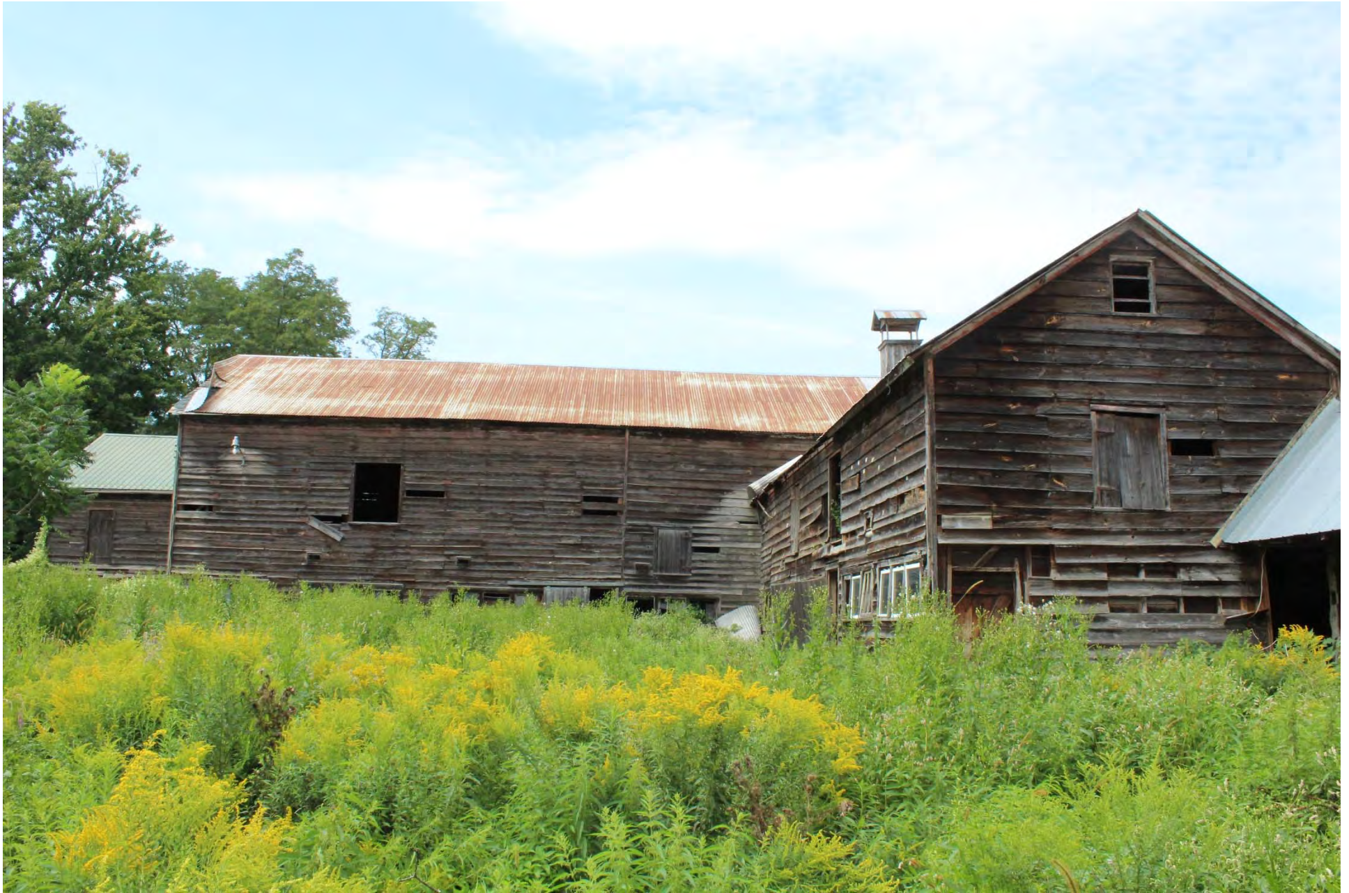
Photo 2. Eastern facade of the oldest portion of the main barn complex. Note the tall vent in the rear of the structure.
