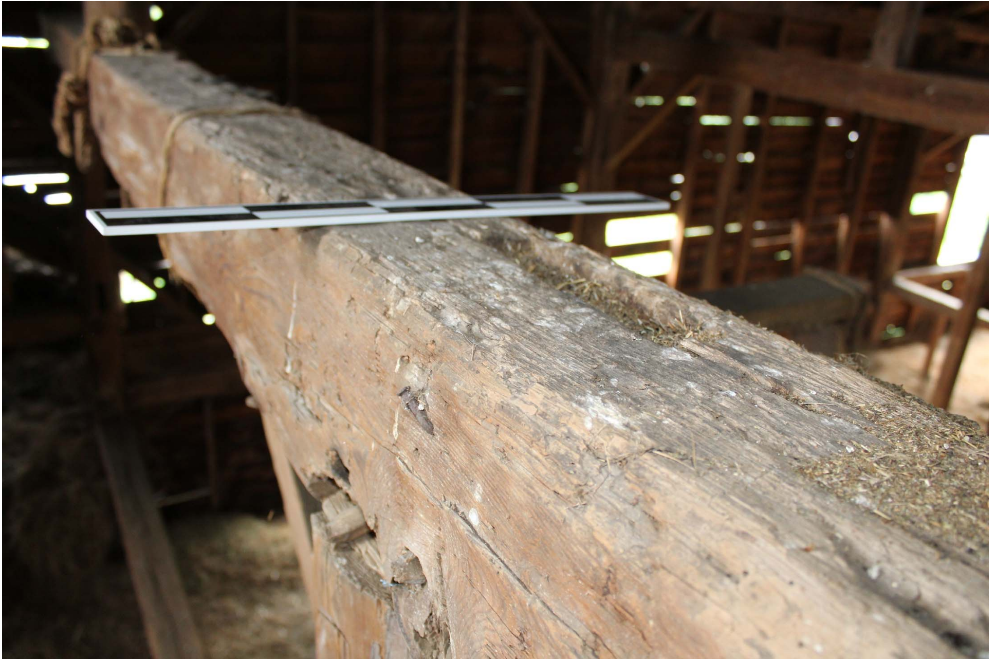
Photo 12. View of mortice where a central crown post original extended to the rafter plate.
