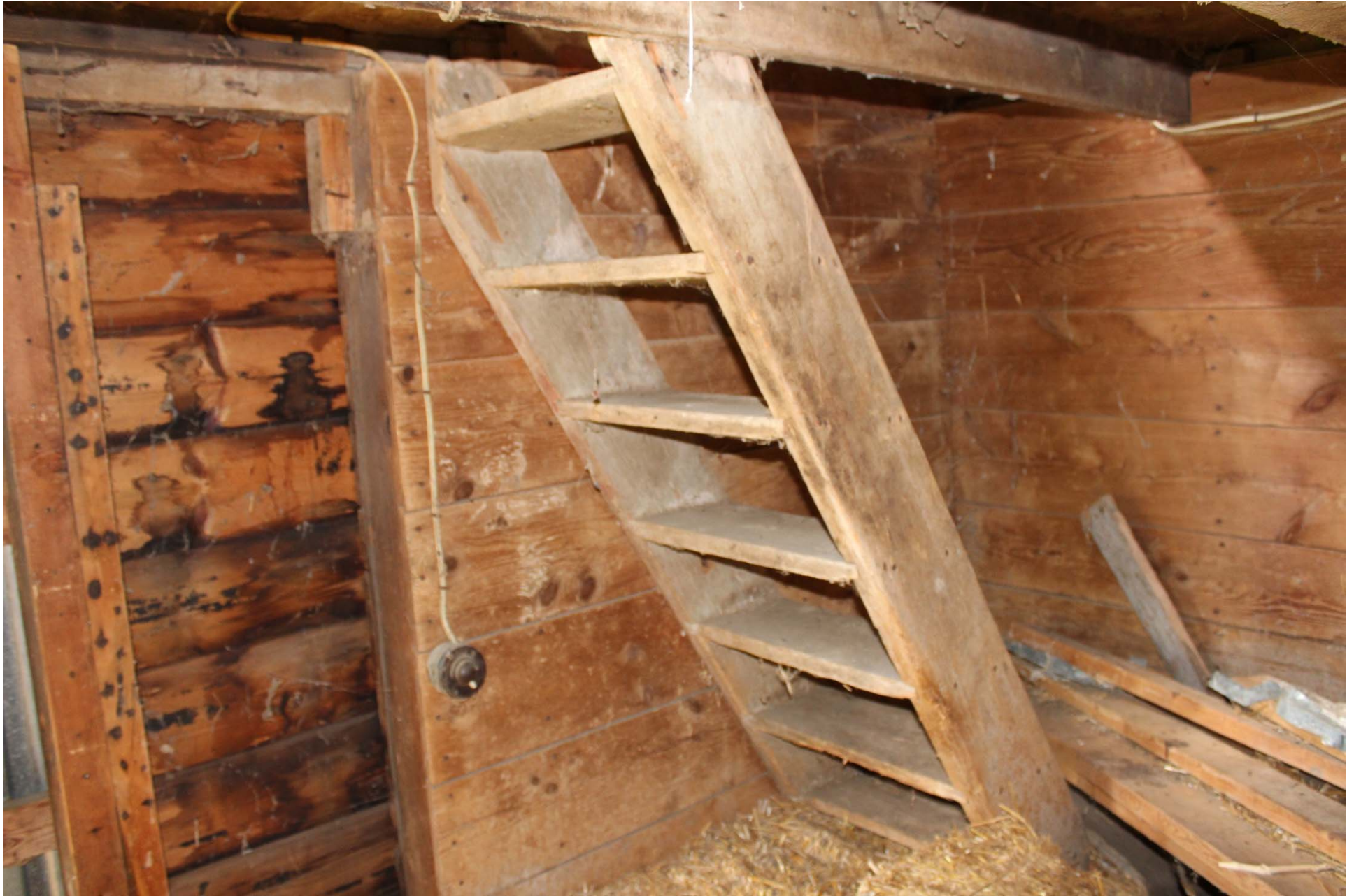
Photo 31. View of stair leading to the upper level of the poultry house.
