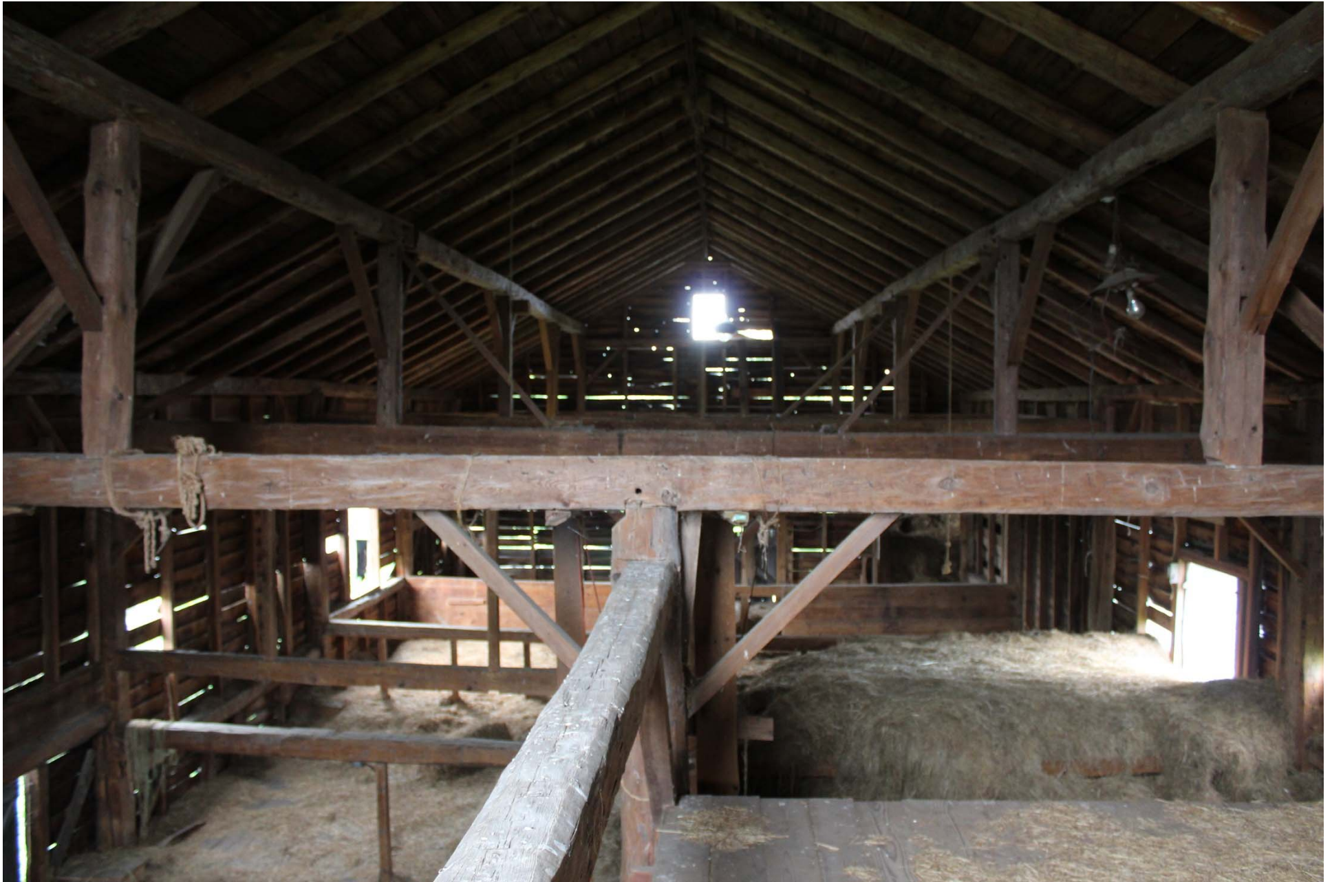
Photo 11. View of Queens truss framing members in the original portion of the main dairy barn.
