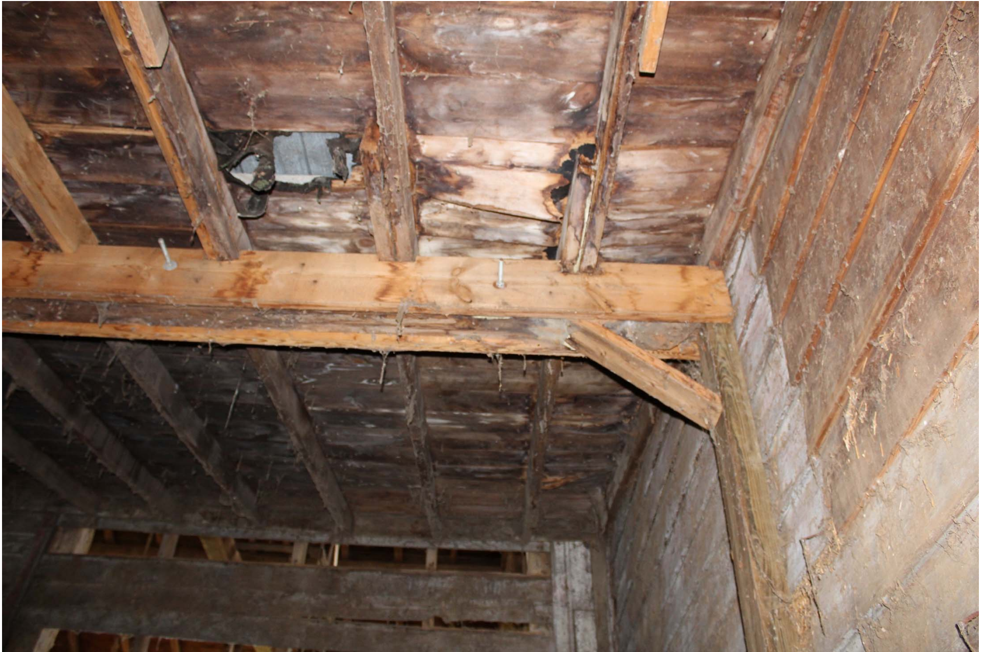
Photo 24. View of sistered and braced rafter and roof repair in the shed addition.
