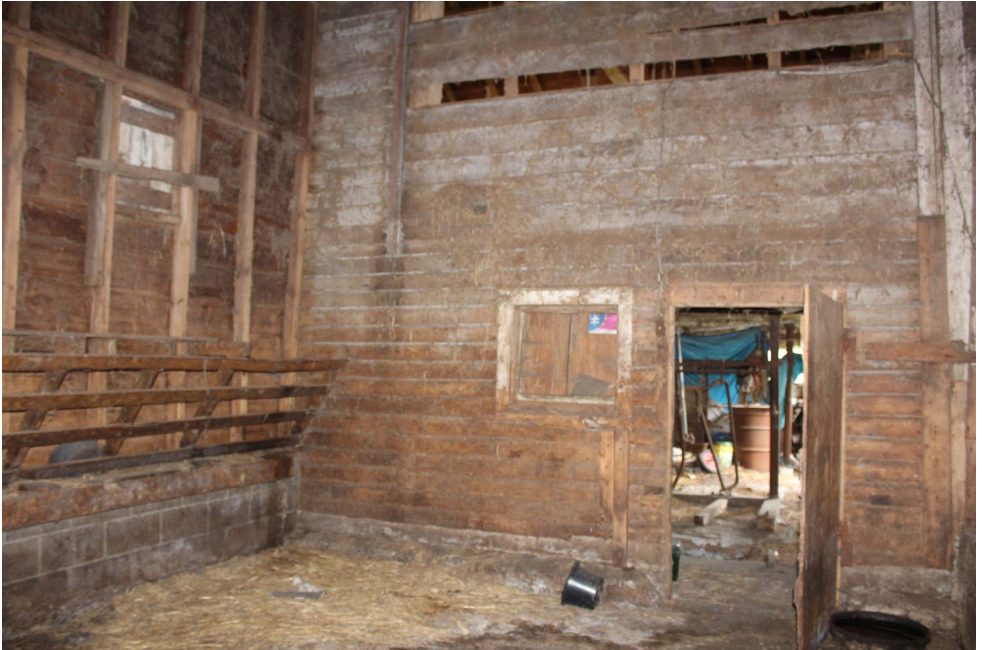
Photo 23. View of the interior of the shed roof addition.
