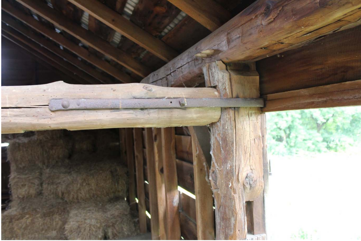
Photo 13. View of wrought iron strap used to connect the purlins to the wall post.
