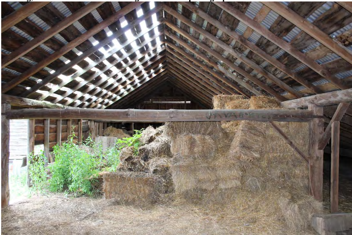
Photo 12. View of framing member in the upper story of the 19 th century addition. Note the name "G.R. Van Dyck" painted on the crossmember.
