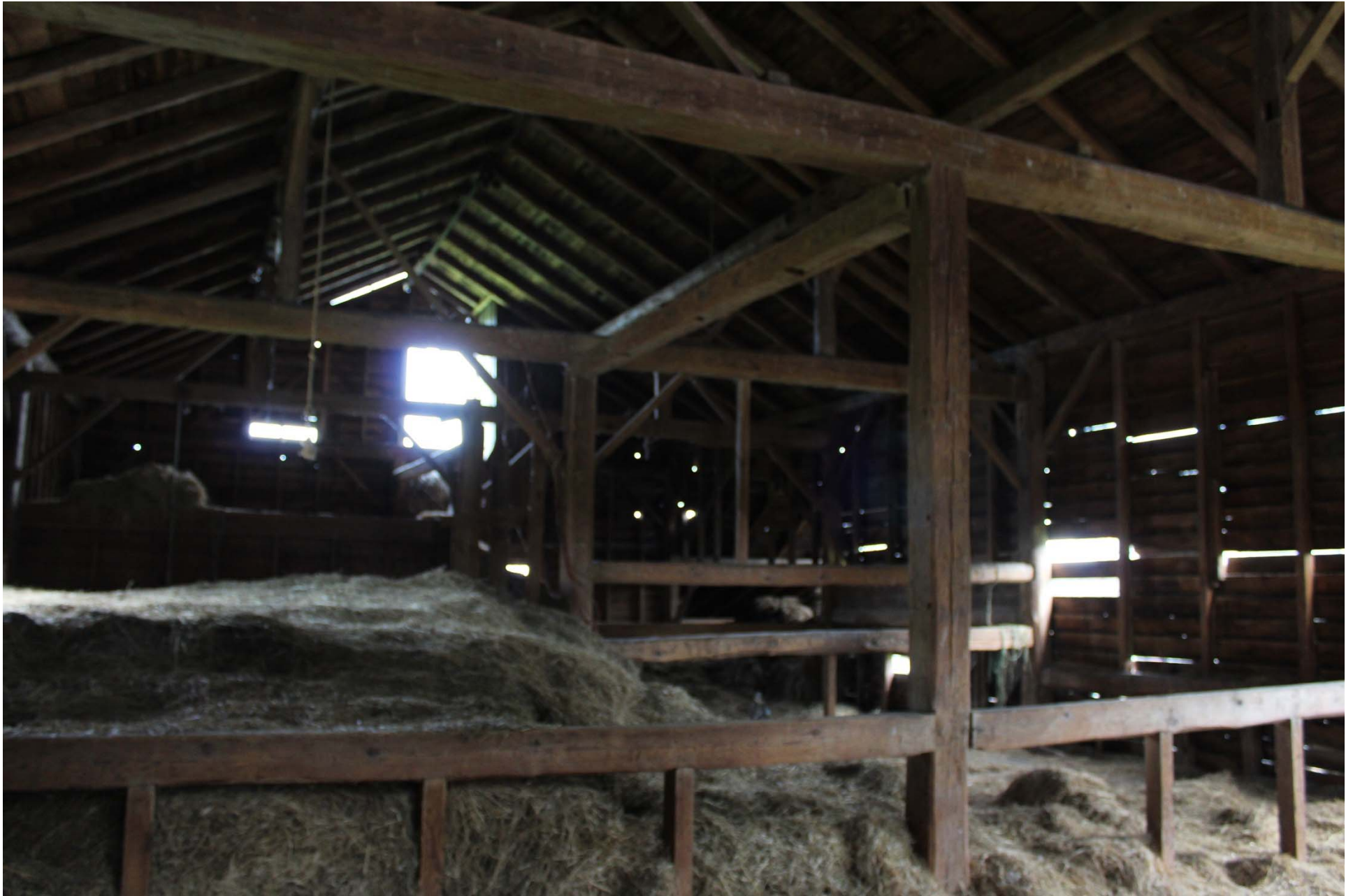
Photo 10. Interior of the main barn showing the truss system and divided hay mows.
