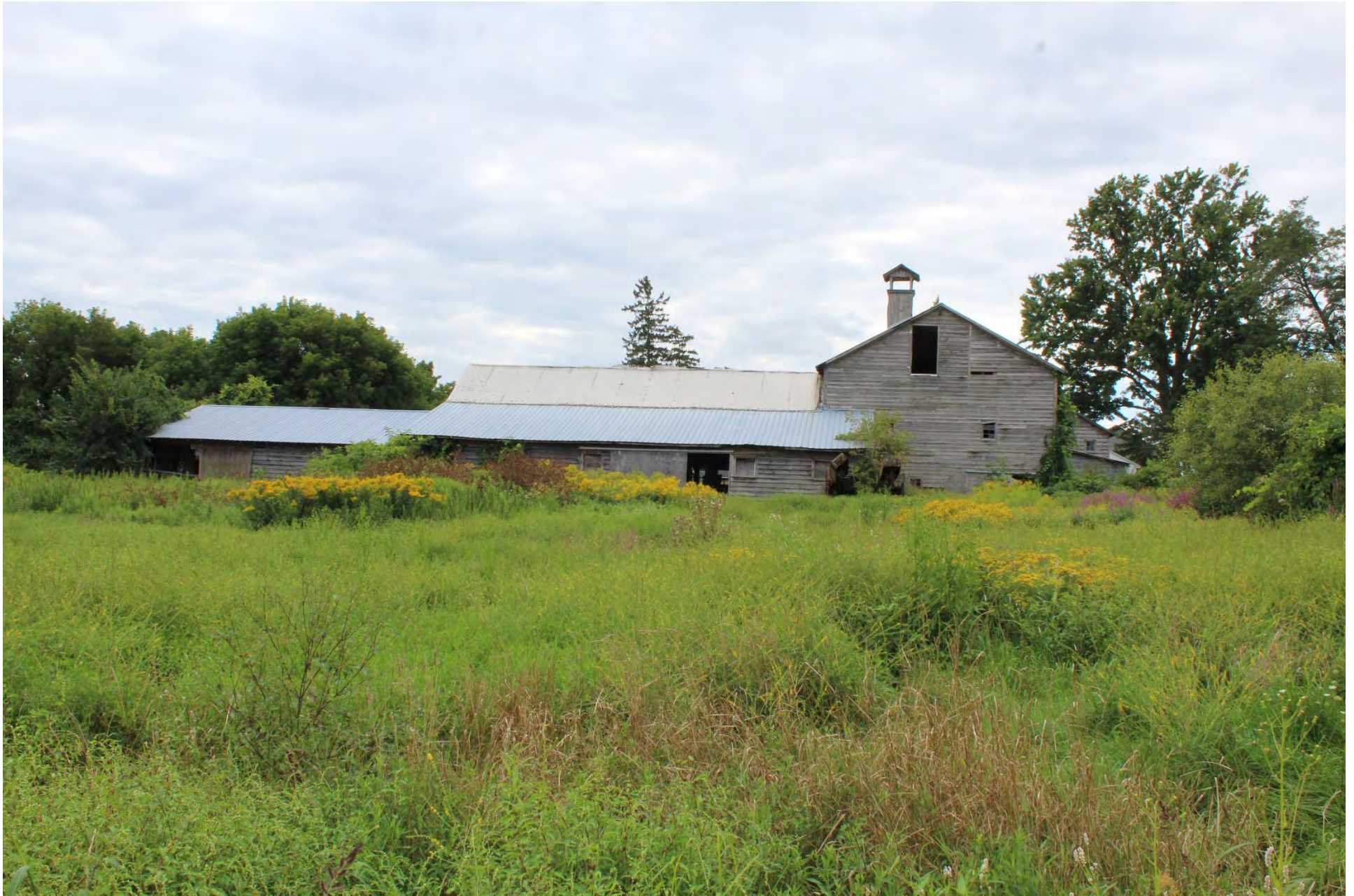
Photo 6. View of the complete north façade of the dairy barn complex.
