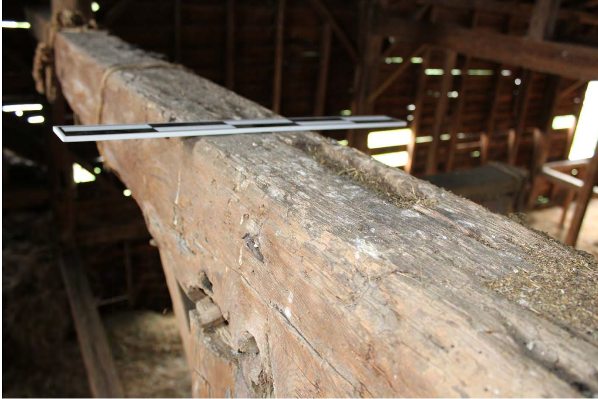
Photo 8. View of mortise where a central crown post original extended to the rafter plate.
