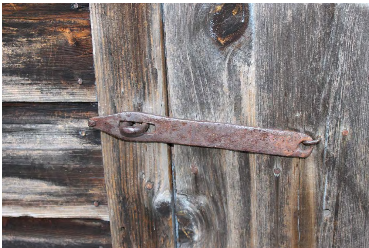
Photo 31. Detail of hand wrought hardware on the eastern façade of the poultry house.
