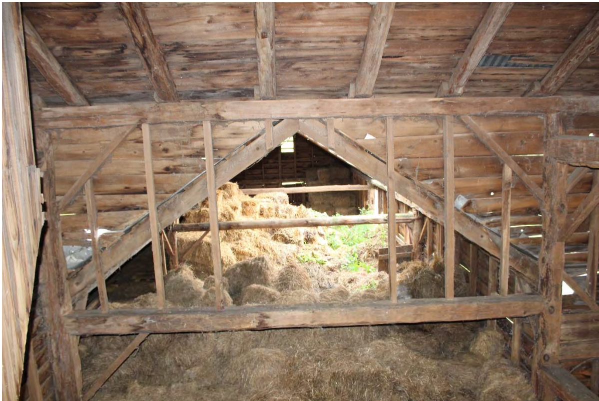
Photo 14. View of the 19 th century addition from the main dairy barn. Note how the vertical framing of the original barn was cut to allow entry into the new addition.
