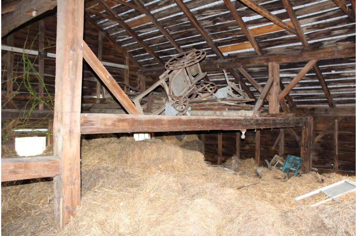
Photo 20. View of framing in the upper story of the horse barn. Note asymmetrical framing and partial H bent at left.
