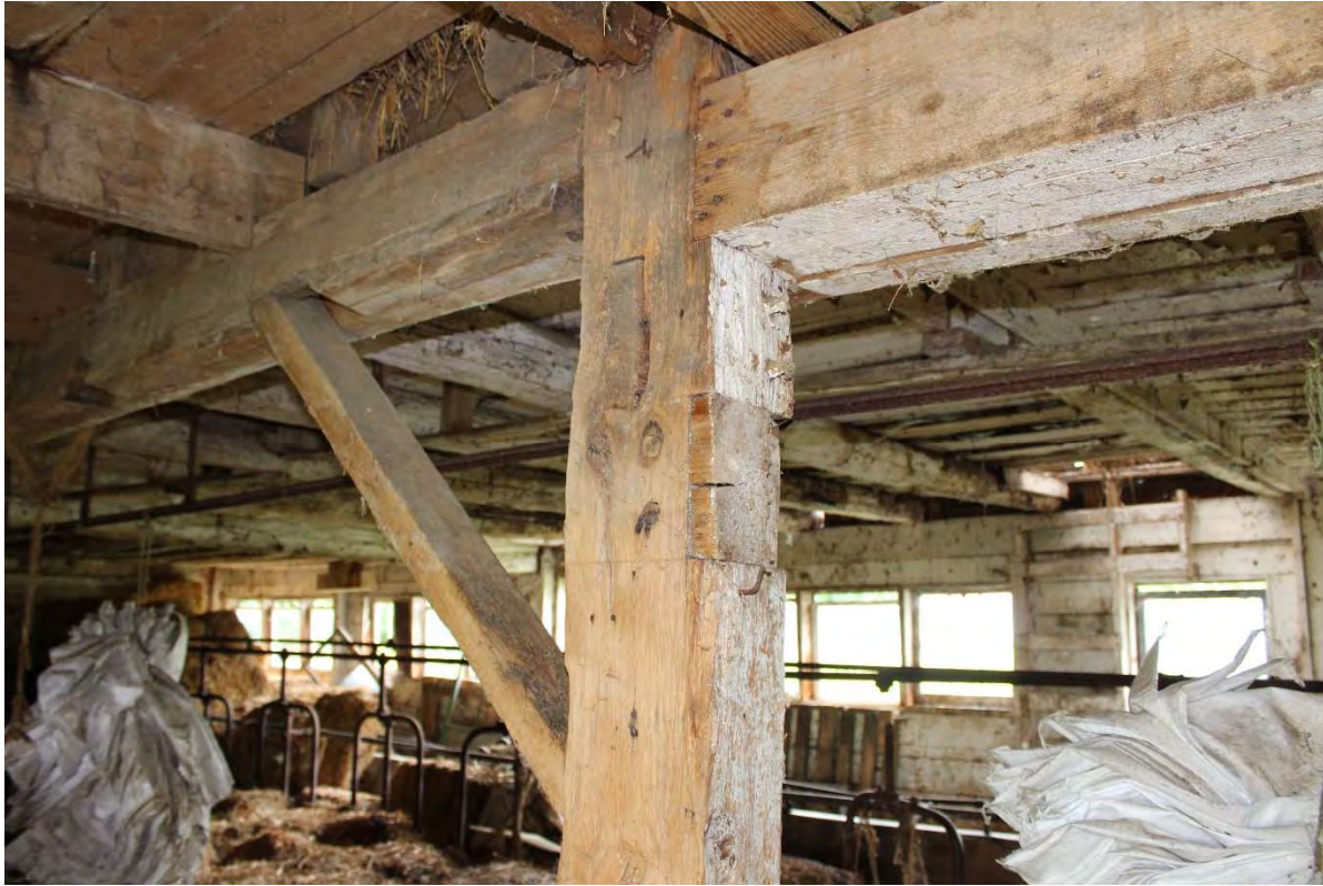
Photo 17. View of timber framed joint with brace in the first floor of the main dairy barn.
