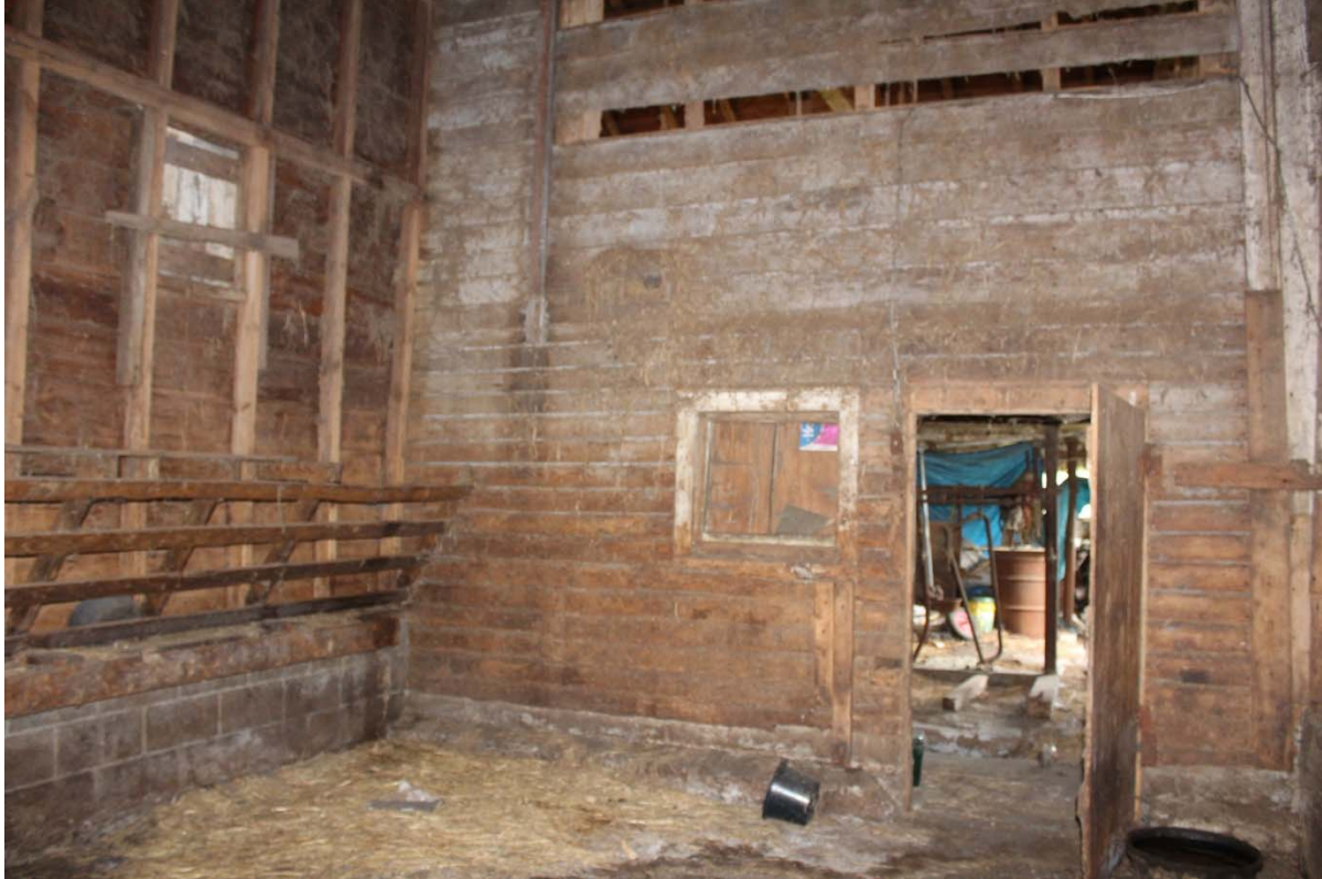
Photo 22. View of the interior of the shed roof addition.
