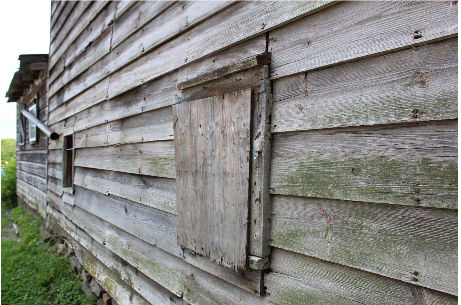
Photo 8. View of window frame and lintel on the west façade of the main dairy barn.
