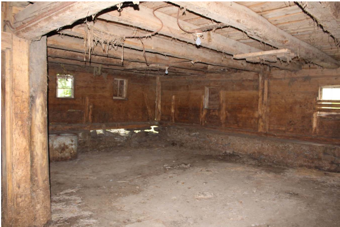
Photo 21. View of the first floor of the horse barn showing the stone foundation.
