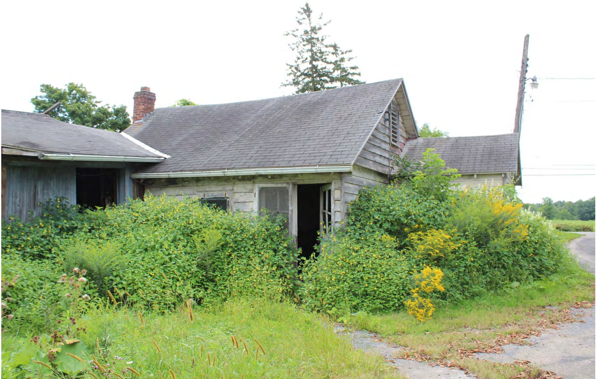
Photo 34. Oldest wood framed portion of the creamery/bottling works building.
