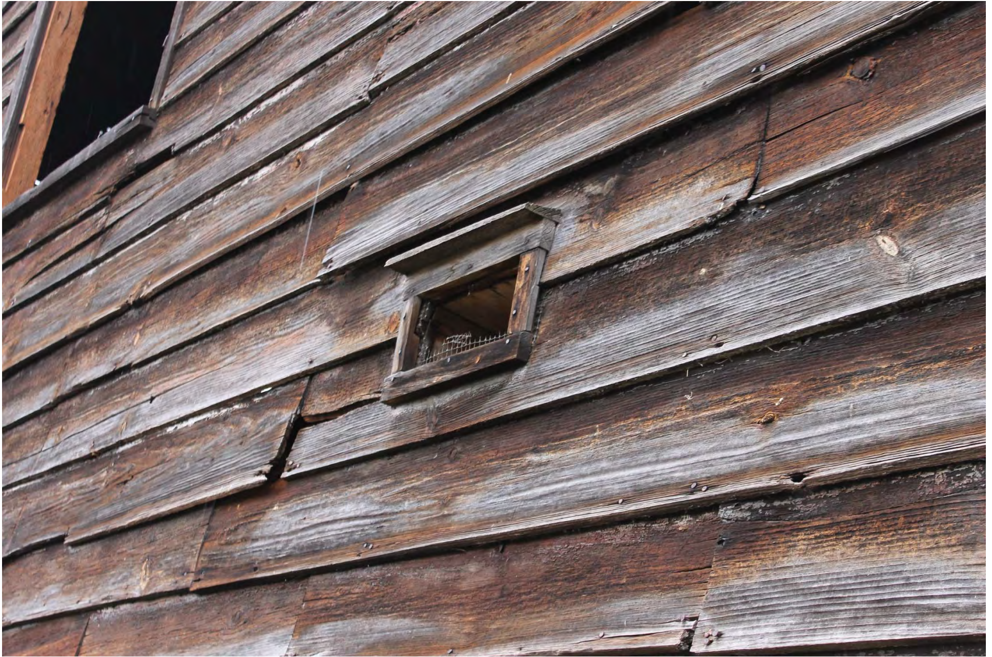
Photo 9. Distinctive vent with eaves and surrounds on the west façade of the main dairy barn.
