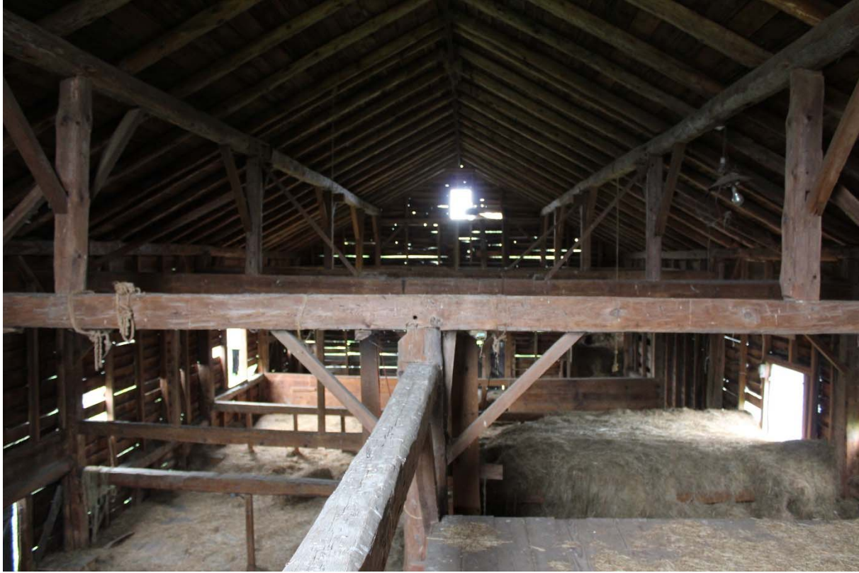
Photo 7. View of Queens truss framing members in the original portion of the main dairy barn.
