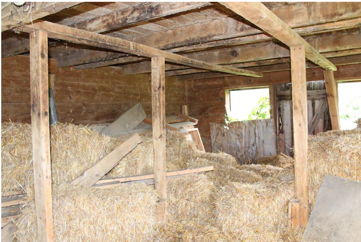
Photo 28. Interior of the lower level of the poultry house.
