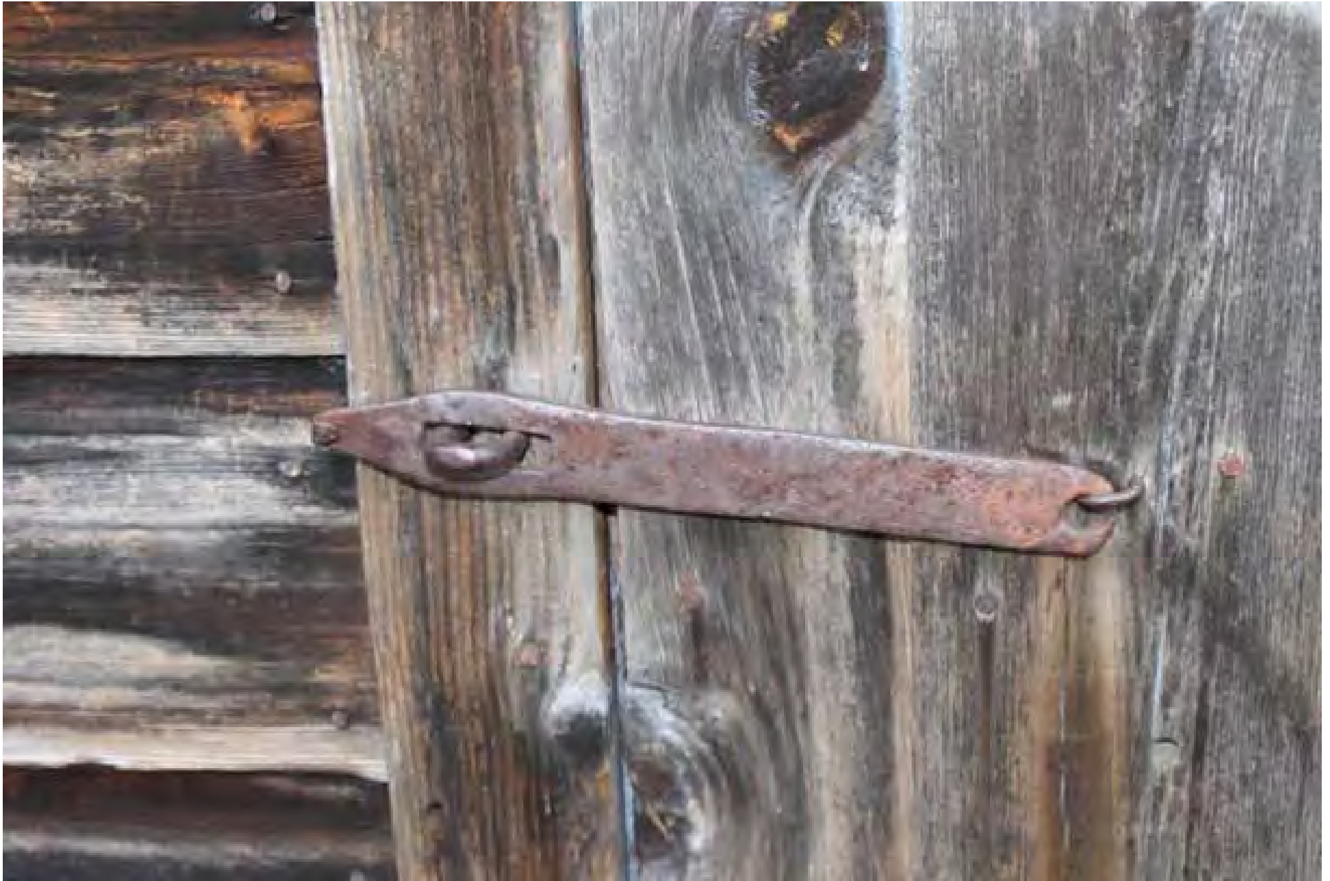
Photo 29. Detail of hand wrought hardware on the eastern façade of the poultry house.
