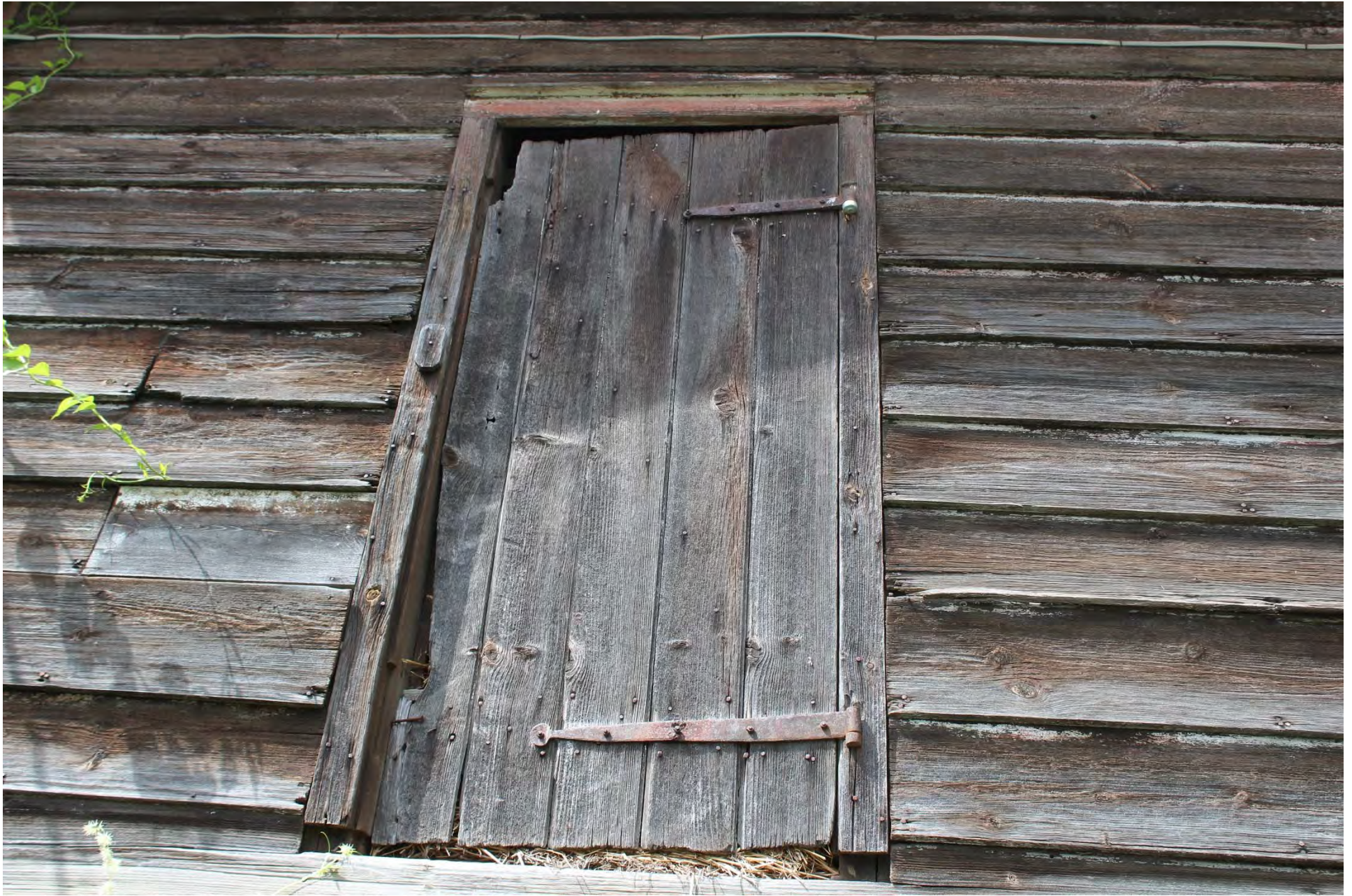
Photo 7. Door with wrought iron strap hinges on the eastern façade of the horse barn.
