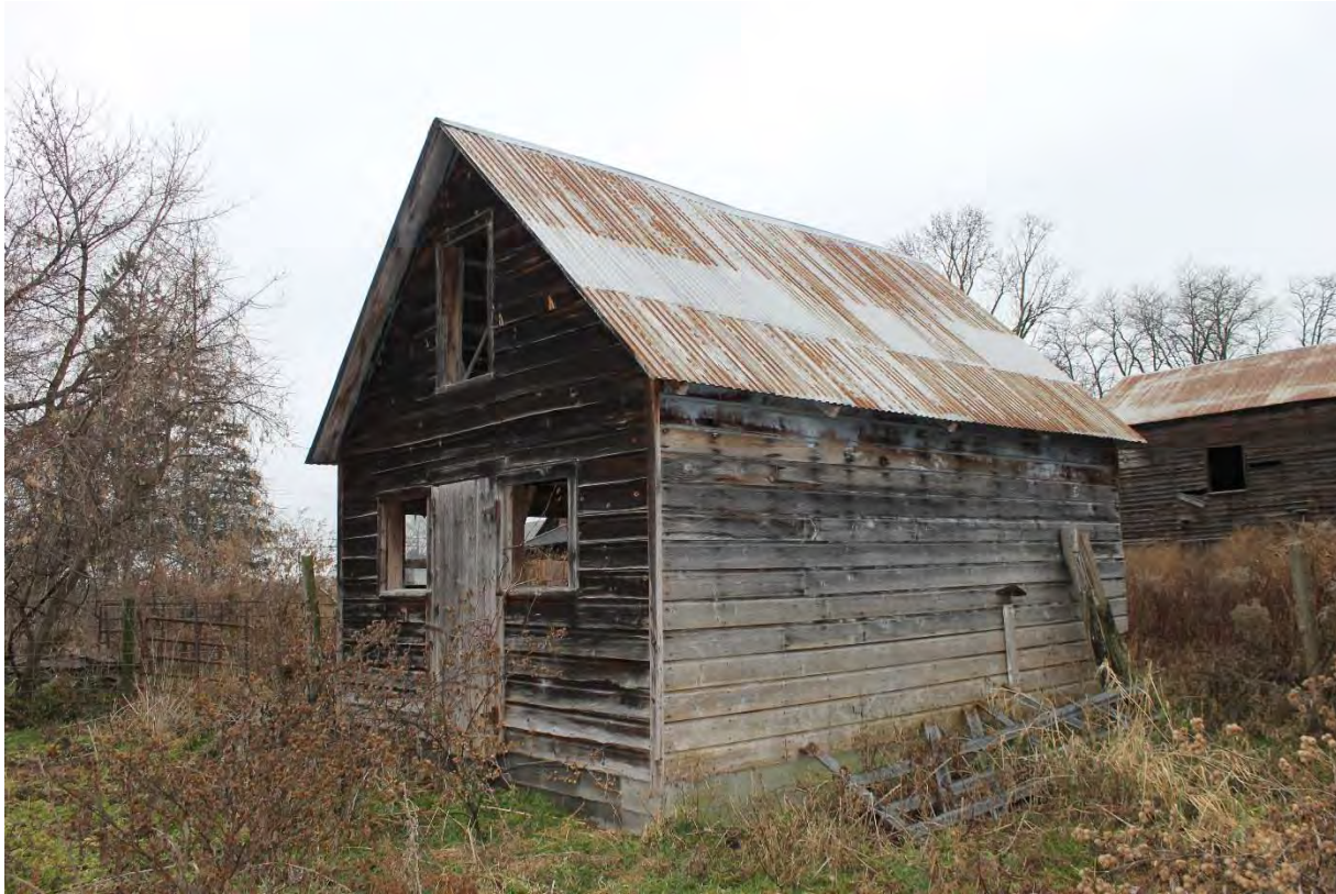
Photo 27. Northeast corner of the poultry house at the Houghtaling/Klienke farm complex.
