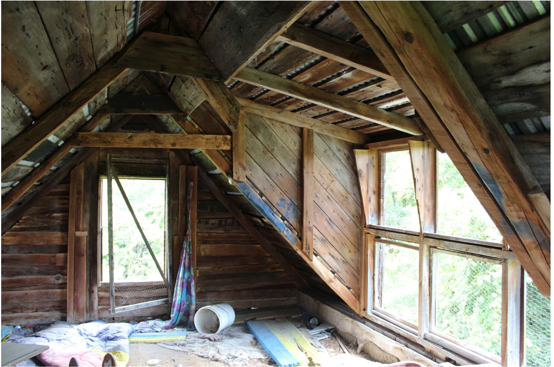
Photo 32. View of the interior of the upper story of the poultry house.
