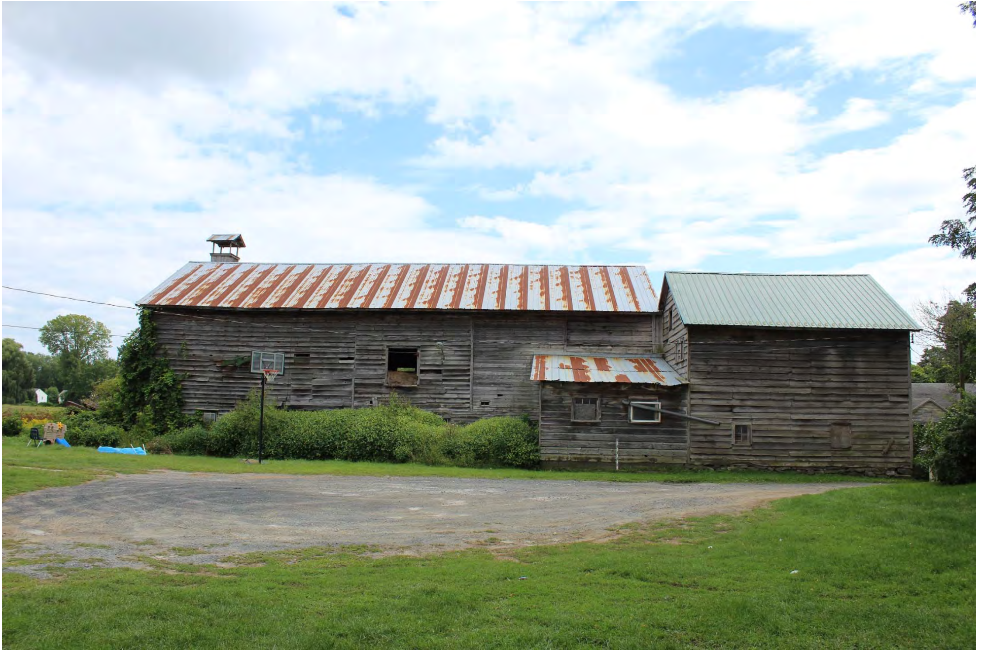
Photo 5. Western facade of the oldest portion of the main barn complex. Note horse barn and 20th century shed addition in the right part of the photograph.
