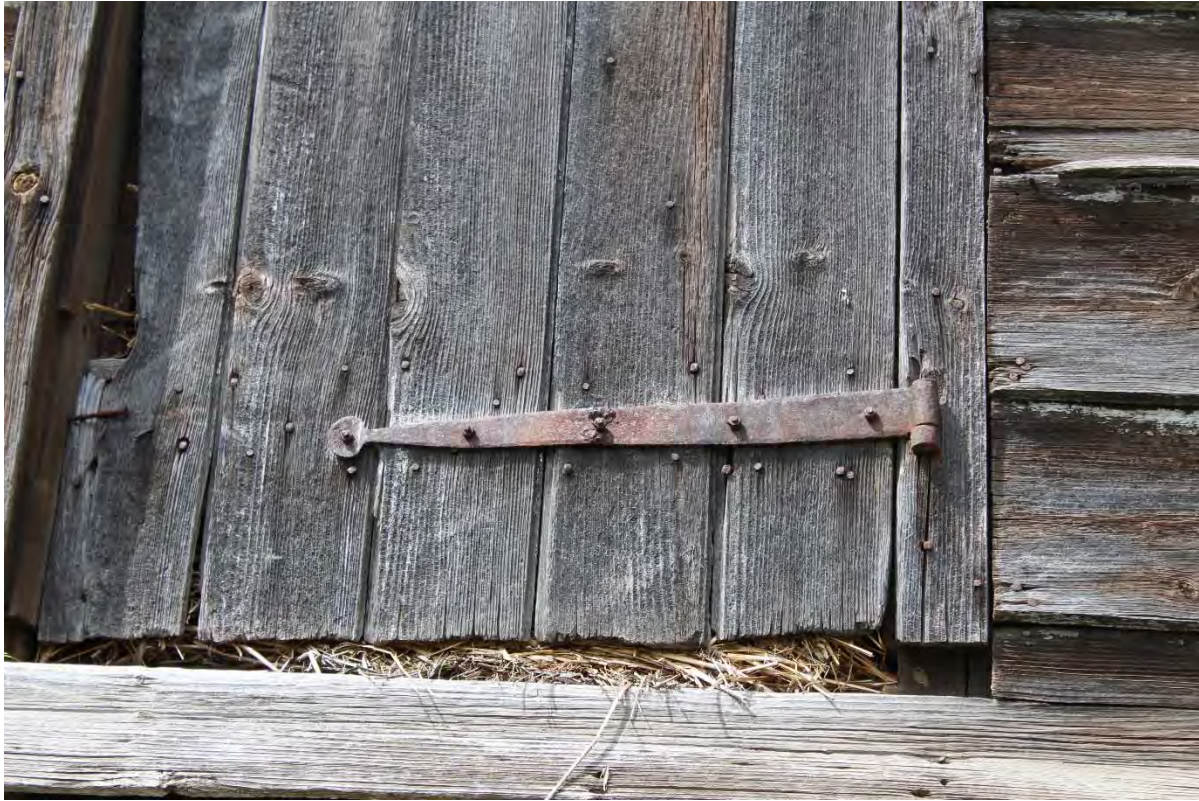
Photo 10. Hand wrought strap hinge on the exterior of the main dairy barn.
