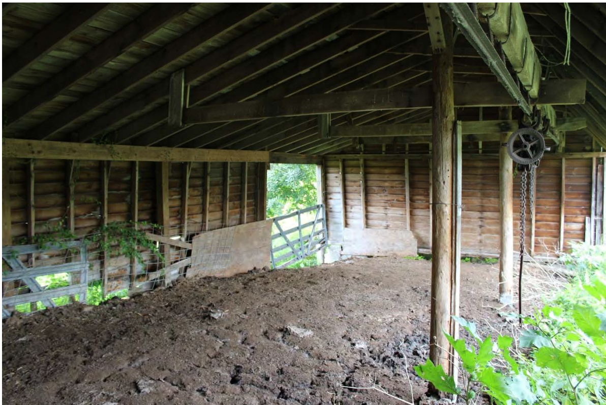
Photo 18. View of shed addition to the east of the 19 th century barn addition. Note the conveyor and above ground track on the right side of the photograph.
