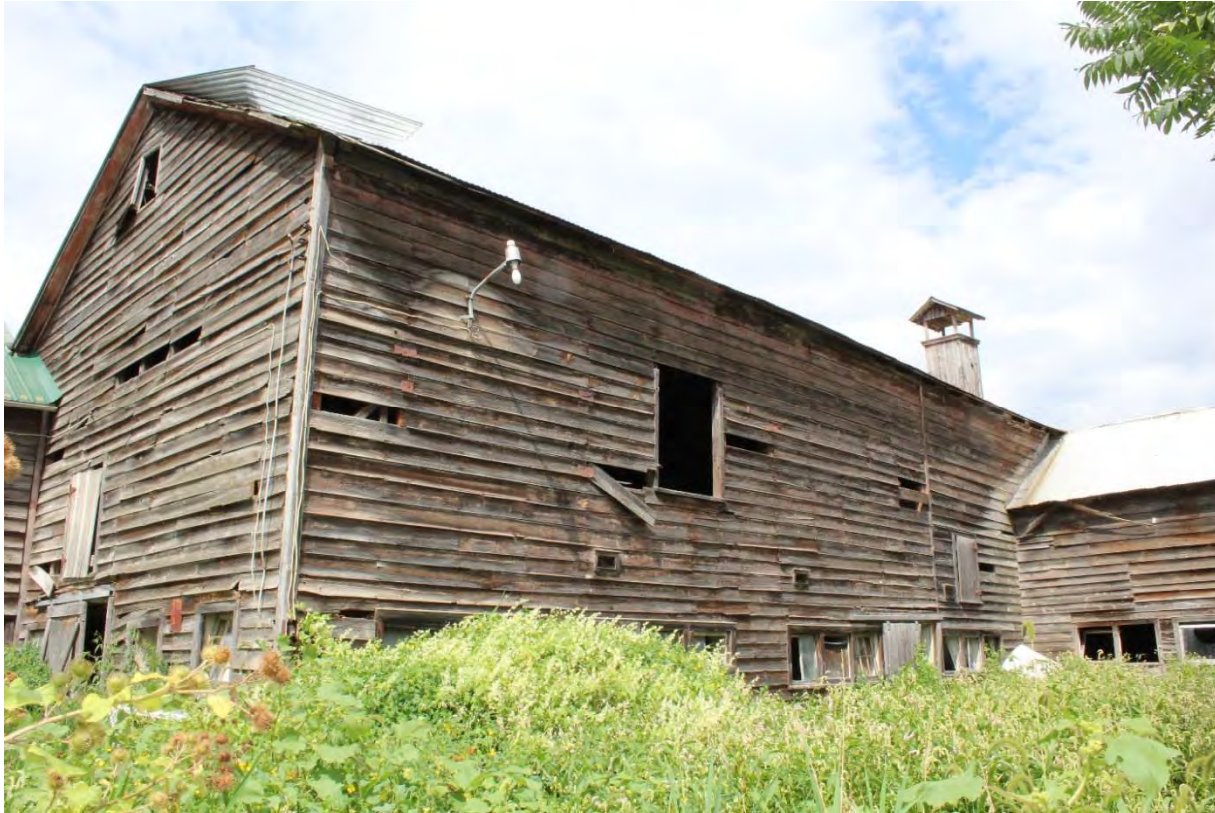
Photo 4. Southwest corner of the oldest portion of the main barn complex. Note the tall vent in the rear of the structure.
