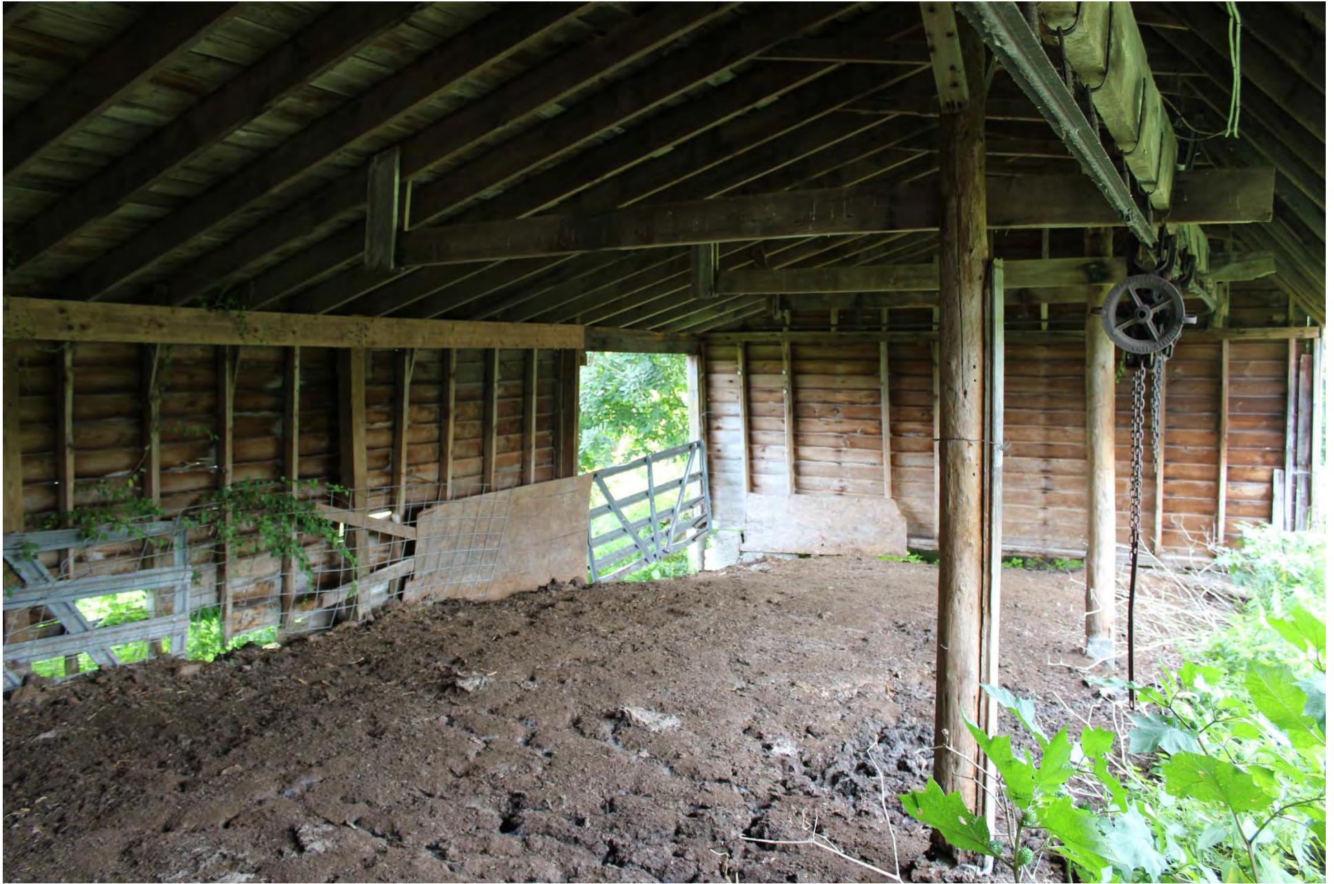
Photo 20. View of shed addition to the east of the 19th century barn addition. Note the conveyor and above ground track on the right side of the photograph.
