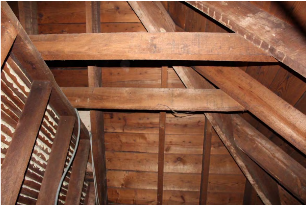
Photo 63. Detail of rafters in a portion of an unfinished attic on the third floor of the Sheriff's Offices.
