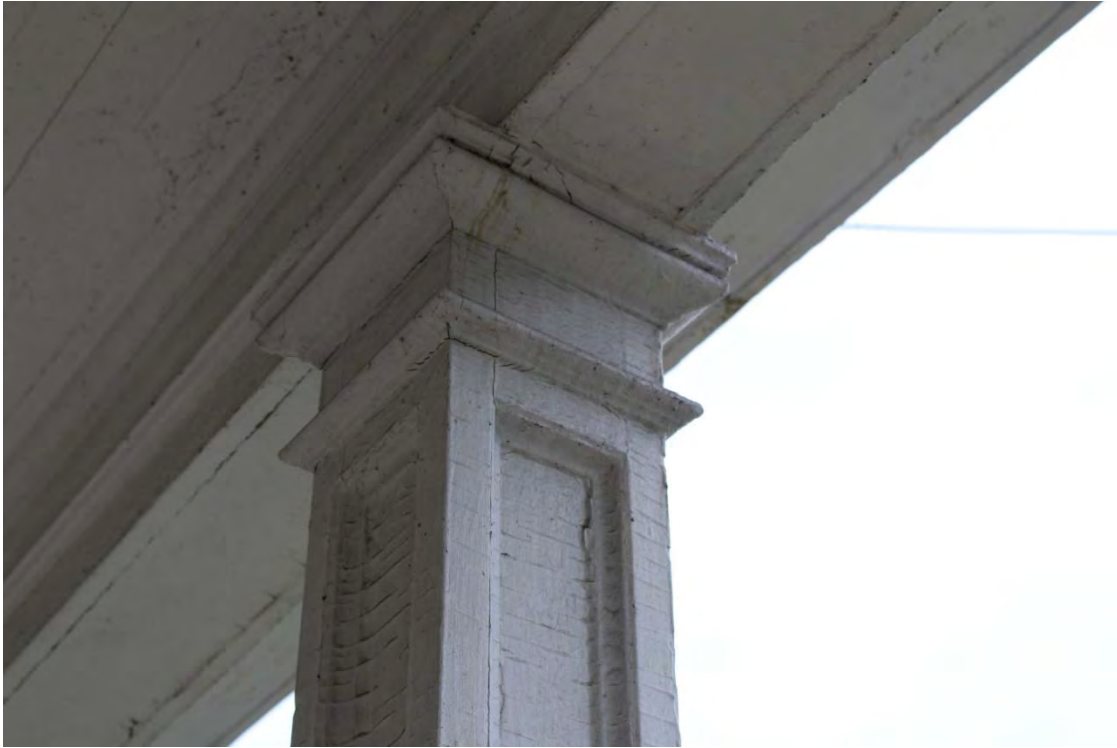
Photo 44. Detail of a Doric column on the front porch of the Sheriff's Offices.
