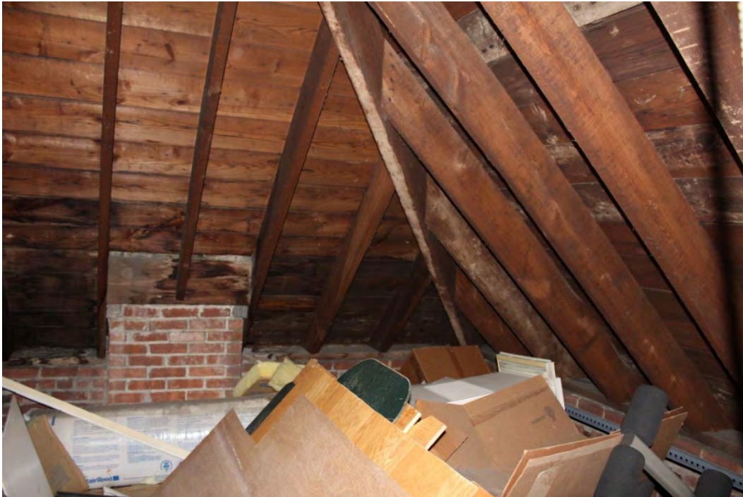
Photo 62. View of a portion of an unfinished attic on the third floor of the Sheriff's Offices.
