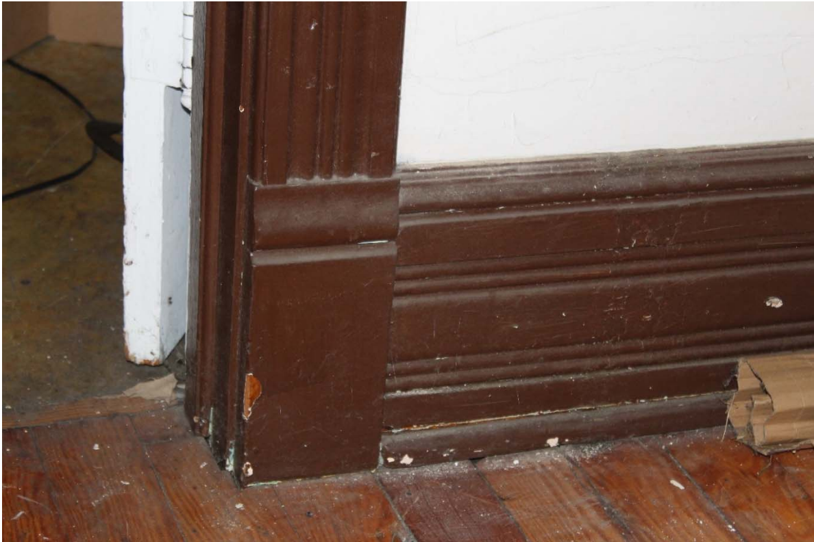
Photo 68. Detail of a door frame and baseboard next to the third-floor restroom in the Sheriff's Offices.
