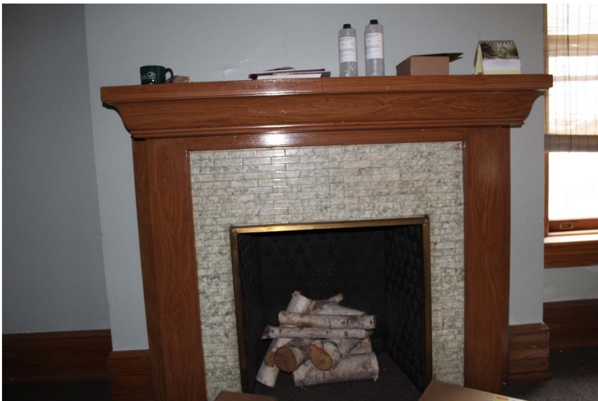
Photo 50. Detail of an office fireplace on the first floor of Sheriff's Offices.
