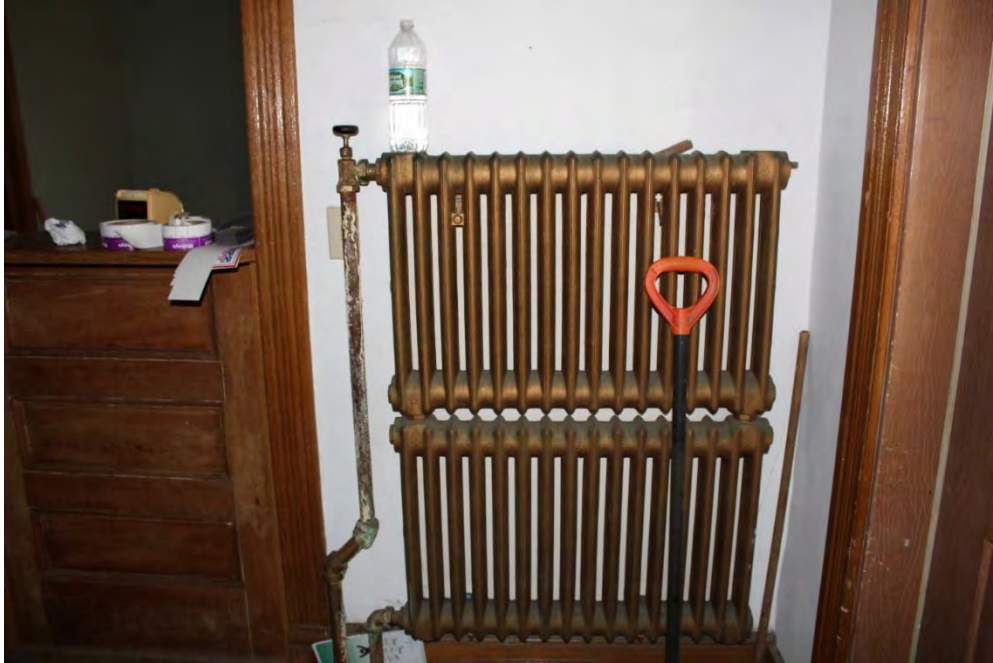
Photo 46. Detail of an original radiator in the Sheriff's Offices.
