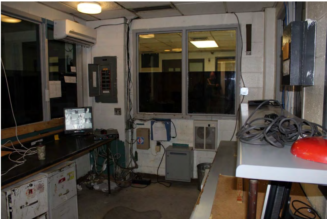
Photo 82. View of the jail control room in D Block.
