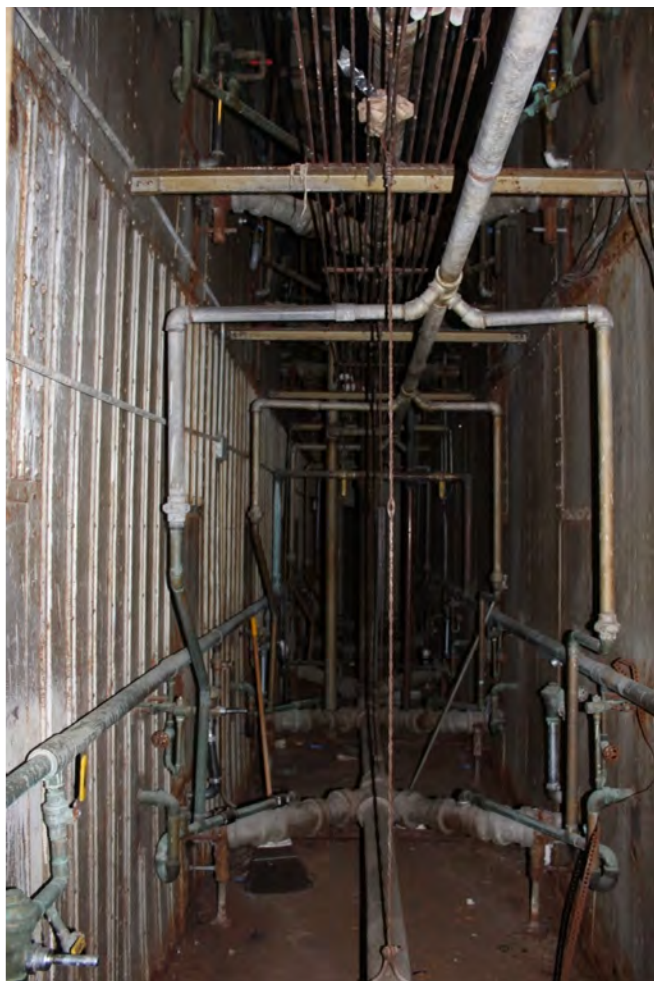
Photo 13. View of the chase in A Block, facing south.
