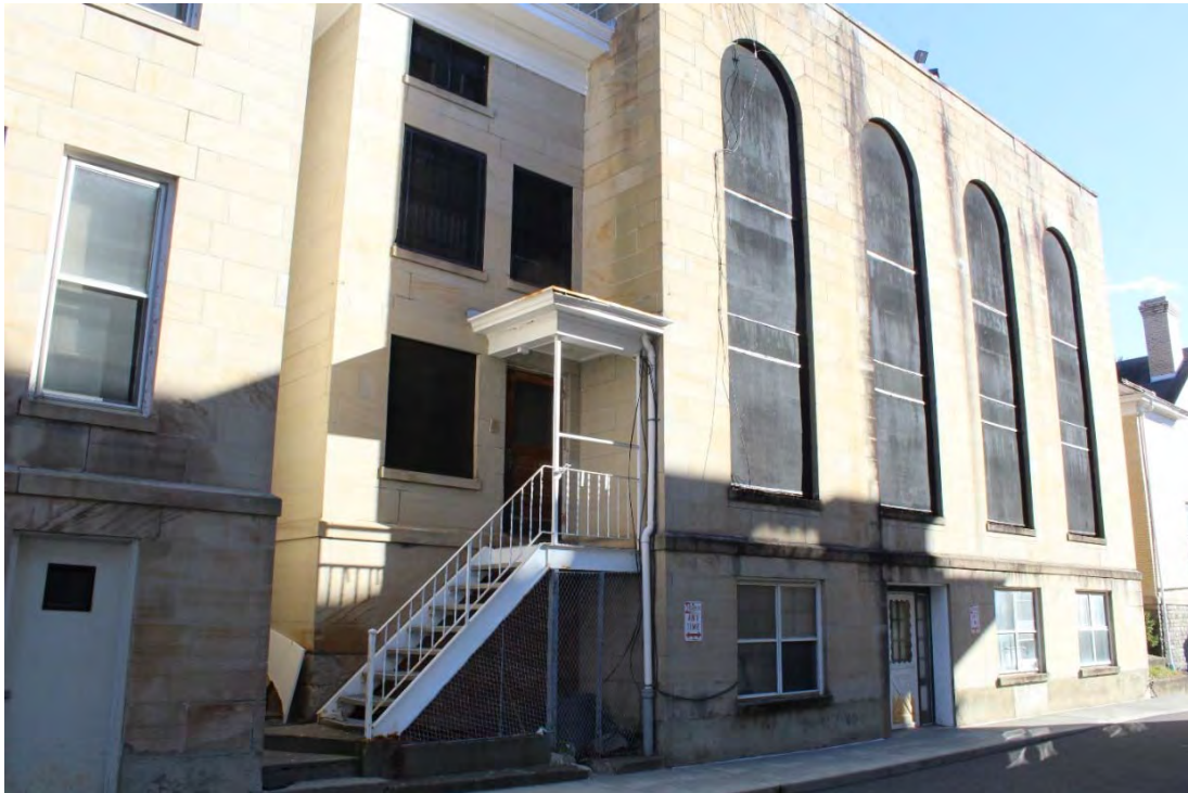
Photo 7. View of the west side of the jail, facing east.
