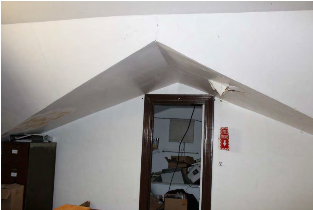
Photo 66. View of shared jail wall and roof peak on third floor of the Sheriff's Offices, facing south.
