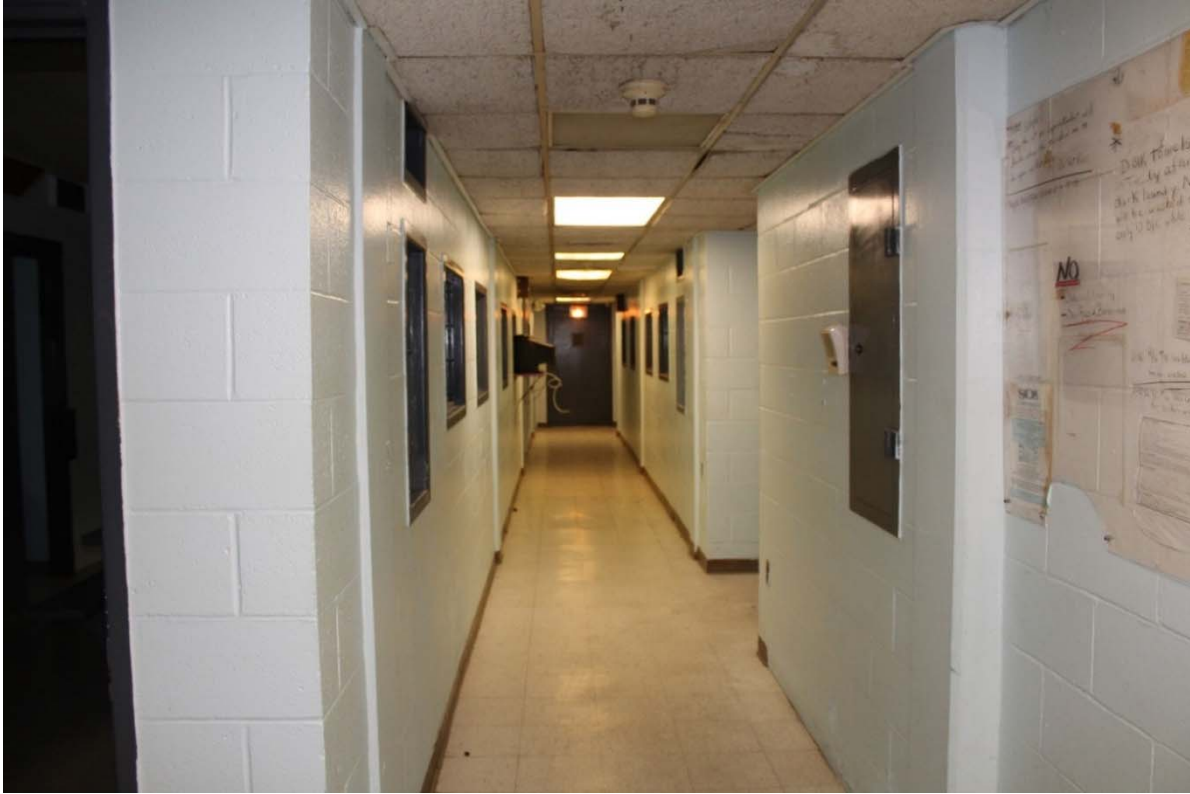
Photo 83. View of the first-floor main hallway in D Block, facing east.
