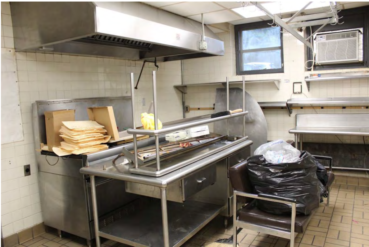
Photo 88. View of the kitchen in D Block, east half.
