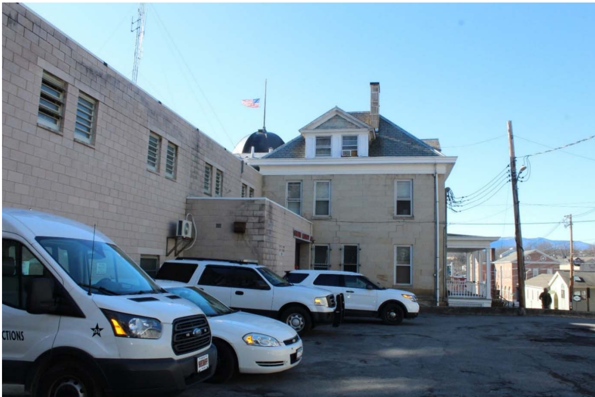
Photo 41. View of the Sheriff's Offices from the main parking lot, facing west.
