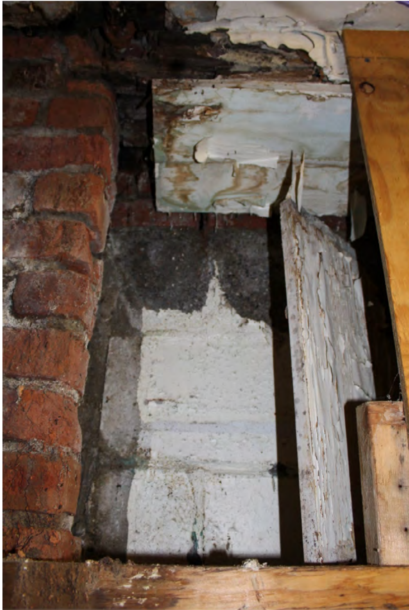
Photo 39. Detail of the juncture of the exterior and interior jail walls in the basement.
