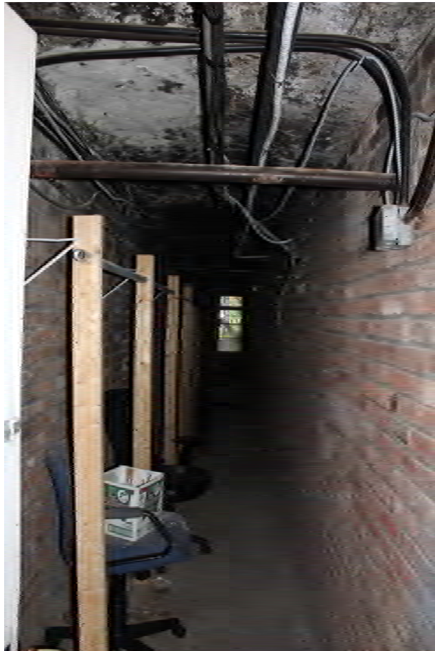
Photo 32. View of the basement alcove located under the chase.
