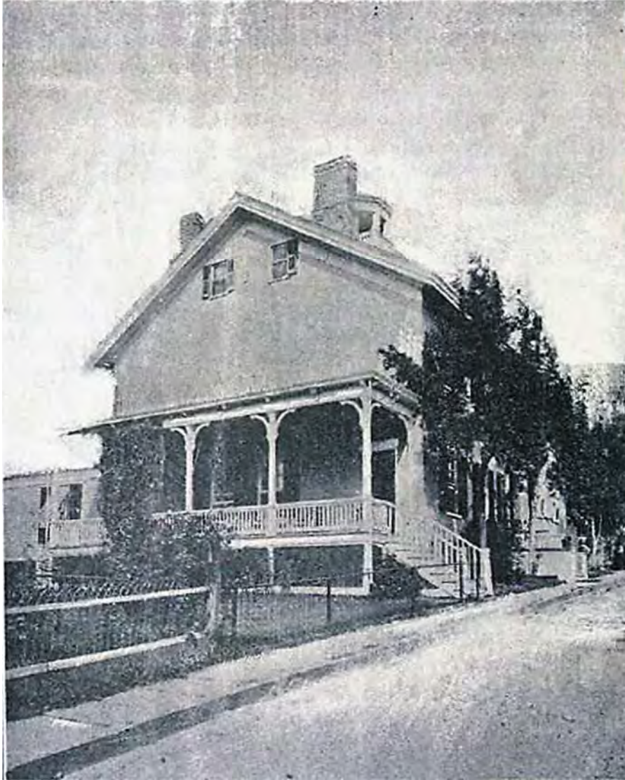
Photo 1. View of the former Greene County Jail/Heidelburgh Inn from Clark St., facing northeast. Photo taken from Gallt 1915.
