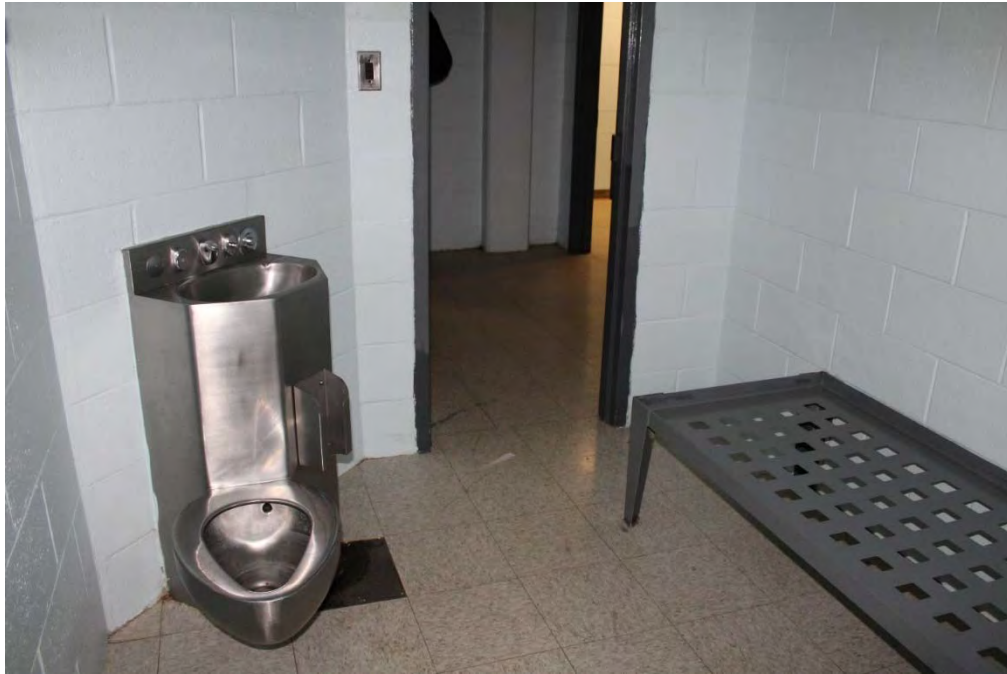
Photo 96. View of the interior of a D Block cell facing out.
