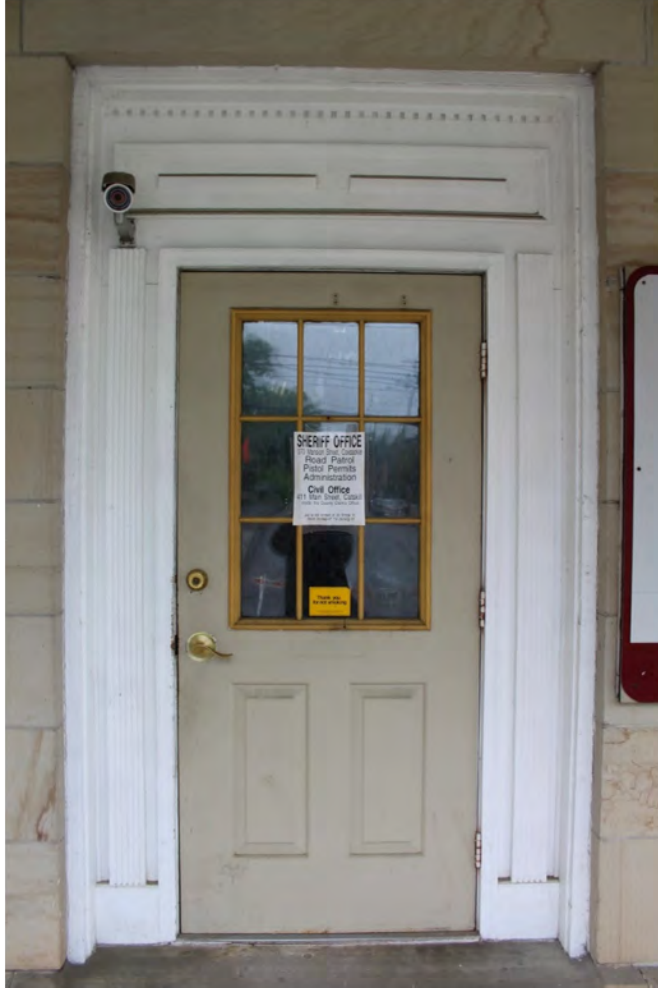
Photo 42. View of the modern front door on the Sheriff's Offices.
