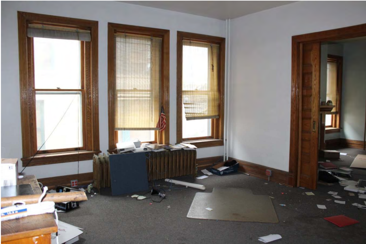
Photo 49. View of an office on southwest corner of the Sheriff's Offices.
