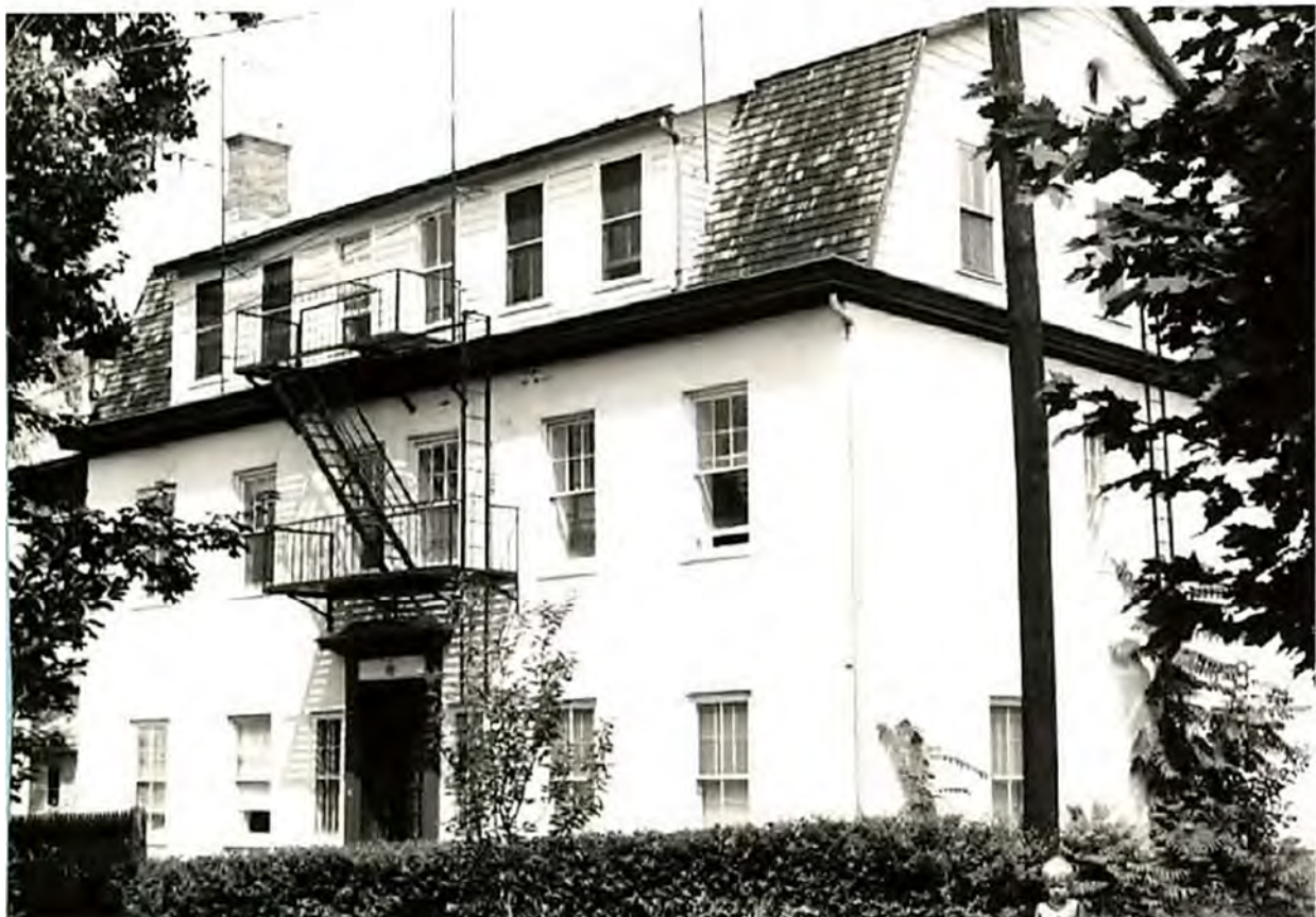
Photo 2. View of the former Greene County Jail/Heidelburgh Inn from Clark St., facing southeast. Photo taken from Flanagan 1980.
