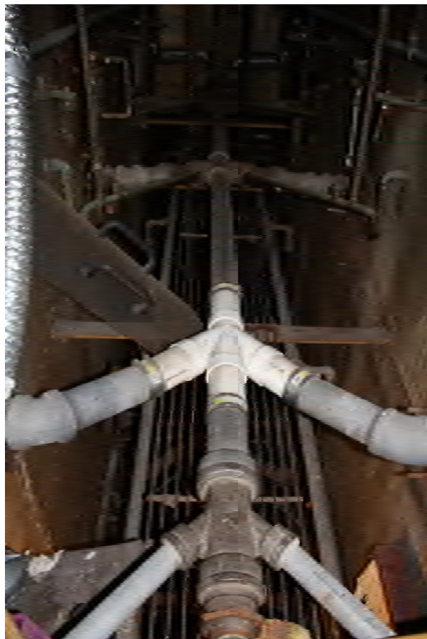
Photo 28. View of the C Block chase, facing south.
