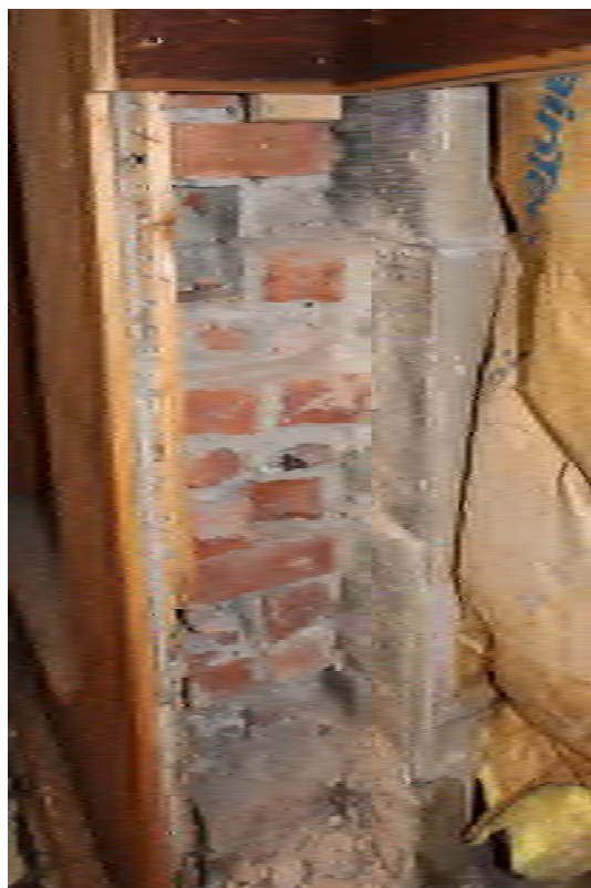
Photo 73. Detail of a wall showing the exterior Ohio sandstone wall and interior brick walls in the east wall of the basement in Sheriff's Offices.
