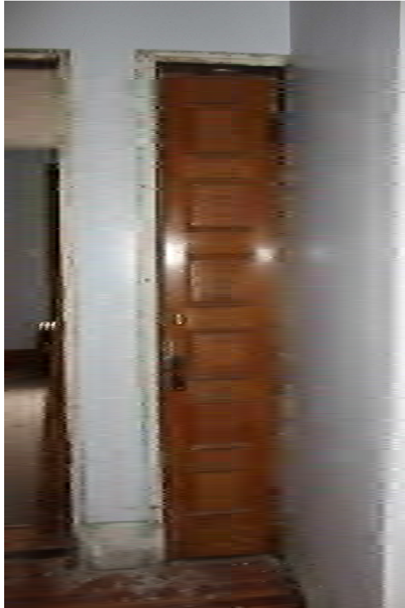
Photo 70. View of a narrow closet door on the third floor of Sheriff's Offices.
