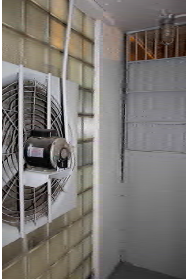
Photo 19. View of the south cell block hallway showing exterior of the shower (right), and the south wall separating from the main structure.
