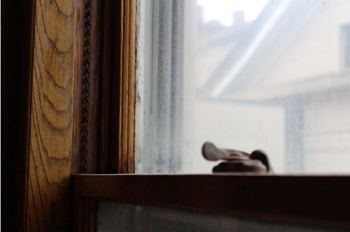
Photo 54. Detail of a frame and sash chain from a second floor window in the Sheriff's Offices.
