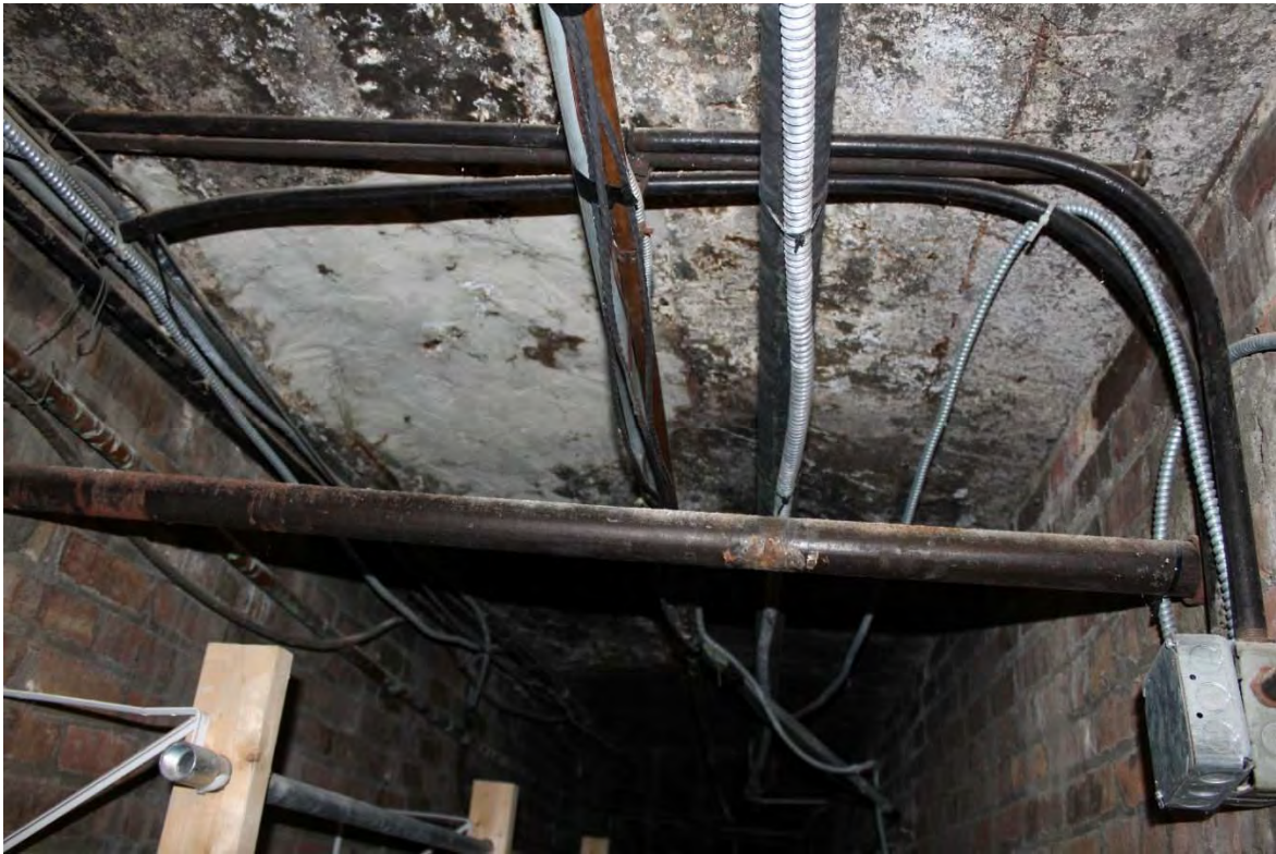
Photo 33. Detail of the ceiling under the A Block portion of the chase floor.
