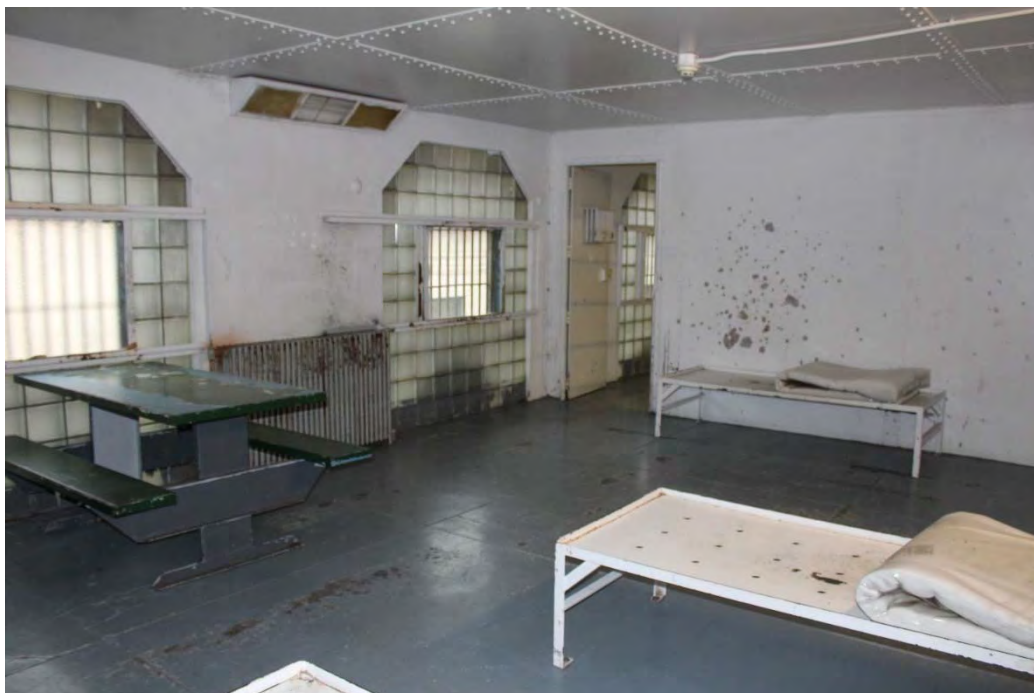
Photo 23. View of C Block dorm housing, facing southeast.
