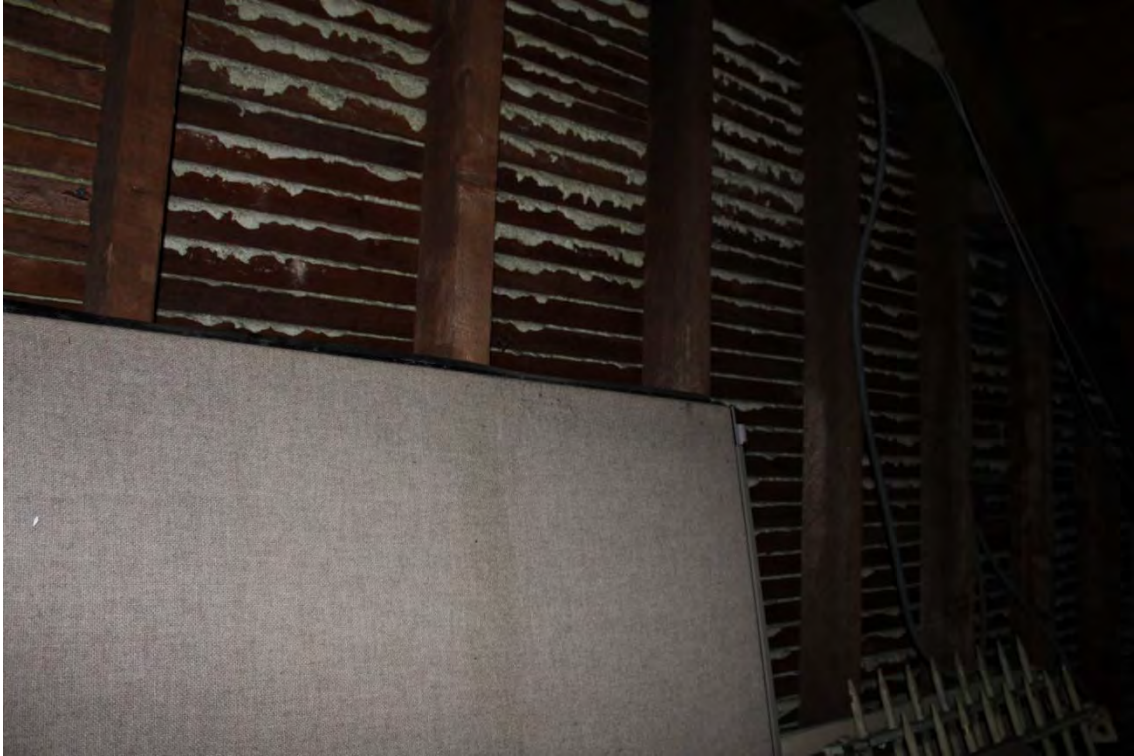
Photo 64. View of lathe and plaster walls in the unfinished attic on the third floor of the Sheriff's Offices.
