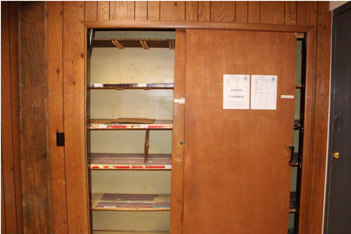
Photo 74. Detail of a closet in the basement of the Sheriff's Offices used for inmate uniform storage.
