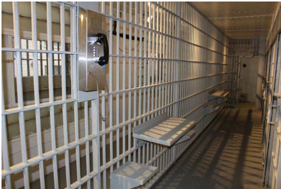
Photo 12. View of the exercise corridor/public area in front of the cell row in A Block, facing north.
