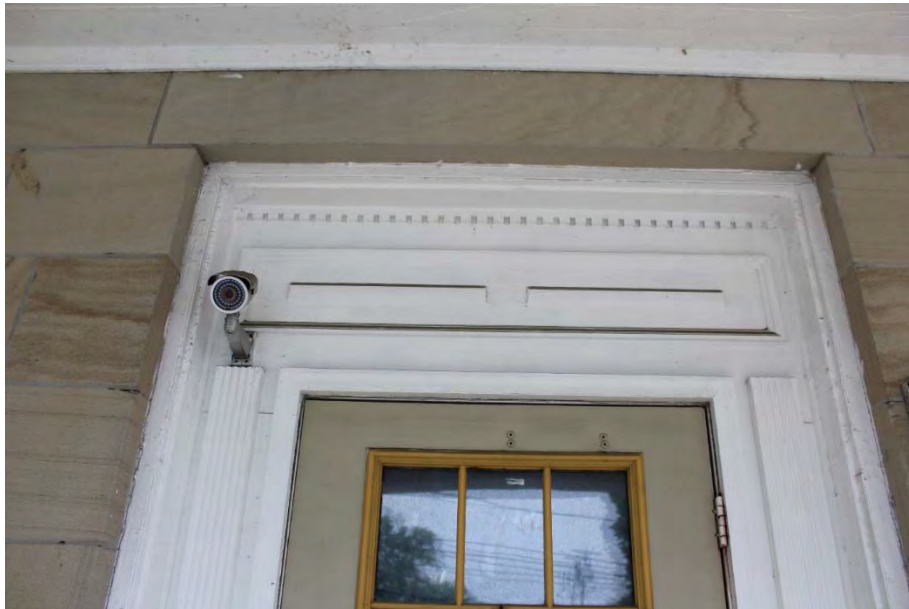
Photo 43. View of the transom above the front door of the Sheriff's Offices.
