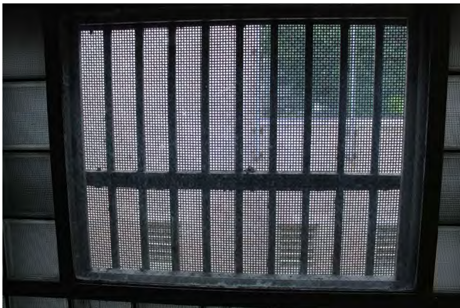
Photo 20. Detail of a typical jail exterior window with exterior steel bars and interior screen in C Block, facing south.
