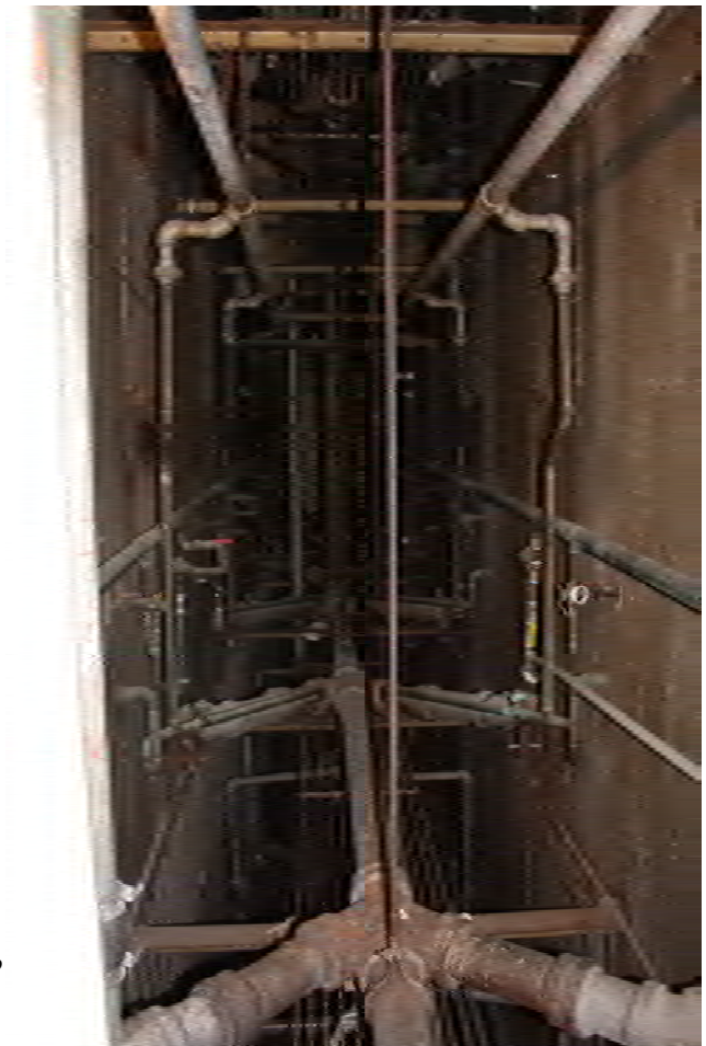
Photo 16. View the chase in B Block, facing south.
