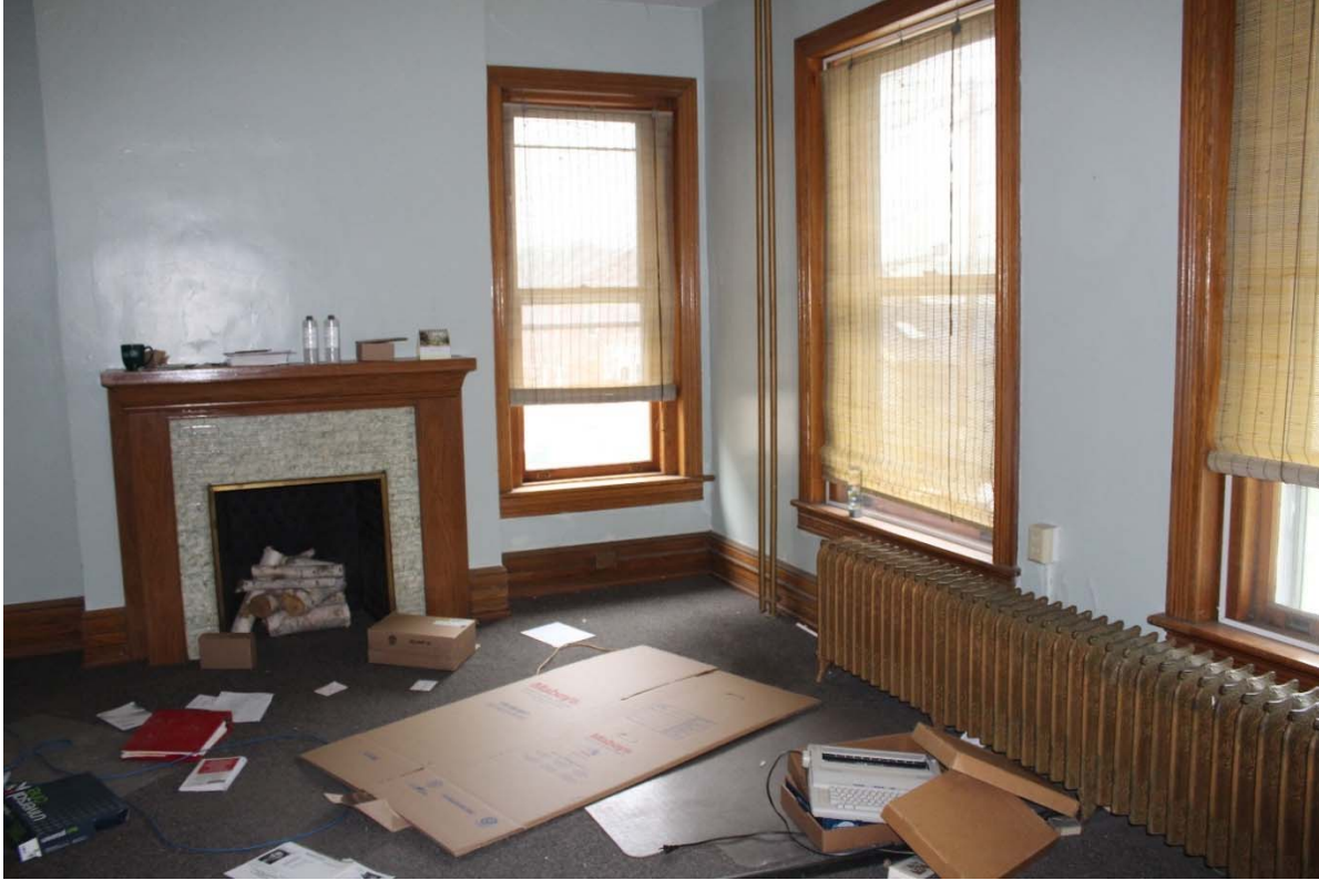
Photo 48. View of an office on northwest corner of the Sheriff's Offices.
