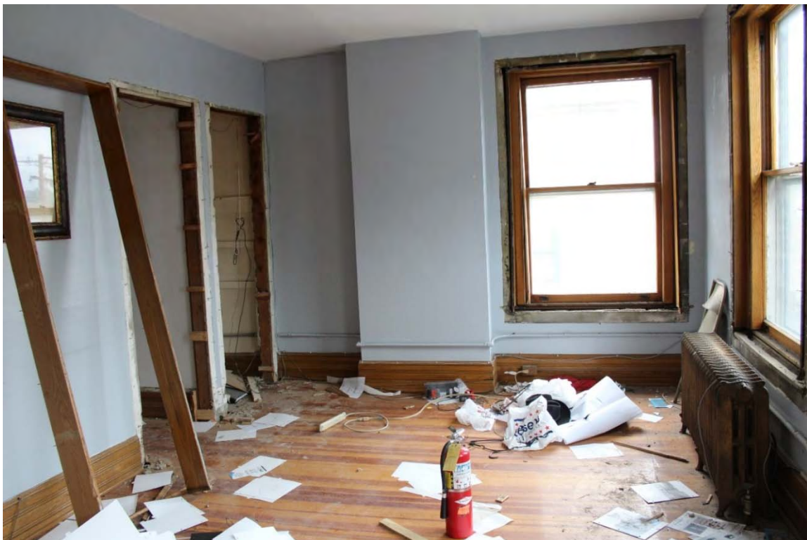
Photo 55. View of the north office on the second floor of the Sheriff's Offices.
