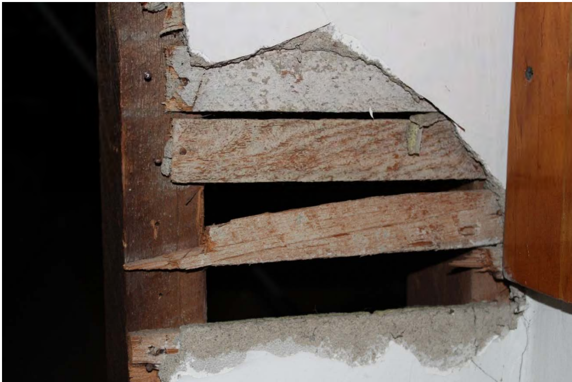
Photo 65. Detail of lathe and plaster walls on the third-floor attic of the Sheriff's Offices.
