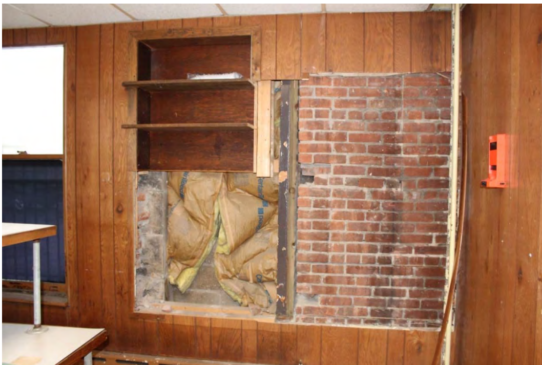
Photo 72. View of an exposed east wall in the basement office of the Sheriff's Offices used for inmate processing.
