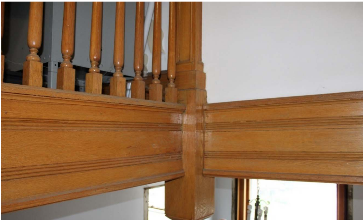
Photo 69. Detail of molding and the stairs railing on the third floor of the Sheriff's Offices.
