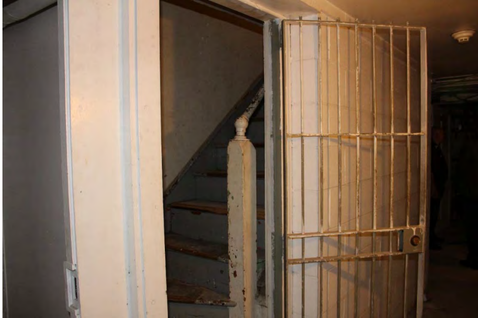
Photo 31. View of the staircase leading from the basement to the first floor.
