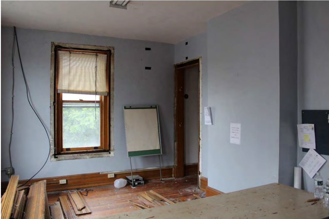
Photo 56. View of the second-floor office in the northeast corner of the Sheriff's Offices.
