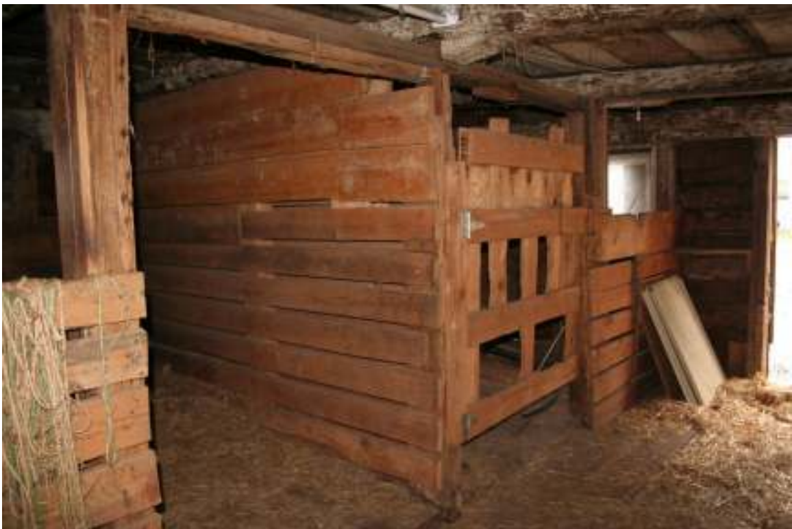
Photo 30. View of interior of easternmost barn showing modern horse stabling pens and white-washed joists above, facing northeast.
