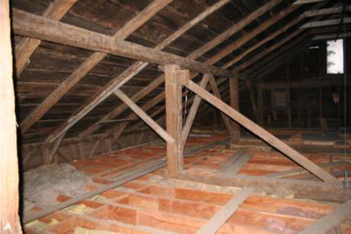
Photo 11. View of the interior of Dutch barn showing rafters, H-bent column, anchor beam, cut-off transverse tie-beam, longitudinal sway bracing and modern bracing, facing southeast.
