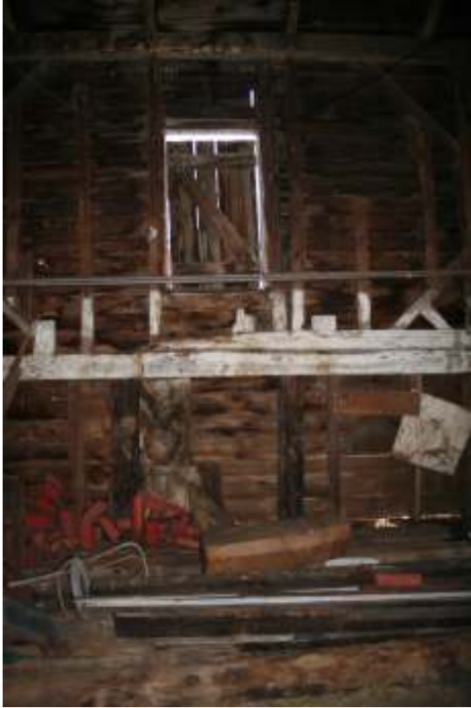
Photo 45. View of interior of cow stable showing location of original hay loft and small hay door, facing west.
