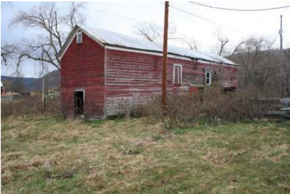
Photo 39. View of westernmost, ground-level cow stable barn, facing northwest.
