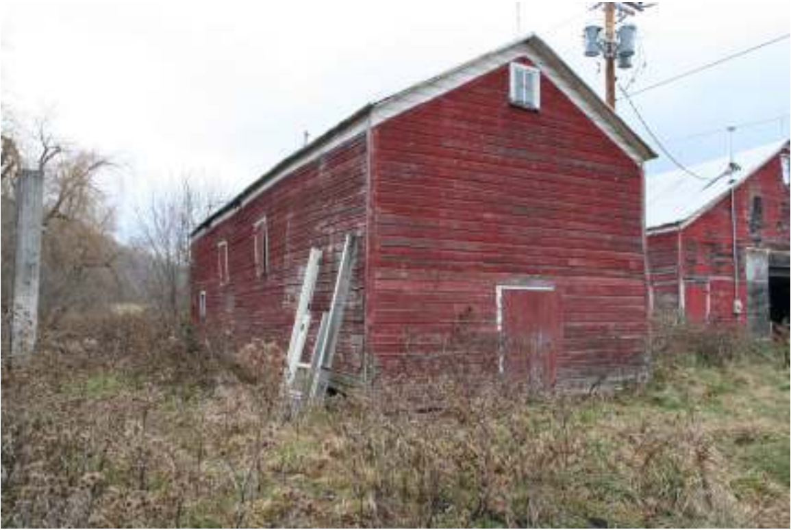
Photo 41. View of cow stable, facing northeast
