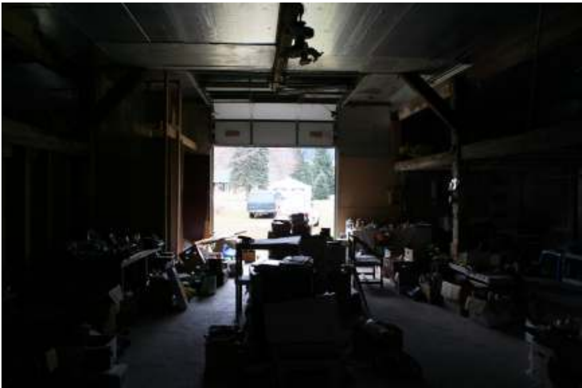
Photo 22. View of Dutch barn ground-level looking down the center aisle, facing south.
