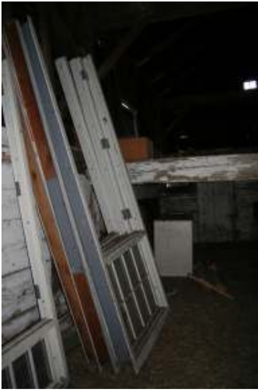
Photo 47. View of interior of cow stable showing white-washed interior with double-boarding, facing northwest.
