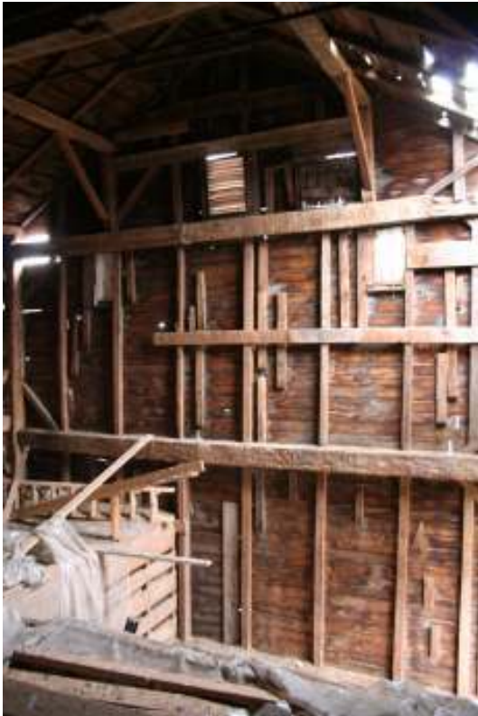
Photo 14. View of the interior west gable wall of the English threshing barn, facing southwest.
