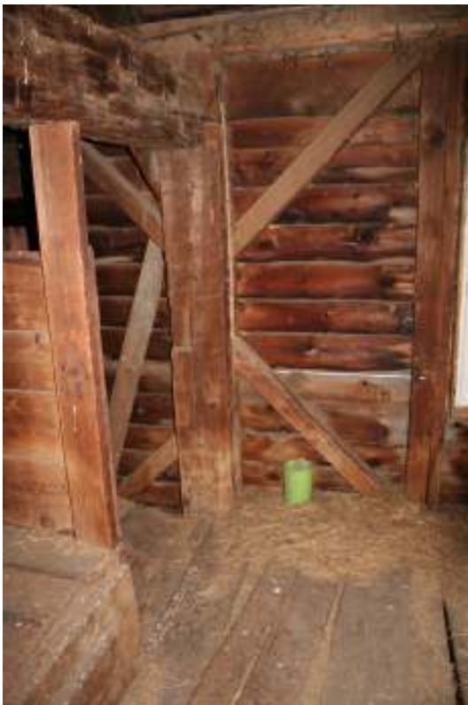
Photo 38. View of loft of easternmost barn showing hewn framing members, facing west.
