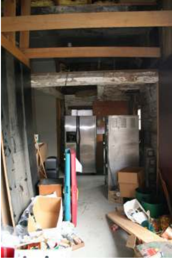
Photo 21. View of Dutch barn ground-level looking at the southeast corner, facing east.
