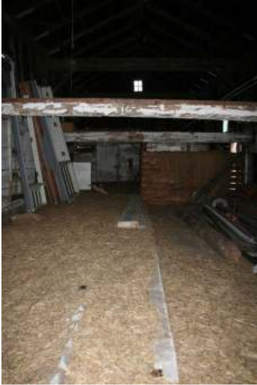
Photo 43. View of interior of cow stable showing concrete floor with manure trough, facing north.
