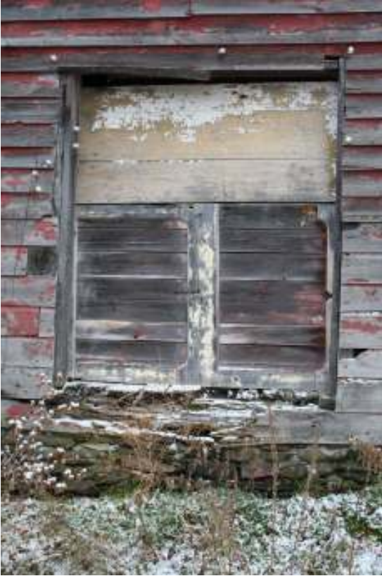
Photo 27. View of side door on easternmost barn also showing the uncoursed fieldstone foundation, facing east.
