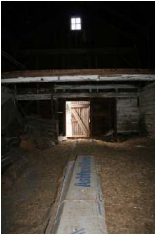
Photo 44. View of interior of cow stable showing concrete floor with manure trough and double-boarded walls with white-wash coating, facing south.
