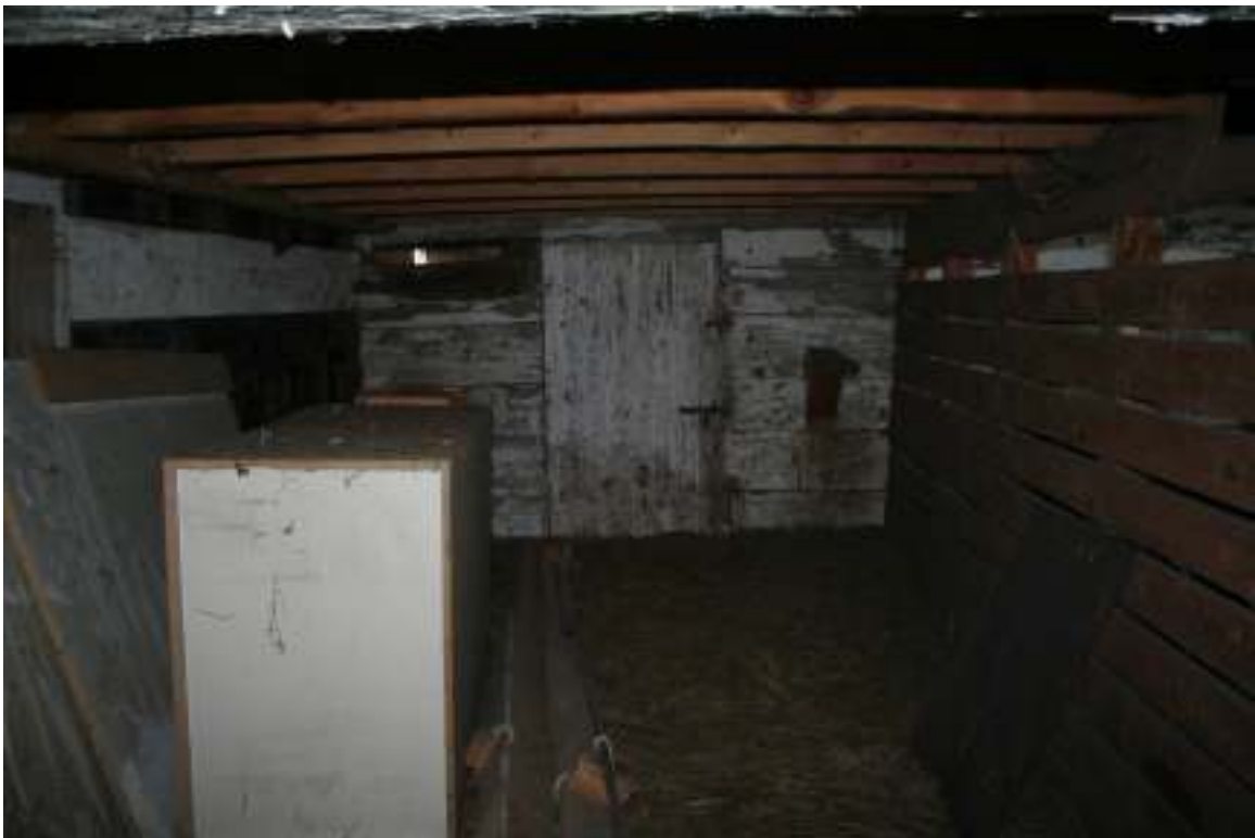
Photo 48. View of interior of cow stable showing location of original hay loft and back pen, facing north.
