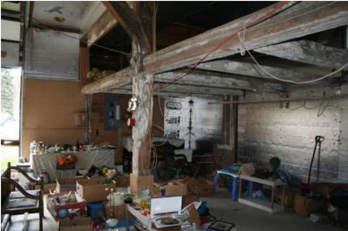
Photo 24. View of Dutch barn ground-level looking at southwest corner showing H-bent column and transverse side-aisle ties all with white-wash coating, facing southwest.
