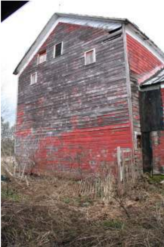
Photo 4. View of English threshing barn addition on Dutch barn, facing east
