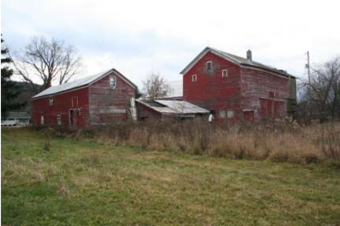
Photo 7. View of Shafer Farm Dutch Barn Complex, facing southwest.
