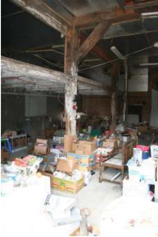
Photo 19. View of Dutch barn ground-level looking down the center aisle, facing northwest.
