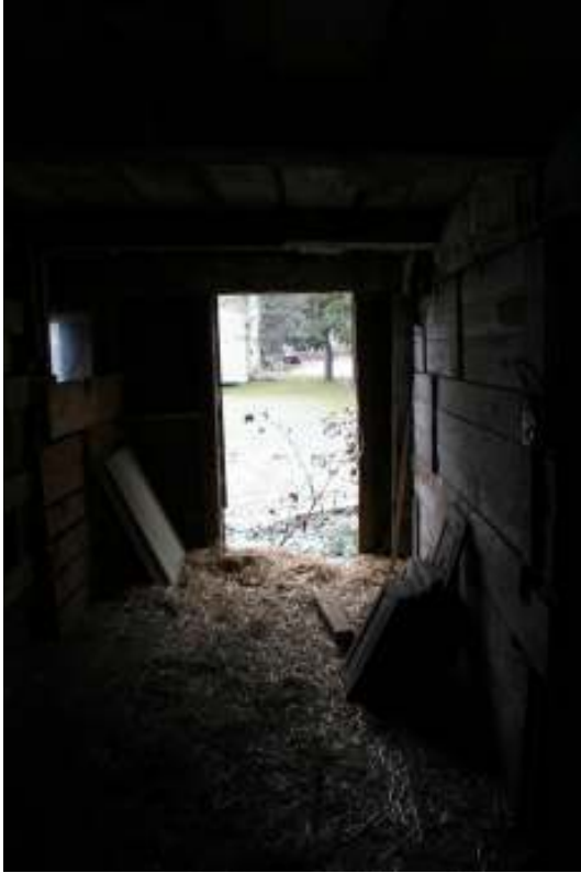
Photo 29. View of interior of easternmost barn showing opening on east wall and white-washed interior walls, facing east.
