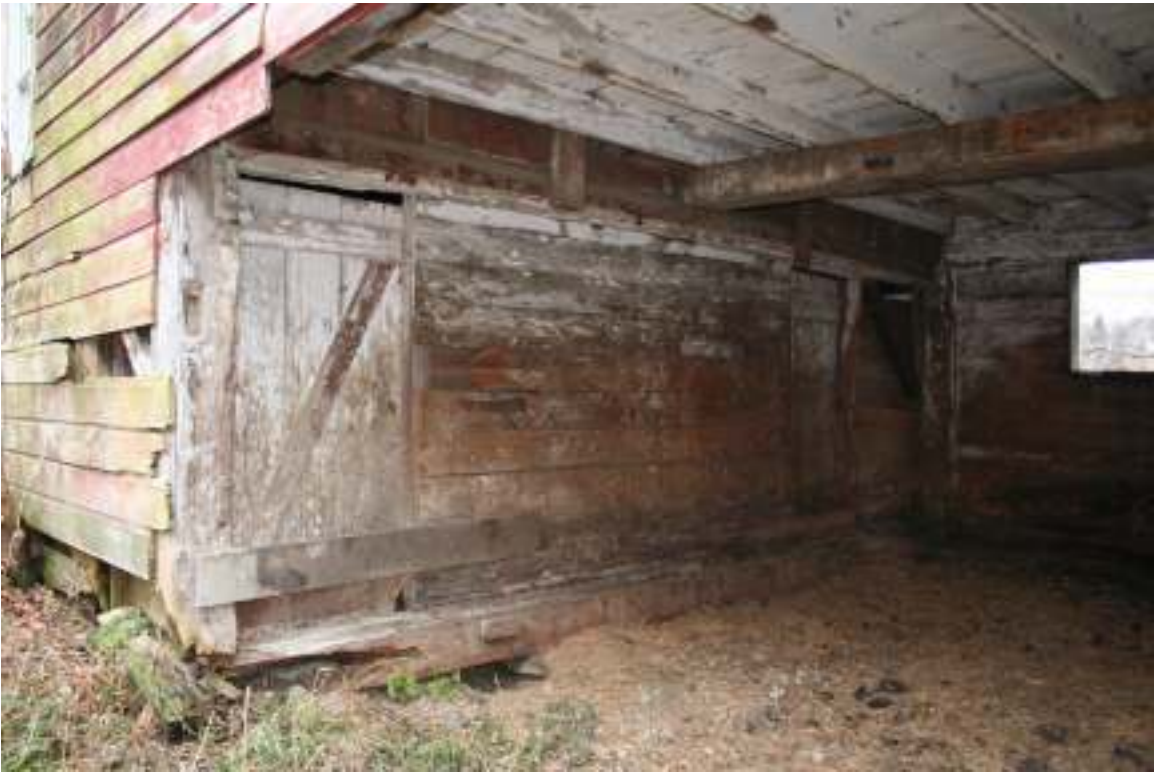
Photo 51. View of vehicle storage in cow stable, facing southwest.
