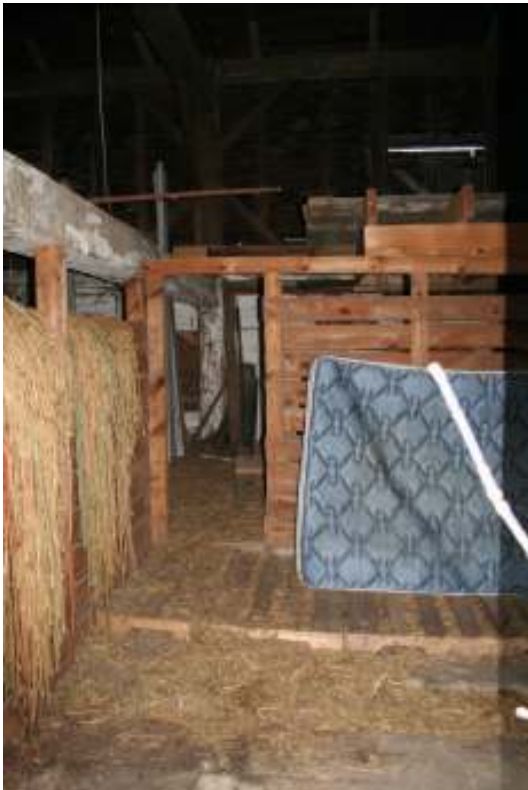
Photo 50. View of interior of cow stable showing small back pen, facing west.
