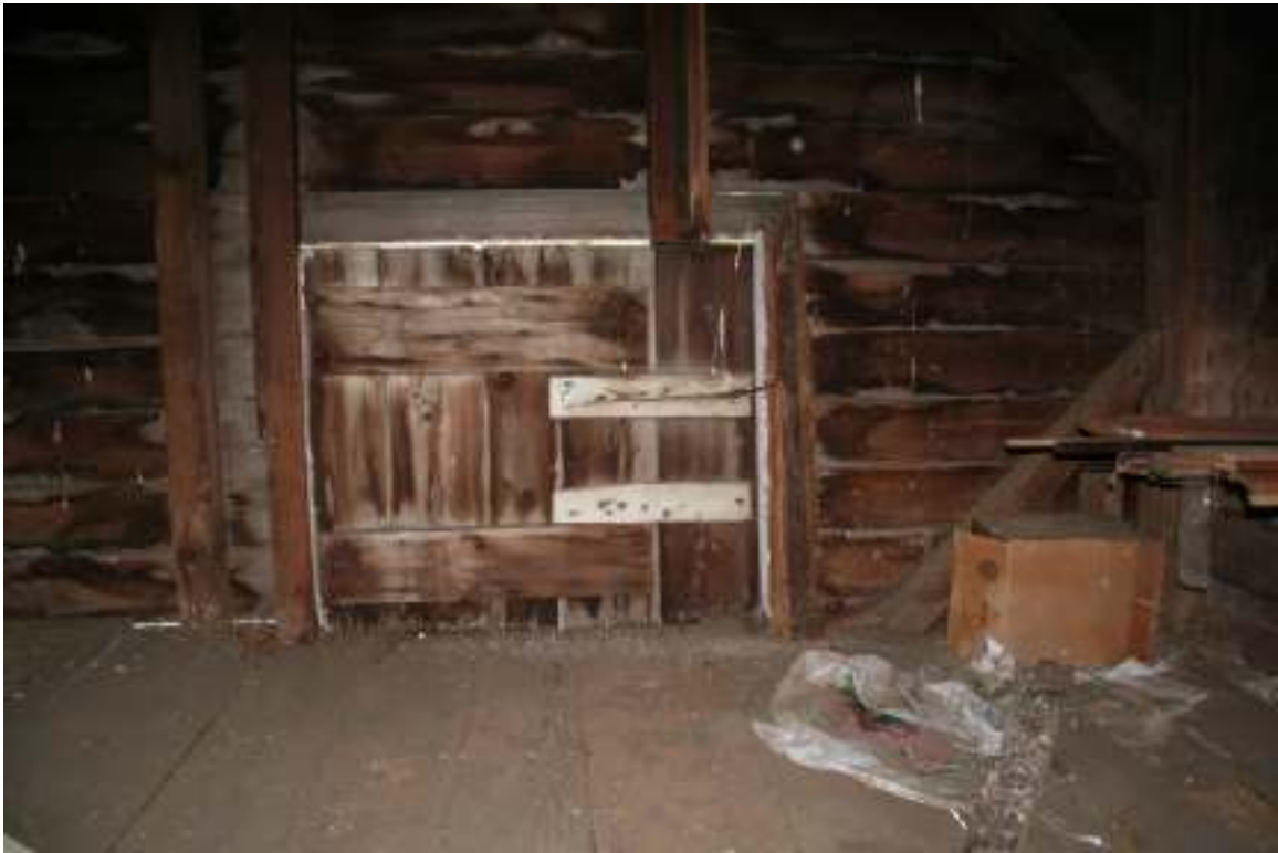
Photo 37. View of loft of easternmost barn showing small door for hay, facing east.
