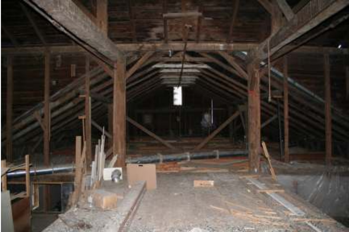
Photo 13. View of the interior of the Dutch B\barn and English threshing barn showing the two barns intersect, facing south.
