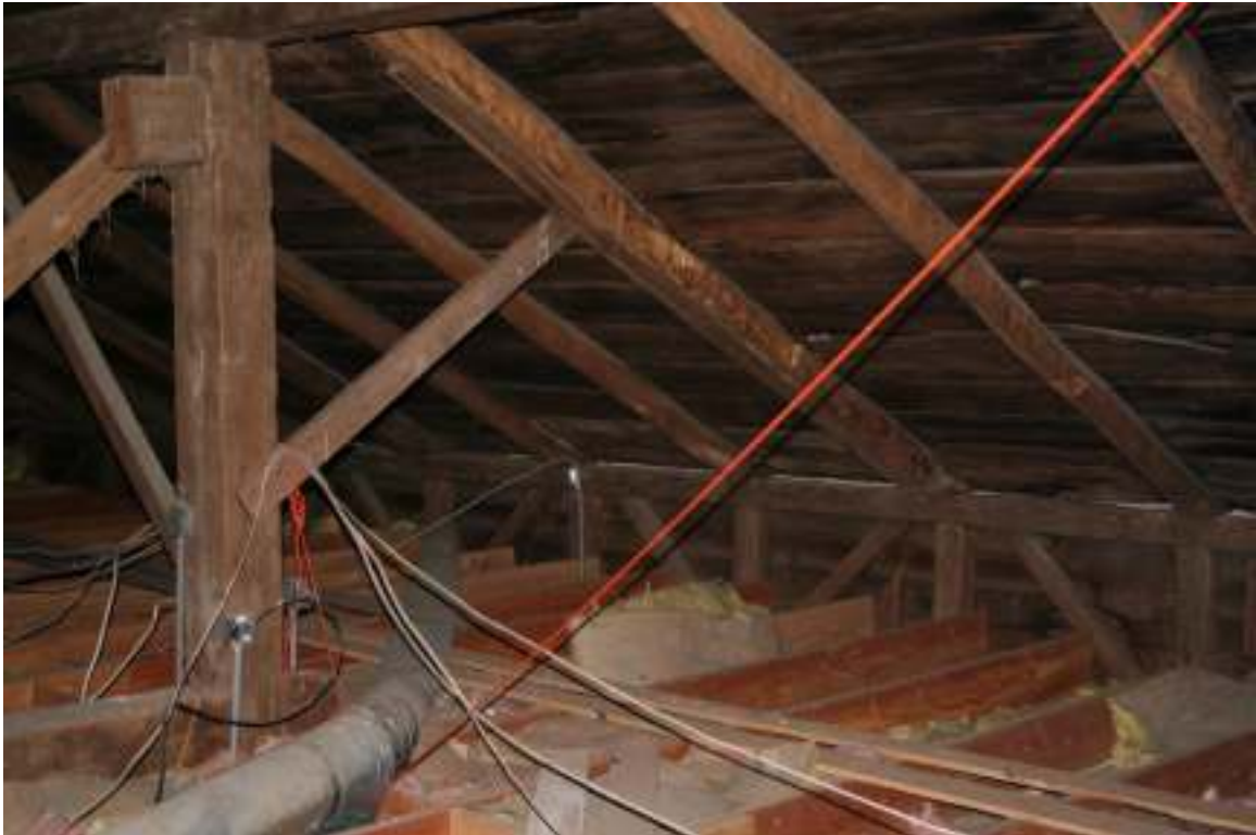
Photo 10. View of the interior of Dutch barn showing rafters, H-bent column, anchor beam, cut-off transverse tie-beam and modern drop ceiling, facing southwest.
