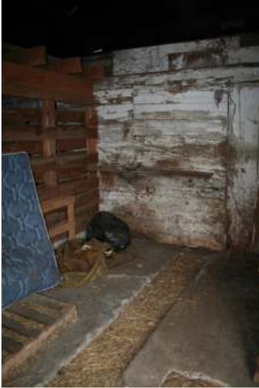
Photo 49. View of interior of cow stable showing small back pen and concrete floor with manure trough, facing northwest.
