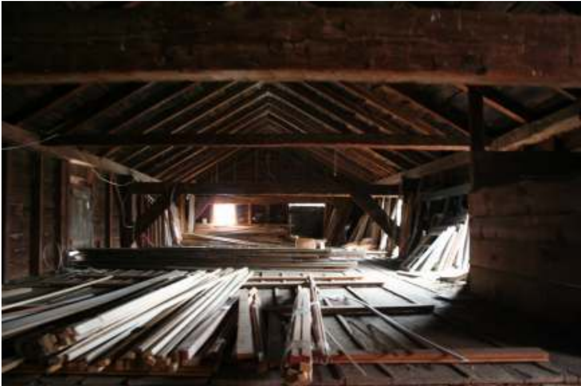
Photo 36. View of loft of easternmost barn showing battened floor boards, facing south.
