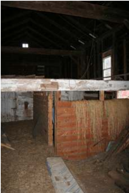
Photo 46. View of interior of cow stable showing modern pen and white-washed timbers, facing northeast.
