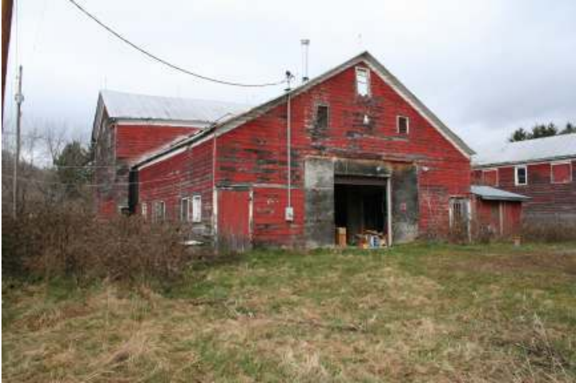
Photo 3. View of Dutch barn from the north side of NYS Route 7, facing northeast.
