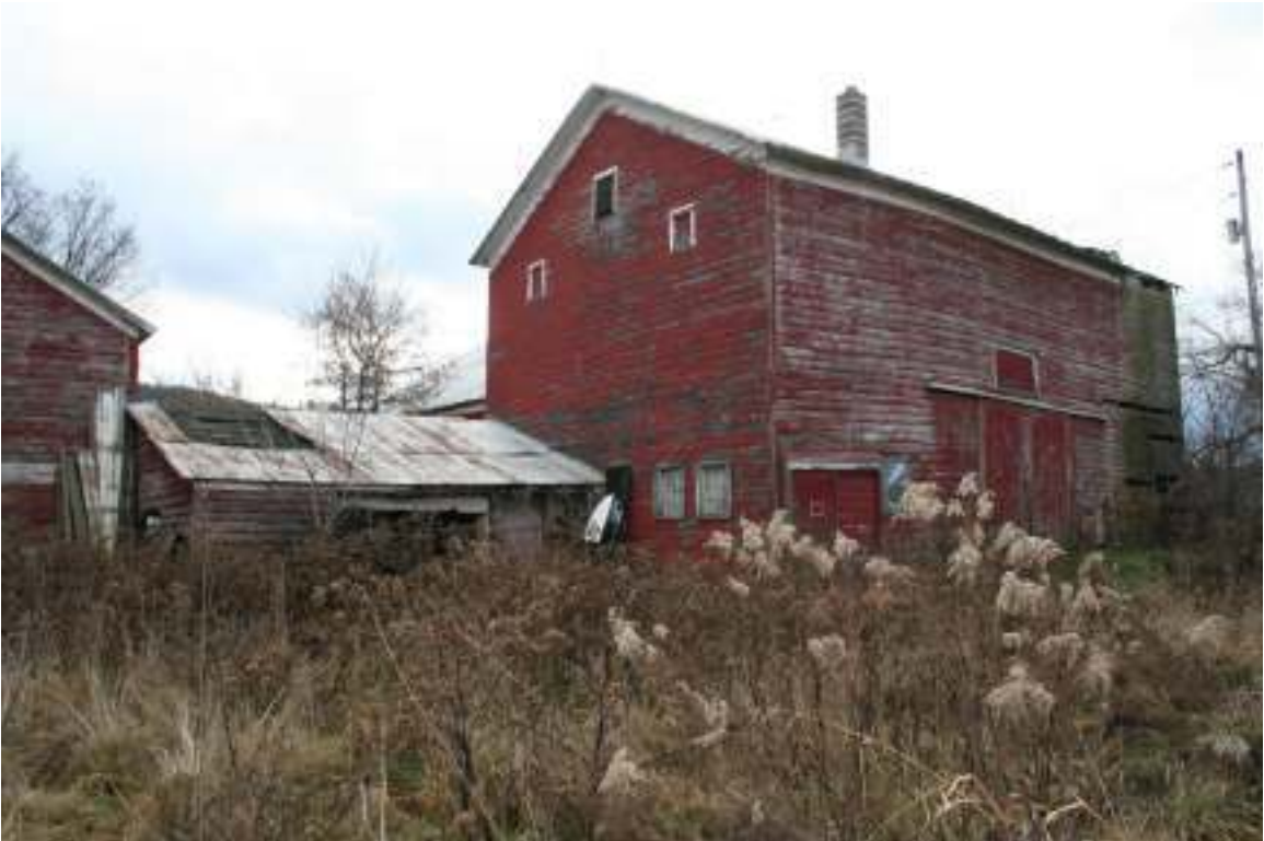
Photo 6. View of English threshing barn addition, facing southwest.
