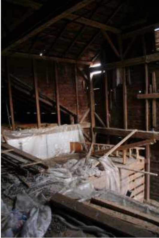
Photo 15. View of the interior southwest corner of the English threshing barn, facing southwest.
