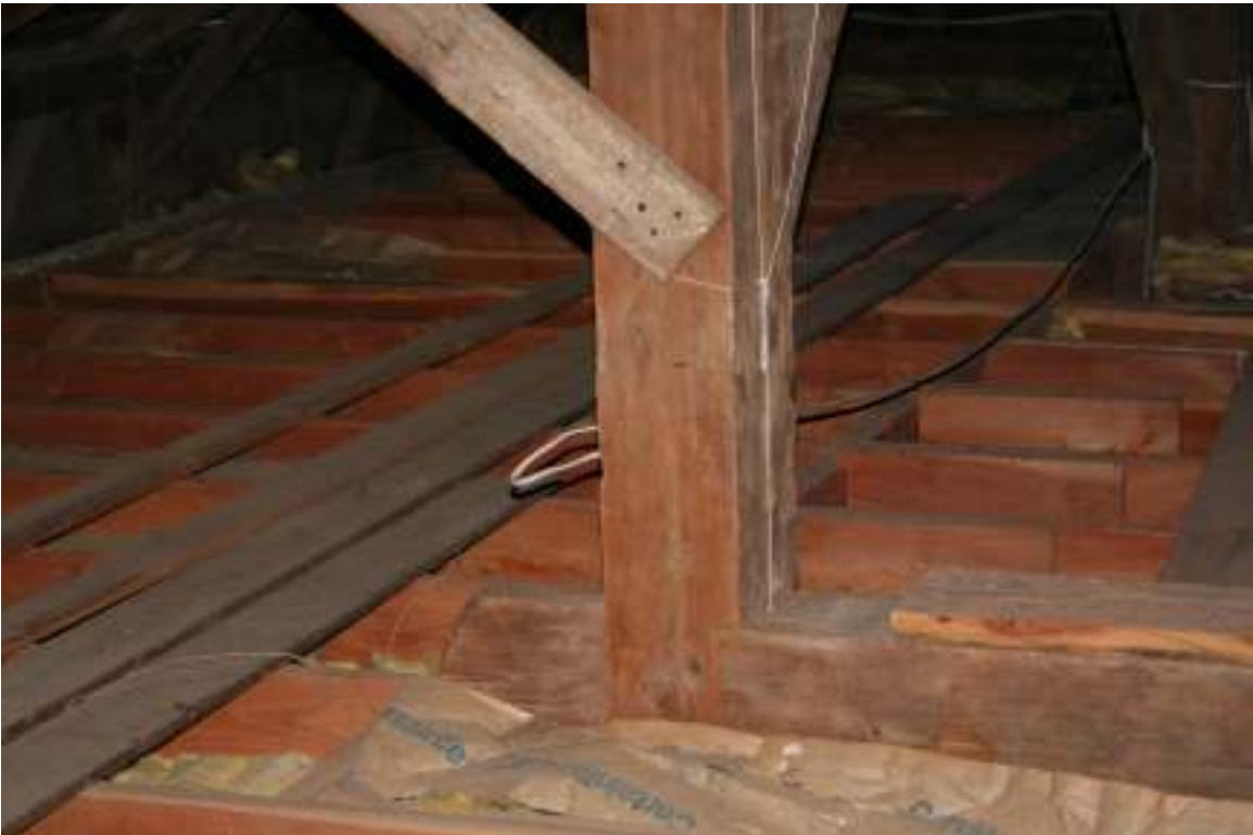
Photo 12. Detail of anchor beam and H-bent column intersection showing marriage marks, facing south.
