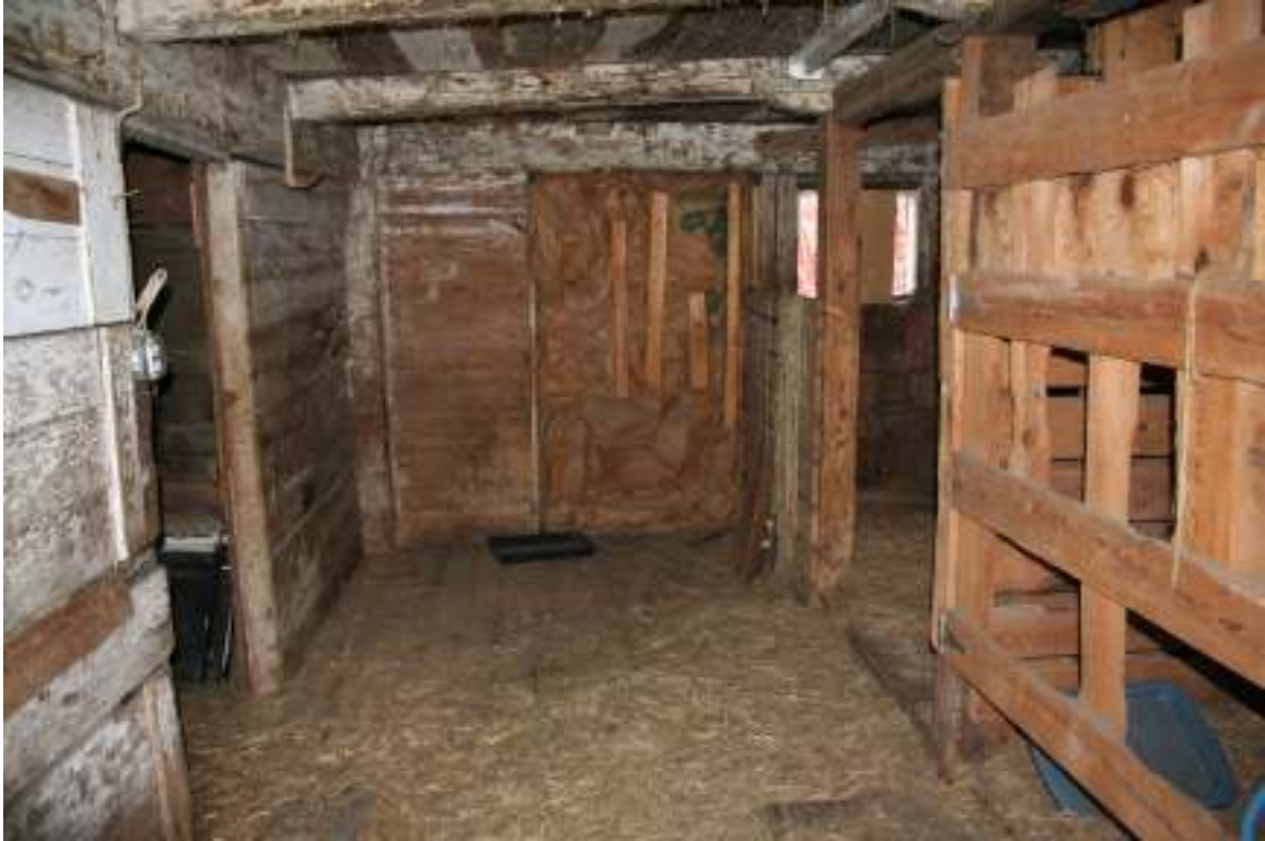
Photo 31. View of interior of easternmost barn showing modern horse stabling pens and white-washed joists and walls, facing west.
