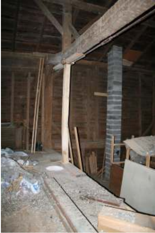
Photo 17. View of the interior north wall of the English threshing barn showing a modern concrete block chimney stack, facing southwest.
