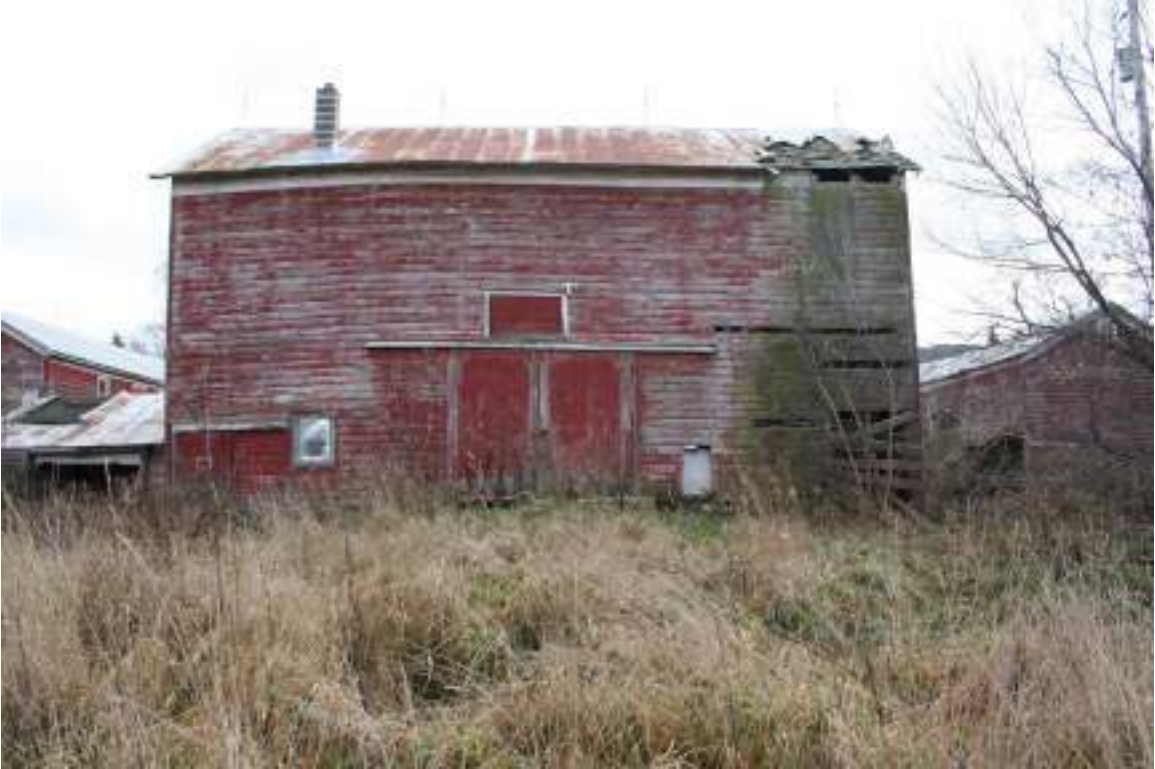
Photo 5. View of English threshing barn addition, facing south.
