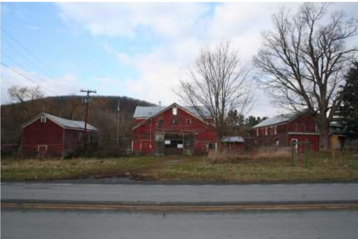
Photo 52. View of Shafer Farm Dutch Barn Complex from the south side of NYS Route 7, facing north.
