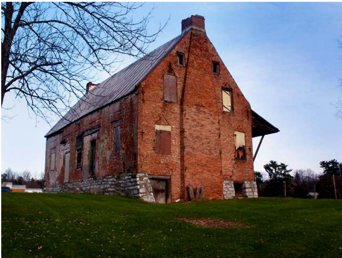
Photo 37. The Van Hoesen House, ca. 1730, near Hudson City, New York. The earliest known brick house surviving in the Hudson Valley. A metal roof added in the 19th century covers the distinctive parapet gables. A brick veneer covers the timber-frame substructure.
