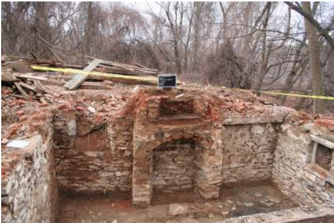
Photo 10. View of north end of McCutcheon House basement showing relieving arch and a portion of the first floor fireplace, facing north.
