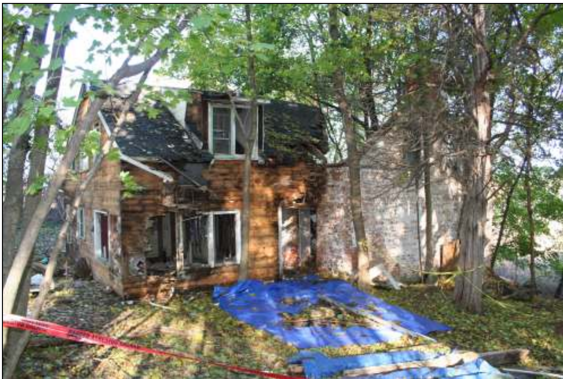
Photo 2. The Peter McCutcheon House, facing north.
