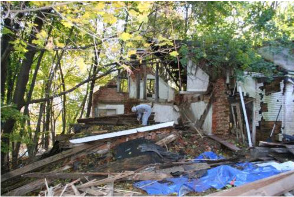
Photo 14. View of structural dismantling and asbestos abatement process, facing southeast.
